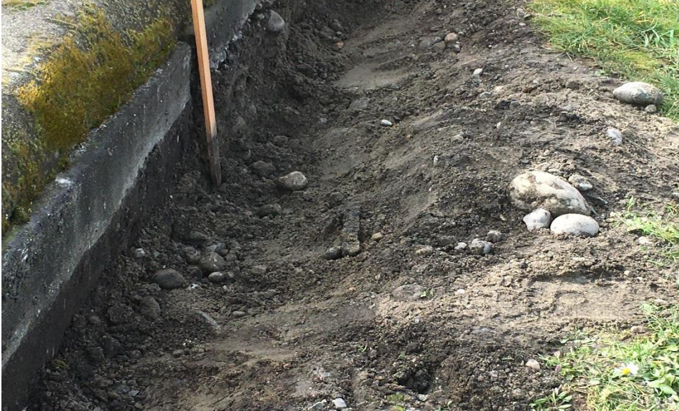
Explanation: Closer view of the area of additional soil removal and location of second-round soil sample TS-soil-030221 .
