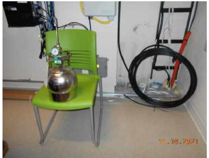
Photograph 4. View of indoor air testing within the Site building.
