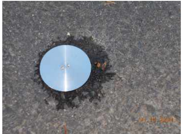
Photograph 6. View of sub-pavement soil vapor monitoring point TVMP-10, located east of the Site building with flush-grade cap in place.
