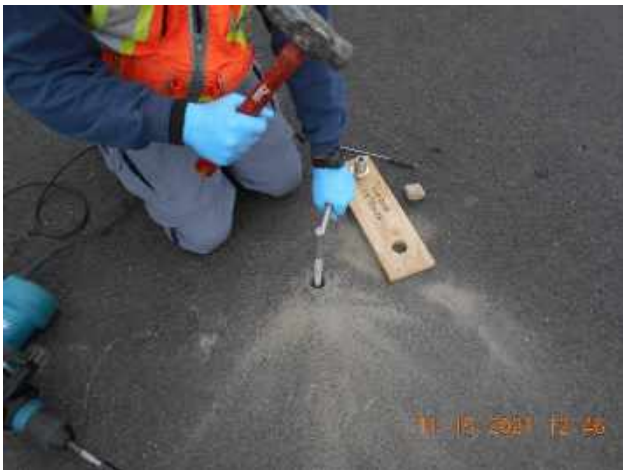
Photograph 5. Installation of sub-pavement soil vapor monitoring point TVMP-10, located east of the Site building.
