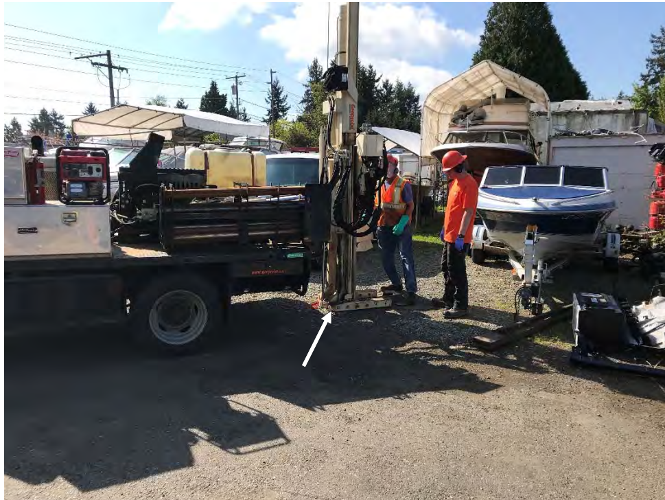
Photograph 12 – FL-211 – Boring location FL211-B5 (white arrow) looking southeast. Boat storage in photo background.
