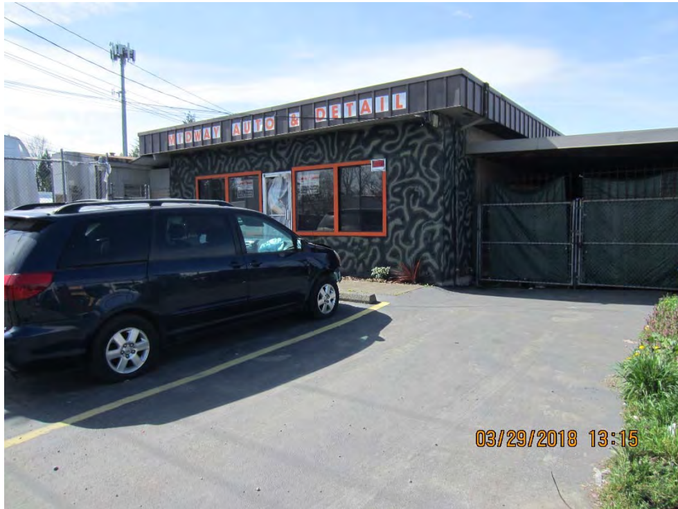
Photograph 1 - FL-210 - Midway Auto & Detail Building, view looking west from 30 th Street S.
