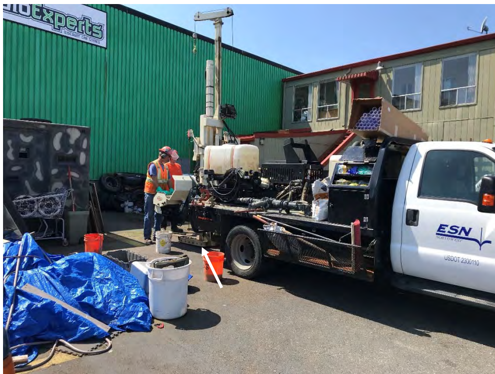
Photograph 11 – FL-212 – Boring location FL212-B2 (white arrow) looking southwest.
