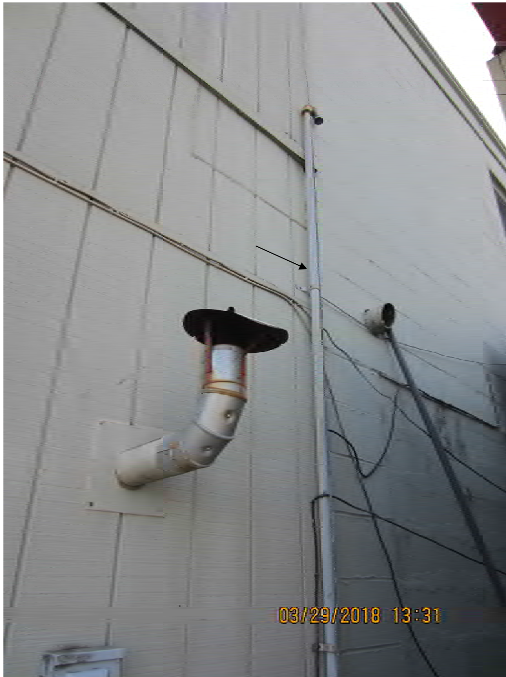
Photograph 9 – FL-212 – Black arrow points to possible UST vent pipe observed on the north side of the apartment building, near the northeast corner of the building.
