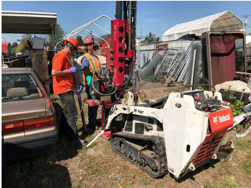
Photograph 15 – FL-213 – Boring location FL213-B10 (white arrow), view looking north.
