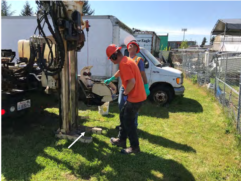
Photograph 14 – FL-213 – Boring location FL213-B8 (white arrow), view looking west.
