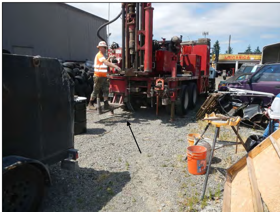
Photograph 16 – Boring location FL209-B9 (arrow), view to west.
