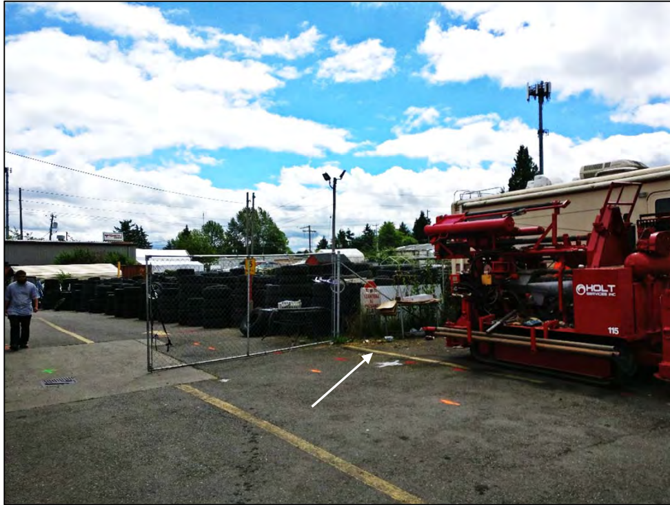
Photograph 9 - Drilling soil boring FL209-B2 (see arrow), view to southeast.
