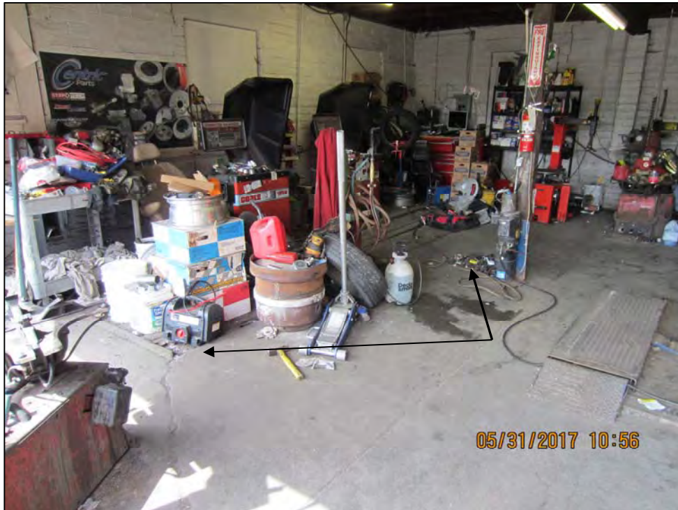
Photograph 3 - FL209, auto repair garage interior, showing wooden-plank-covered pit (arrows), covered by stored items.
