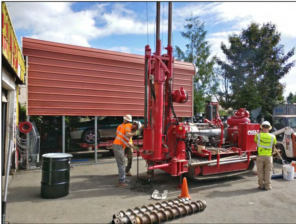
Photograph 11 – Drilling boring FL209-B4, view to north
