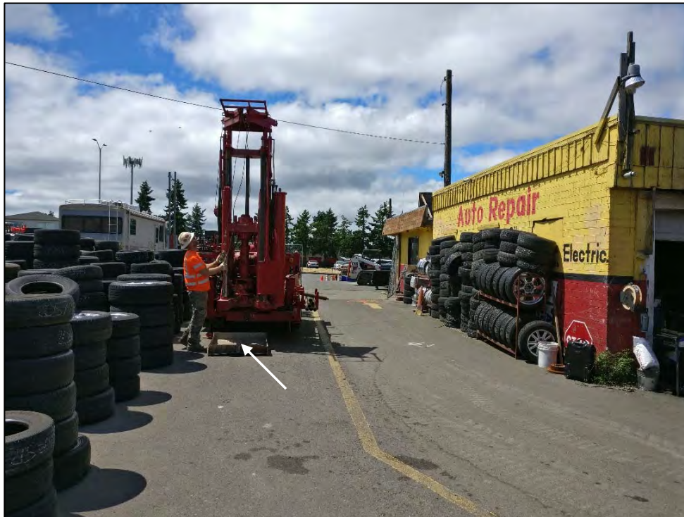
Photograph 10 - Drilling soil boring FL209-B3, view to west.
