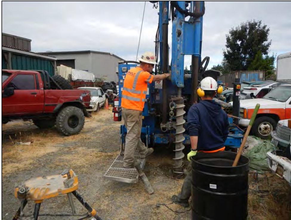
Photograph 23 – Boring location FL209-B12, view to west.
