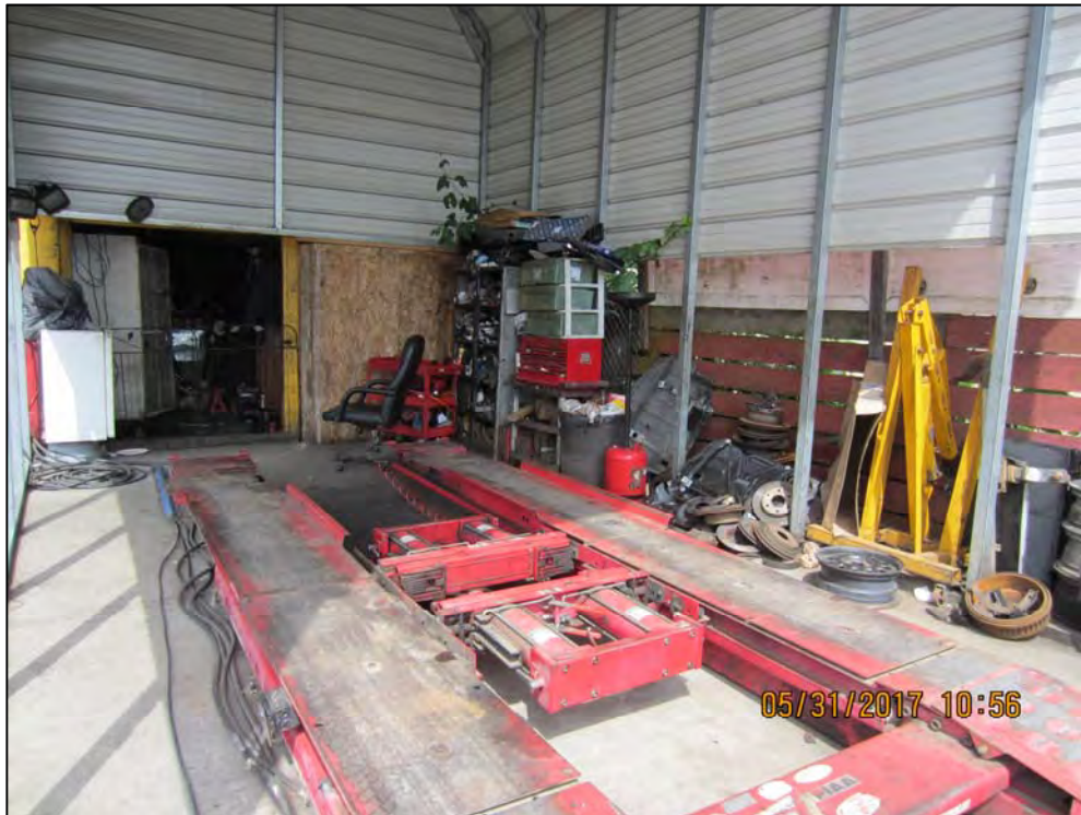
Photograph 4 - FL209, aboveground hoist located east of auto repair building in temporary shed.
