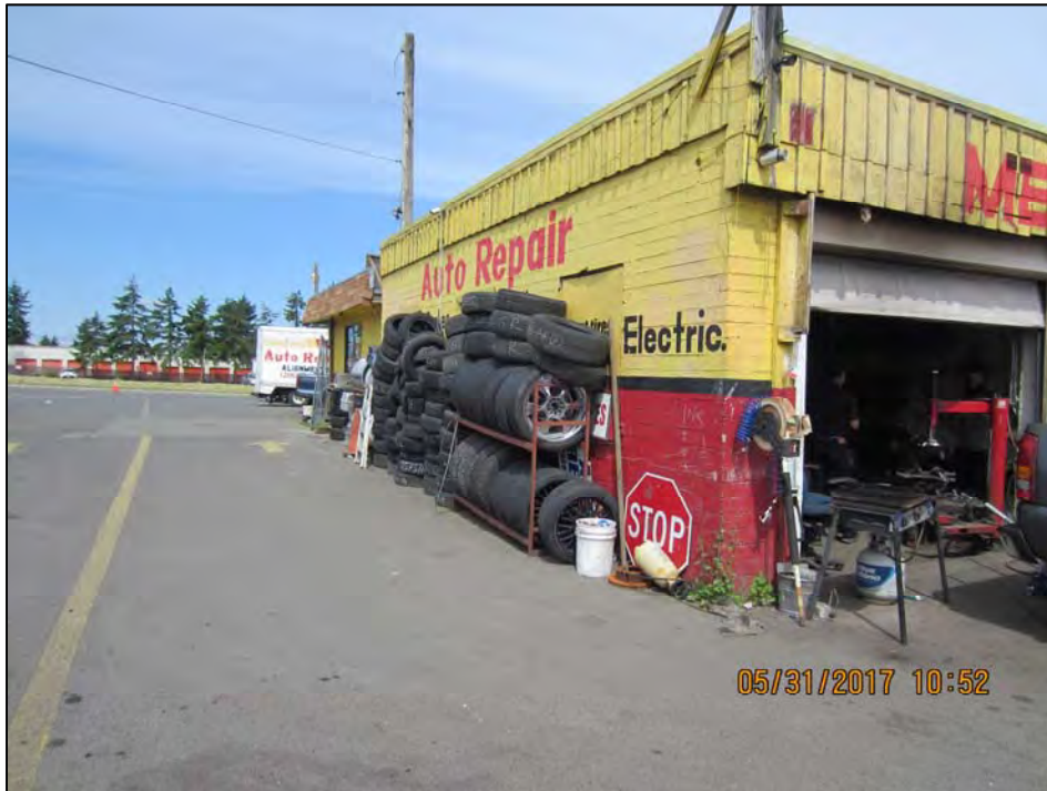
Photograph 1 - FL209, auto repair building and entrance off Pacific Highway S. Photo shows concrete pad in center of paved drive; presumed oil/water separator or storm drain. View to west.
