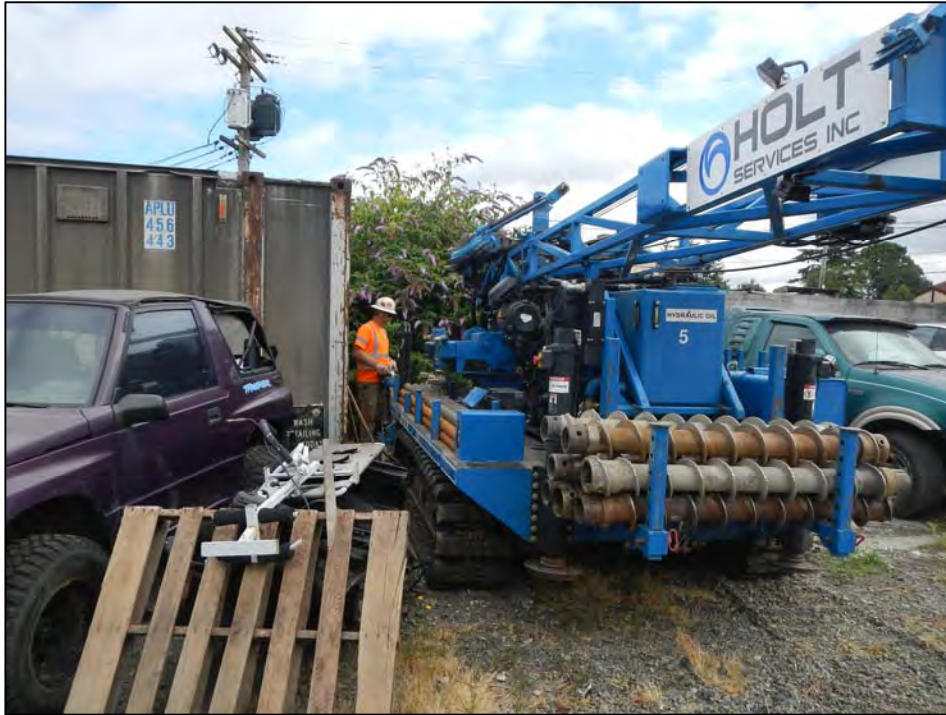
Photograph 17 – Boring location FL209-B10, adjacent to north fence where residual petroleum-contaminated soil reportedly remains. View to north.
