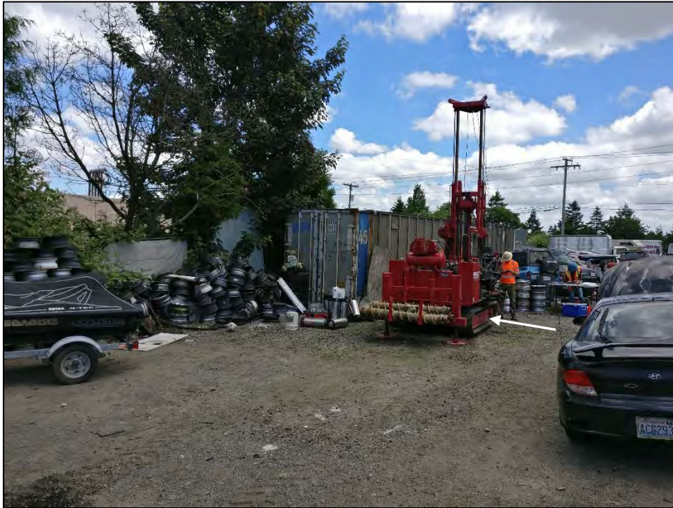
Photograph 13 – Boring location FL209-B6, view to northeast.
