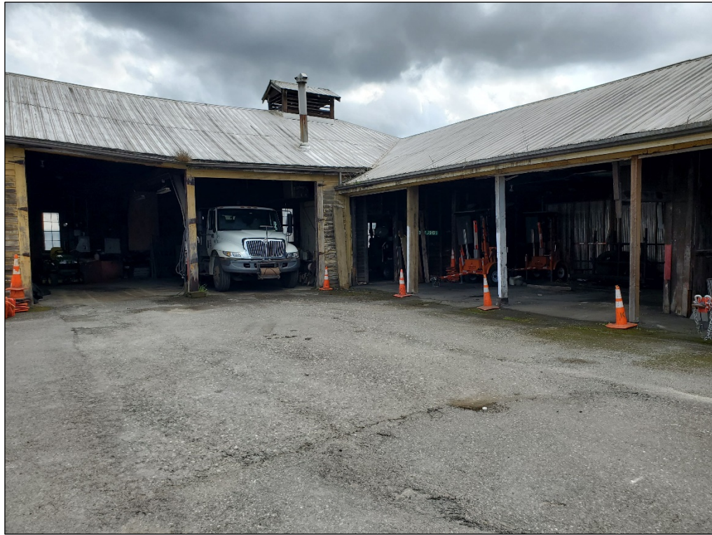
3. Capped area of Building 3.
