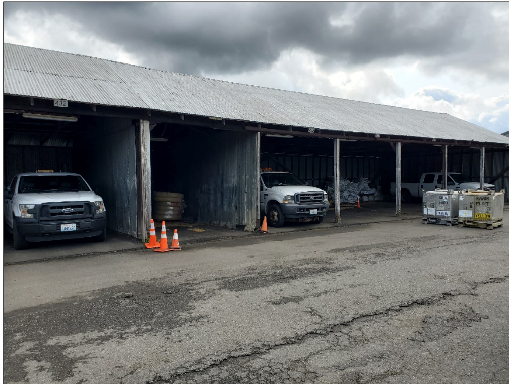
1. Capped area of east truck storage shop.
