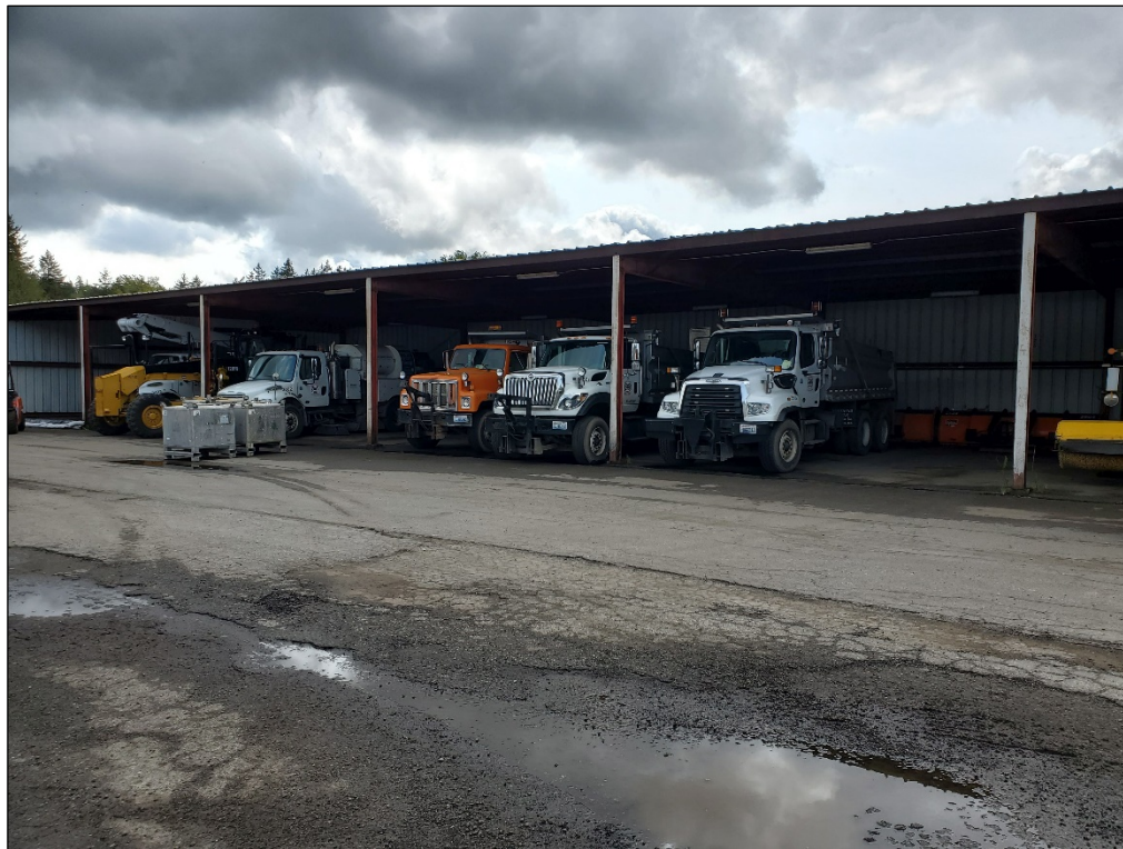
2. Capped area of south truck storage shed.
