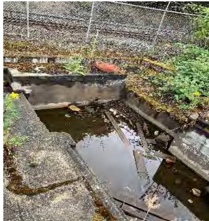
Photograph A-2-16. Concrete vault with standing water. (July 2019)
