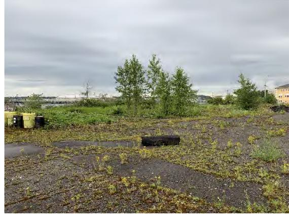
Photograph A-2-14. Containment Area: concrete slabs with weeds growing along joints. (July 2019)
