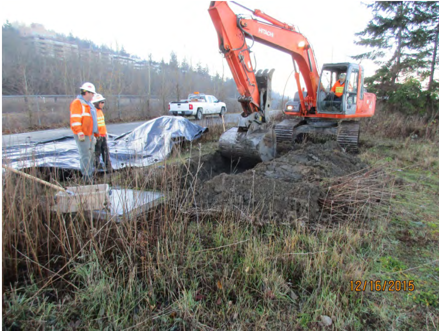
Photo 1: Excavator and start of test pitting (at location TP-TTWP-C)
