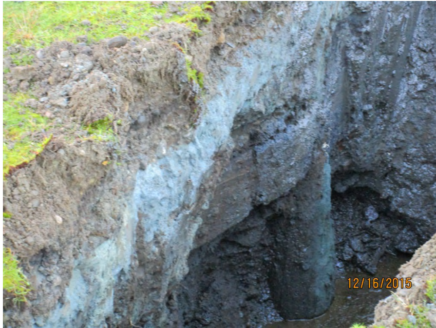
Photo 11: TP-TTWP-N –Wood pile and pile cap (wood wall behind pile cap not shown)
