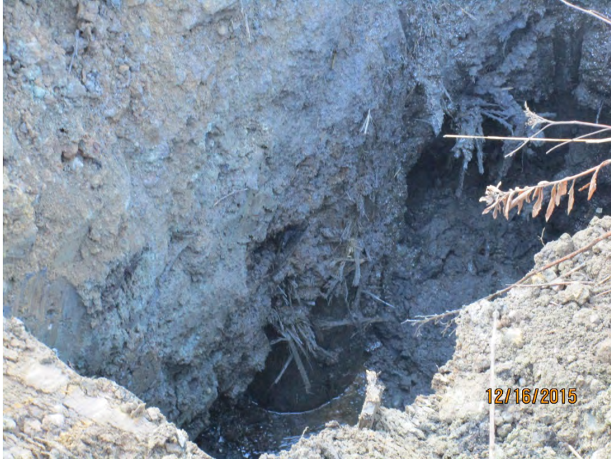
Photo 7: TP-TTWP-C – Wood pile
