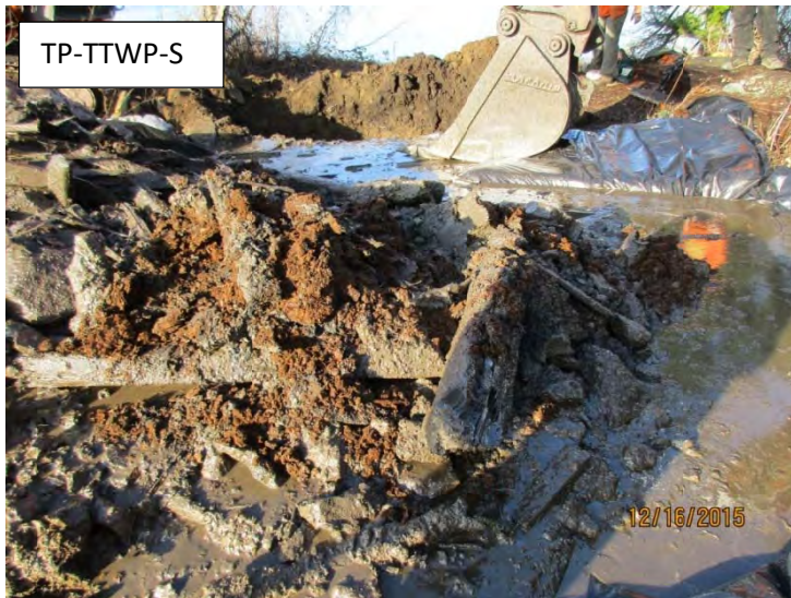
Woody debris in TP-TTWP-S (left) high volume of wooden piles and timbers. TP-TTWP-N (right) significant large dimensional lumber debris present.
