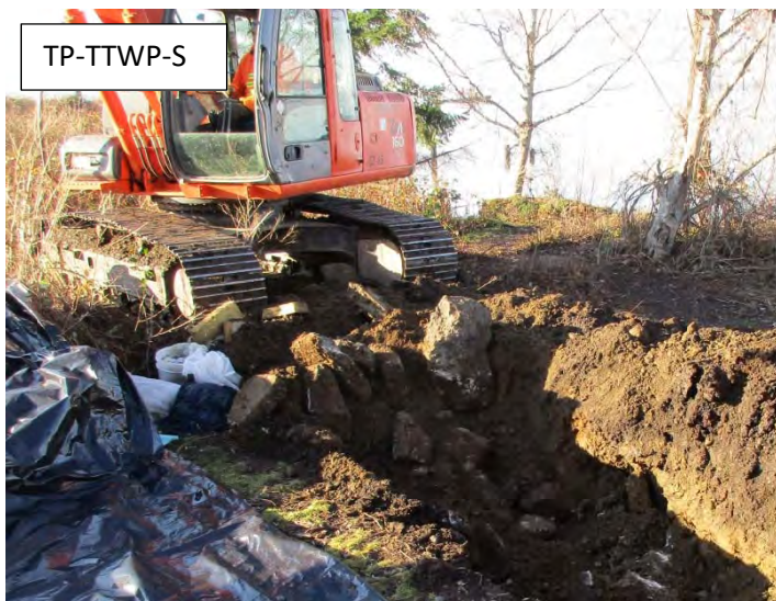
Concrete debris in the surface of TP-TTWP-S (left) and woody debris in TP-TTWP-WF (right).
