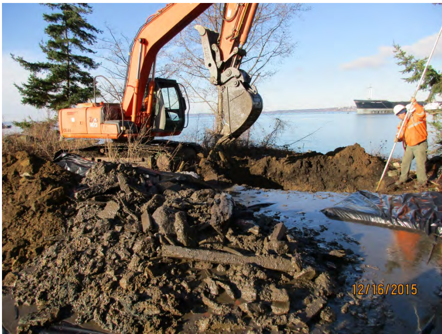
Photo 4: TP-TTWP-S – High volume of wood debris
