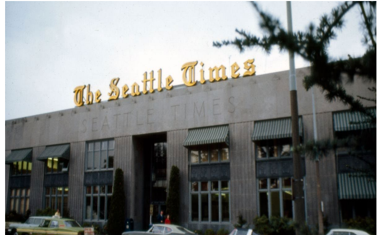
Historic Seattle Times building facade.
