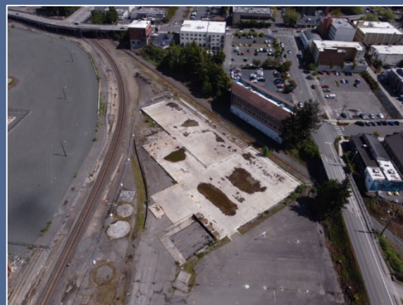
Aerial view of Lignin Operable Unit and downtown Bellingham, May 2021
