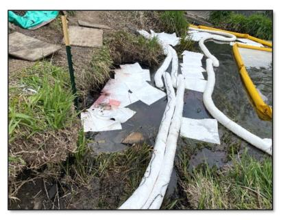
embankment adjacent to the South Fork Palouse River. An April 2022 fuel release from a 10,000-gallon Above Ground Storage Tank (AST) resulted in impact to underlying site soils and near shore river water.
