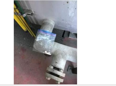
White fibrous insulation with various colors of pipe wrap covers (e.g., also includes red pipe in southwest corner of room that runs to north section of room). Difficult to quantify due to distribution and various wrap colors.
