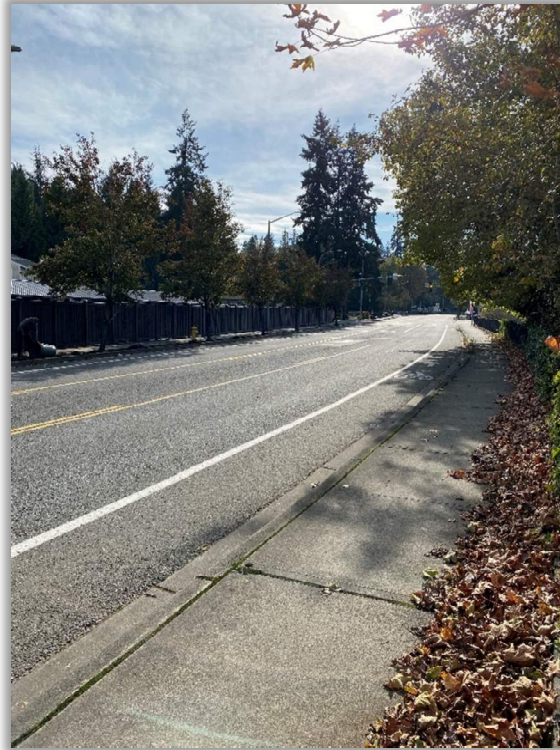
View looking north from the proposed driveway on Slater Ave NE
