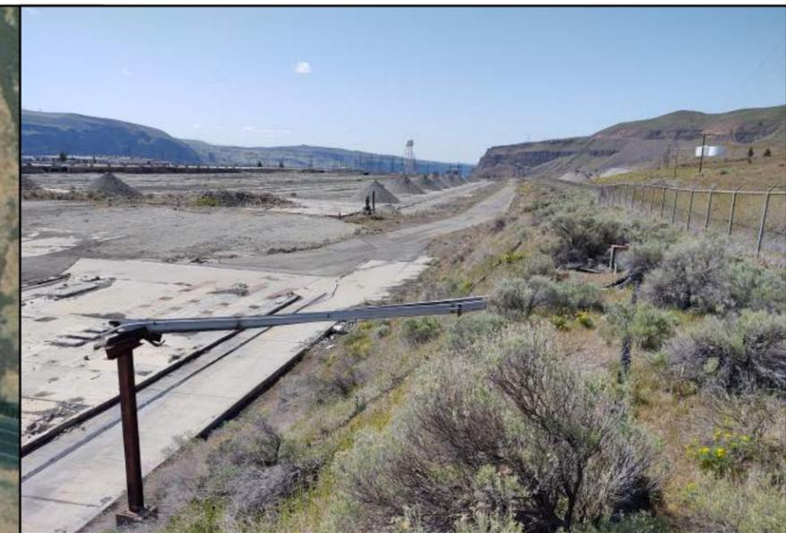
View to west of 190-PSP-2" SO<sub>2</sub> purge line emerging above ground to join northern wall of former Tertiary Treatment Plant (SWMU 8).
