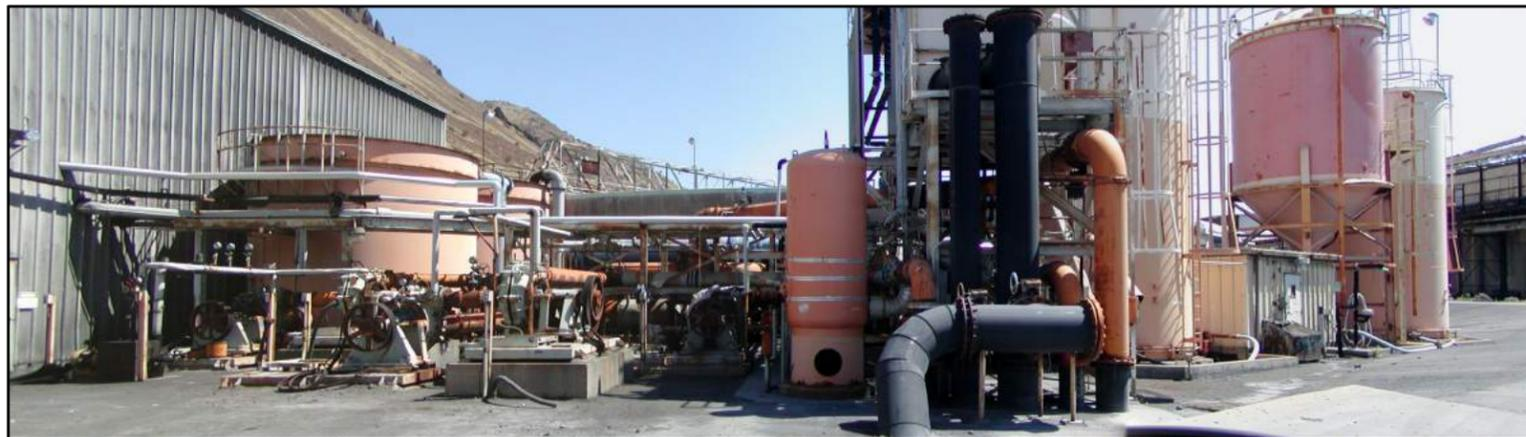
Panorama to the east showing pipe network, recycle tanks (left), caustic tanks (center), CaCl<sub>2</sub> tanks (right), tertiary treatment building (far left) and large clarifier (background center).
