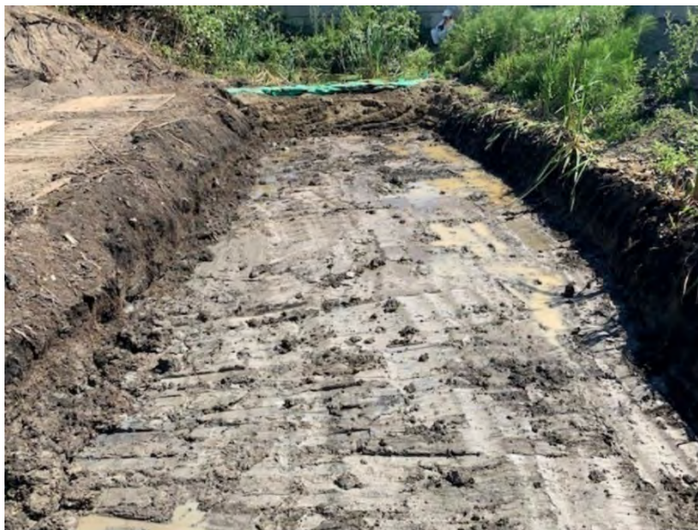
Figure 48: Bottom and western sidewall of RAU D11
