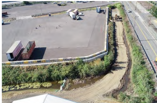
Figure 8: Temporary Access Road Inside the Ditch
