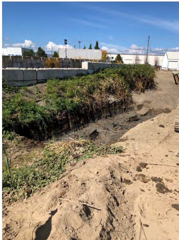
Figure 46: Bottom and western sidewall of RAU D9
