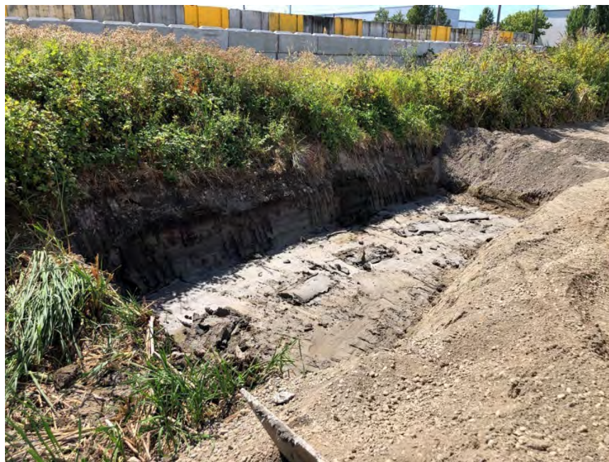
Figure 41: Bottom and western sidewall of RAU D4
