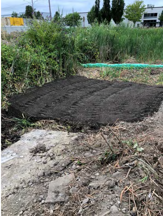
Figure 15: Typical Steam bed backfilling
