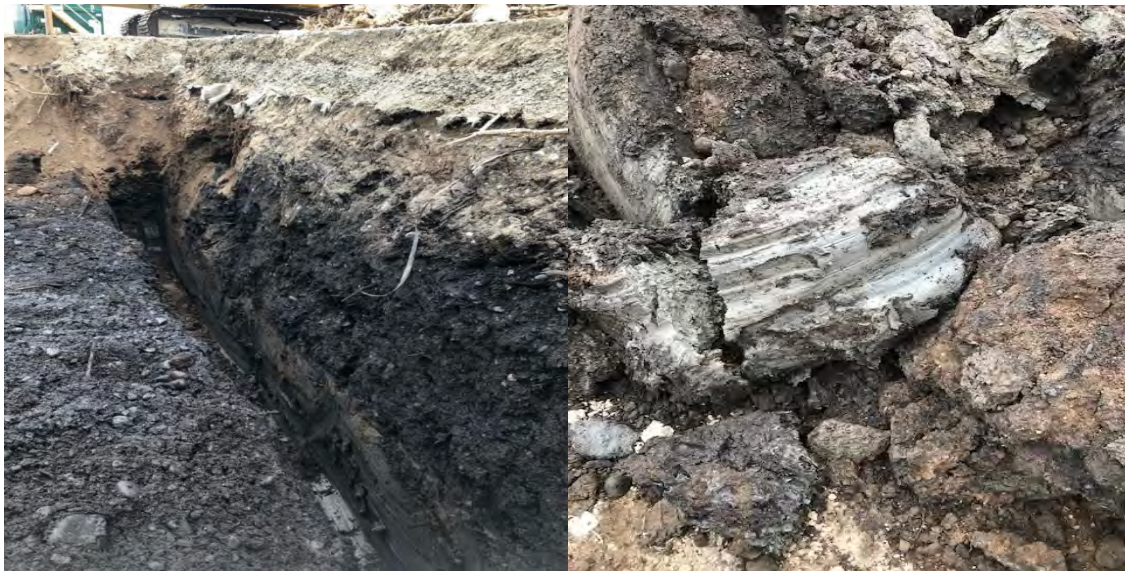
Figure 10: Trench prior to filling with Clay
