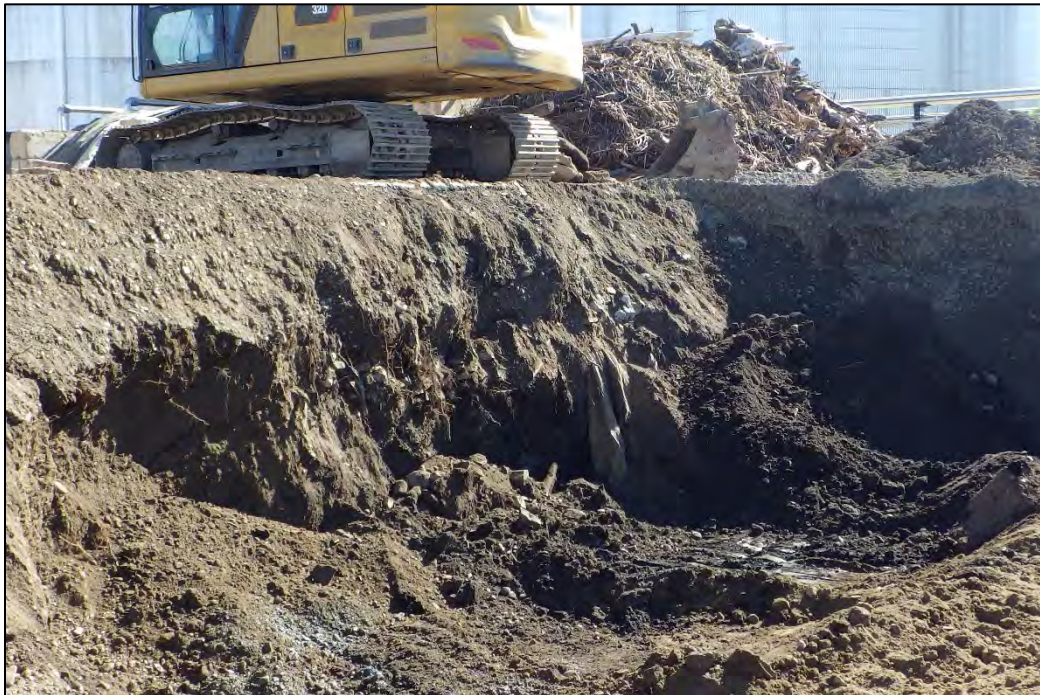
Figure 5-5. Overview of RAU B14 with modern debris within berm, facing east.
