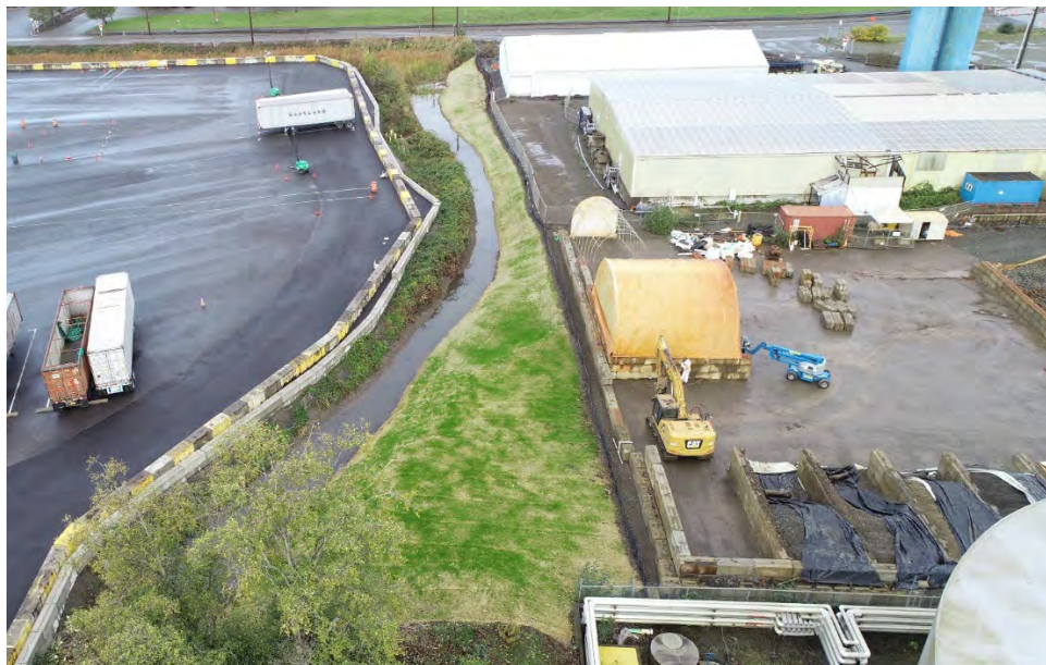
Figure 14: Aerial View 10 days after hydroseeding
