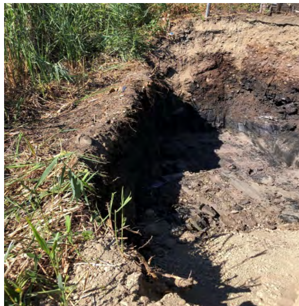
Figure 17: Bottom of RAU B1. Note oil staining in headwall
