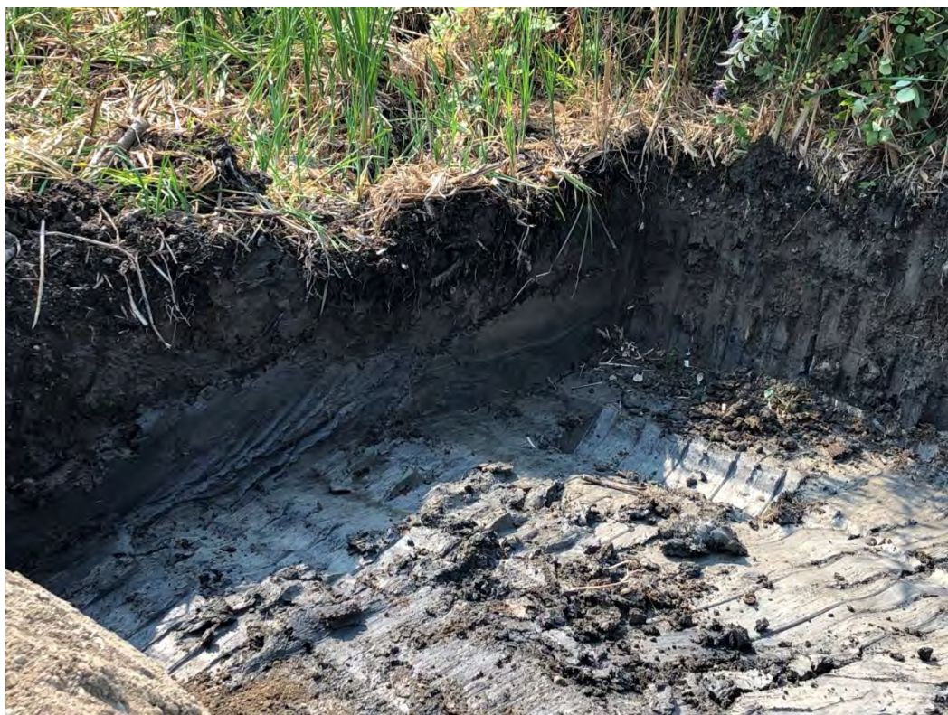
Figure 39: Bottom of RAU D2 NOTE: Three foot thickness of clay-rich silt bottom
