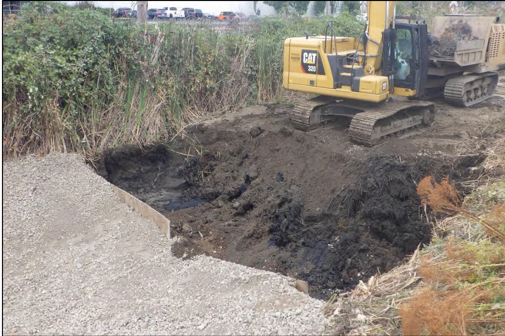
Figure 5-8. Overview of excavation within RAU D-19 during remediation clean up. Blackened sediments visible at bottom of unit, view northwest.
