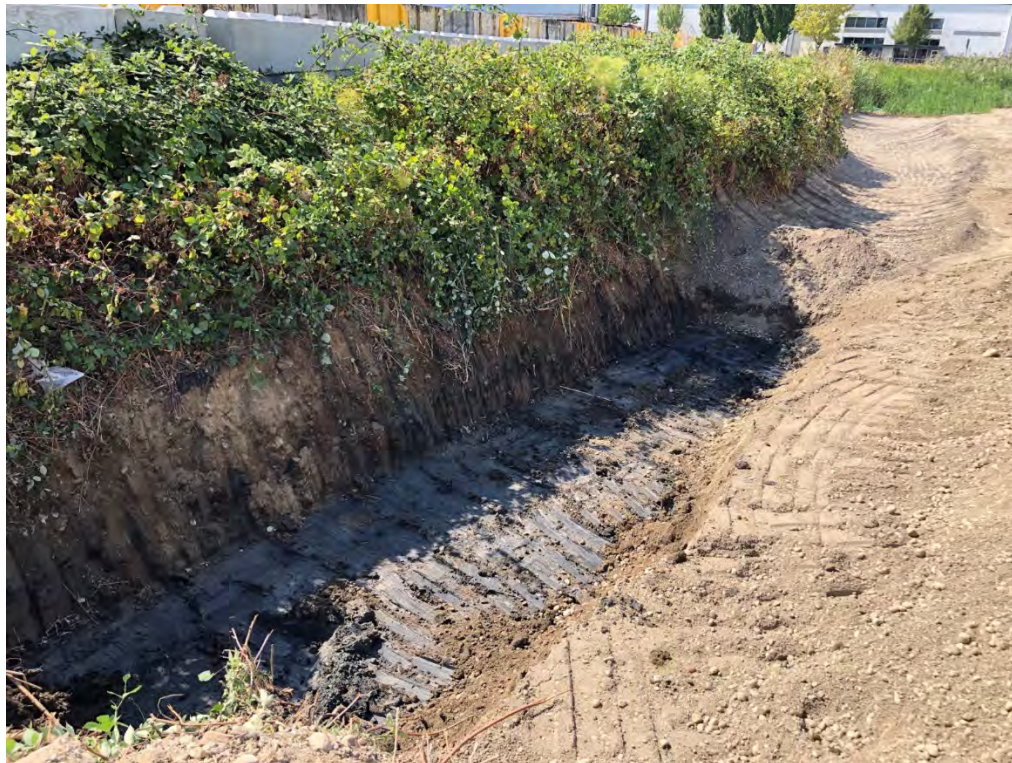
Figure 44: Bottom and western sidewall of RAU D7
