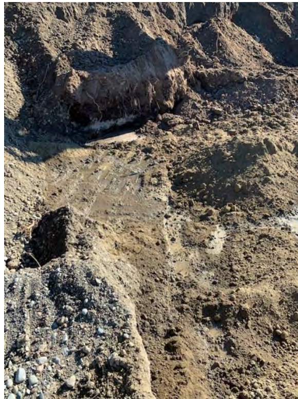
Figure 36: Excavation of RAU B14 - Note Waste water sludge as white band in sidewall
