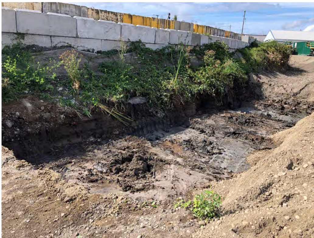
Figure 47: Bottom and western sidewall of RAU D10
