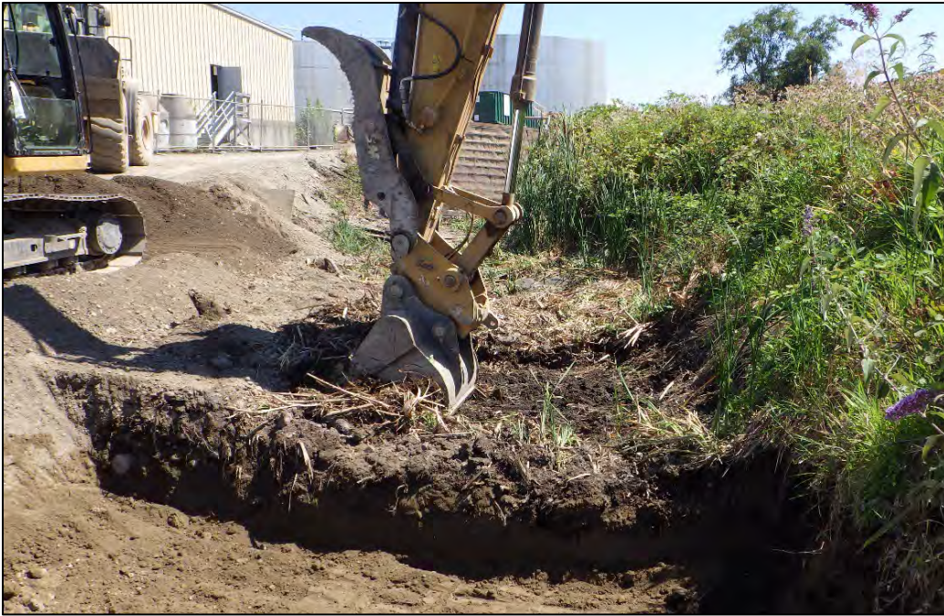
Figure 5-1. Overview of initial vegetation removal of RAU-D4, facing east.
