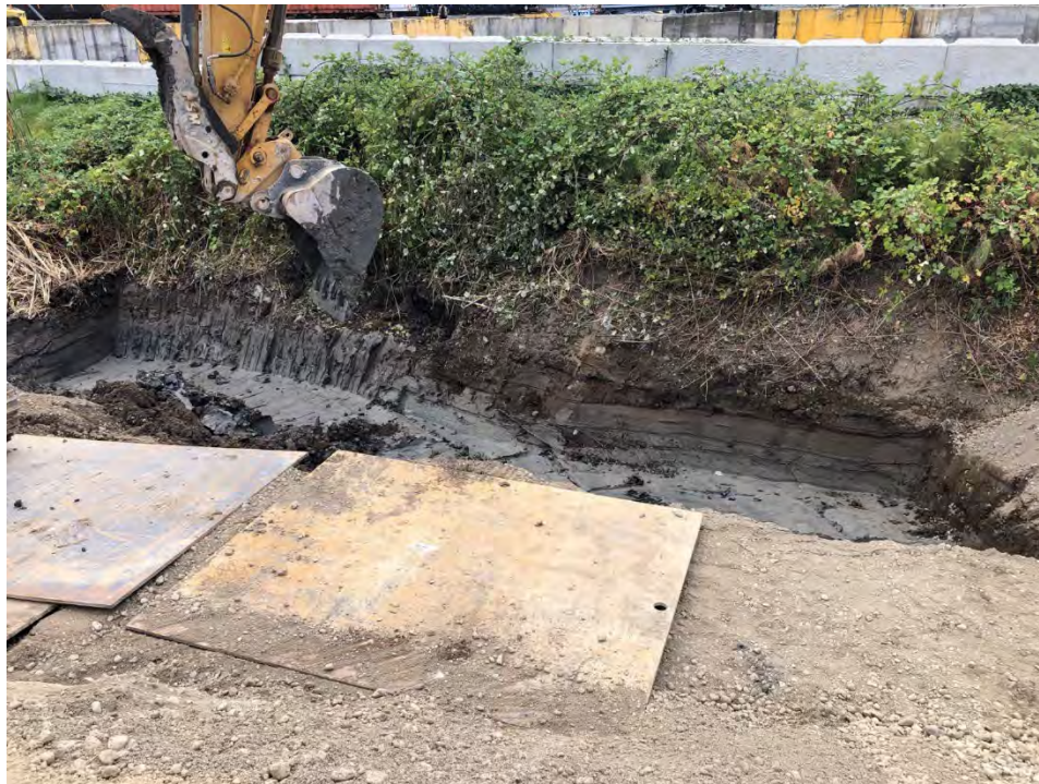
Figure 7: Eastern excavation limit
