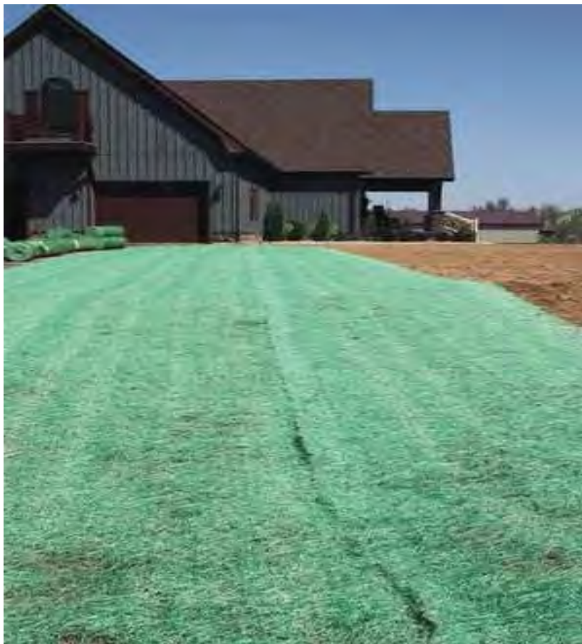
Figure 12: Stock Photograph – Bio-gradable Erosion Control Netting (Product Installed)
