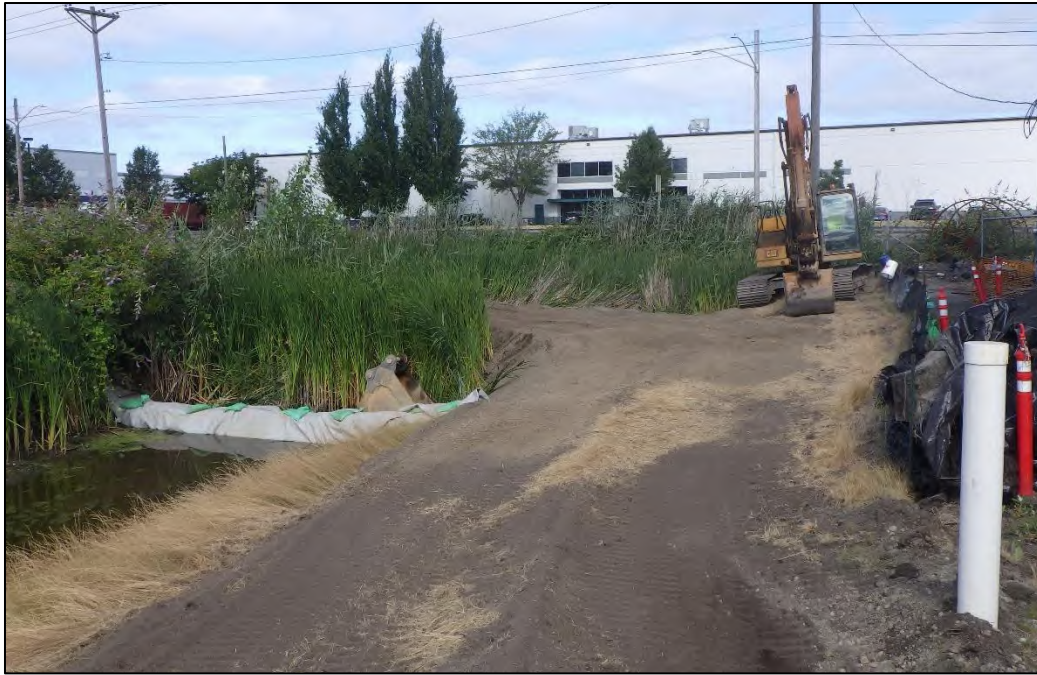
Figure 5-2. Overview of sandbag dam and access road construction in the northern portion of the APE, view west.
