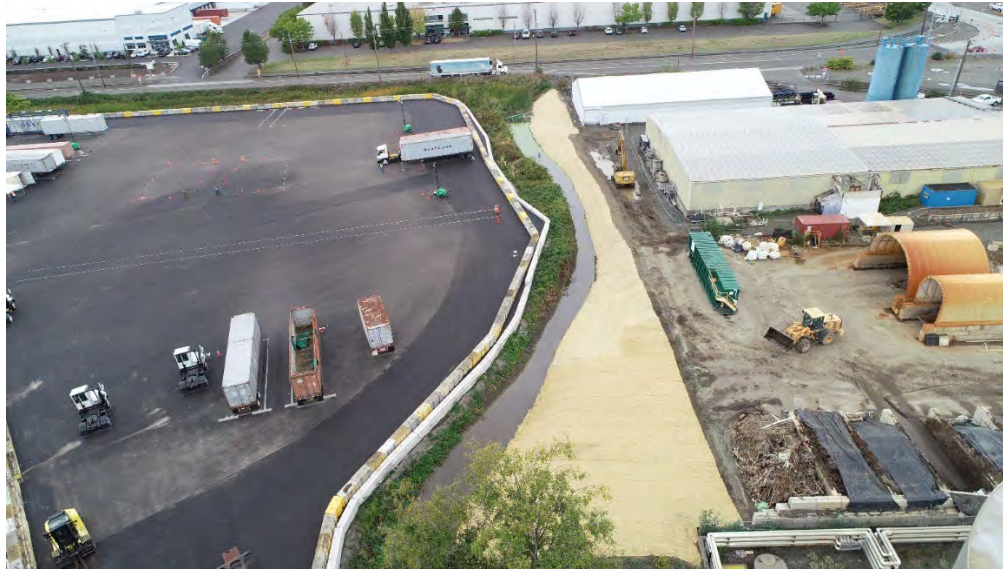
Figure 13: Aerial view of straw mat prior to hydroseeding
