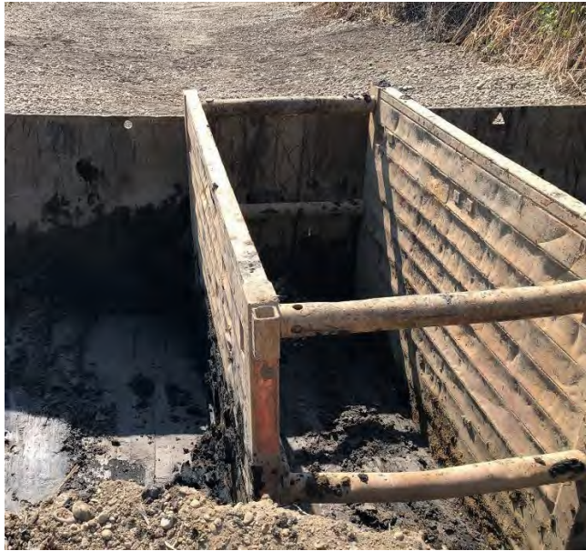
Figure 13: Use of a Trench Box and Steel Sheeting to Ensure that All Impacted Soils Are Removed and to Prevent Caving.
