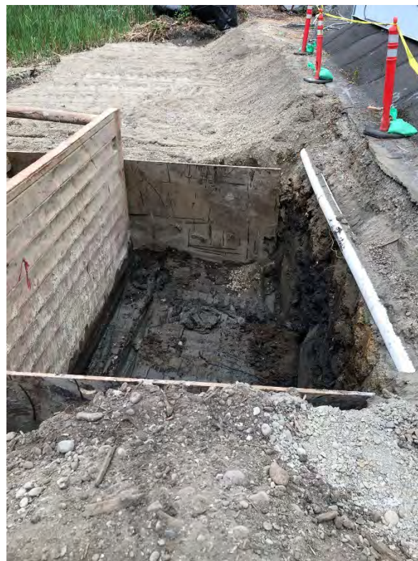
Figure 26: Use of steel plates and trench box to prevent caving
