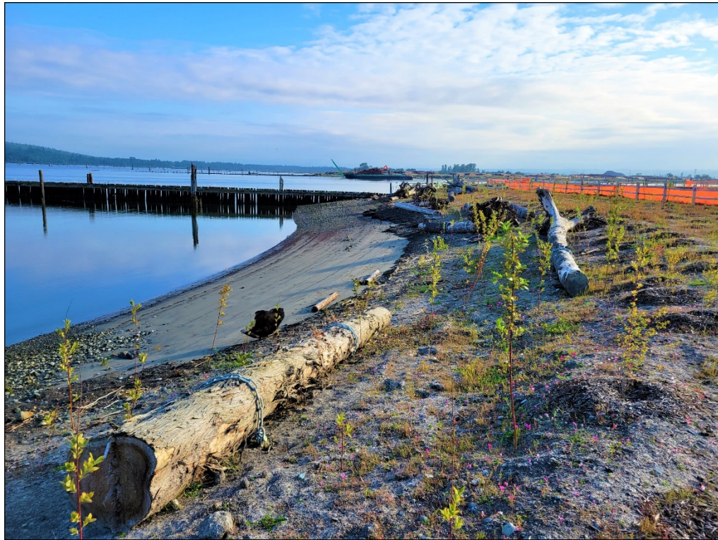
Shoreline Restoration Plantings Photograph C
