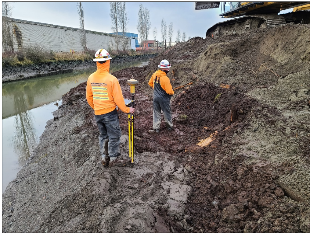
Shoreline Restoration Photograph F
