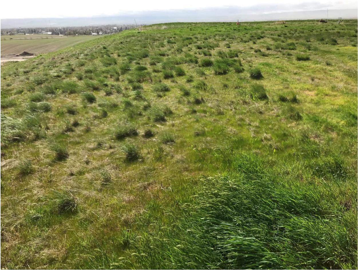
Photo 3 Photo showing condition of cap over part of Area 6 during an inspection for the periodic review.
