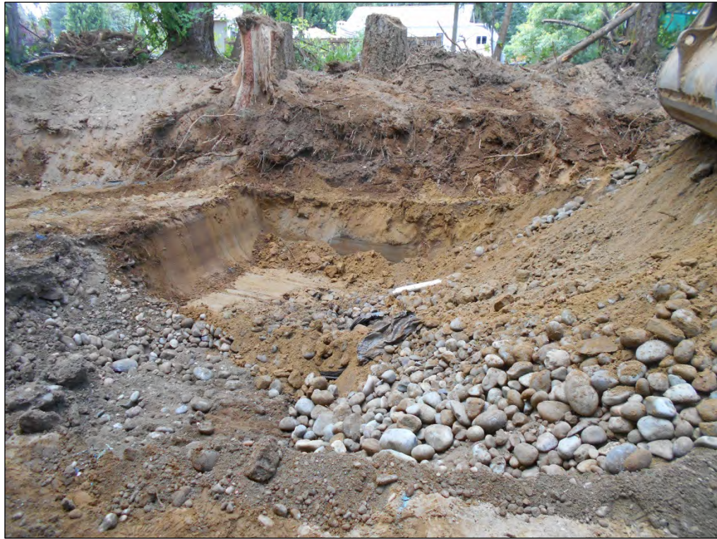
3. Looking south at the Site; uncovering 1996 excavation area backfill.
