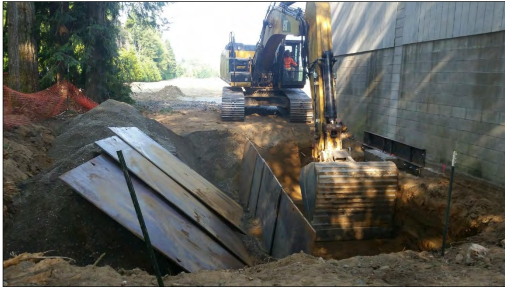
7. Looking west at the Site; excavating Slots A through D.
