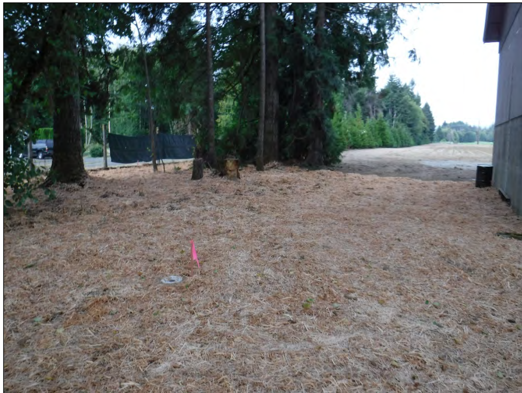
10. Looking west at the Site; Site restoration and new monitoring well locations.
