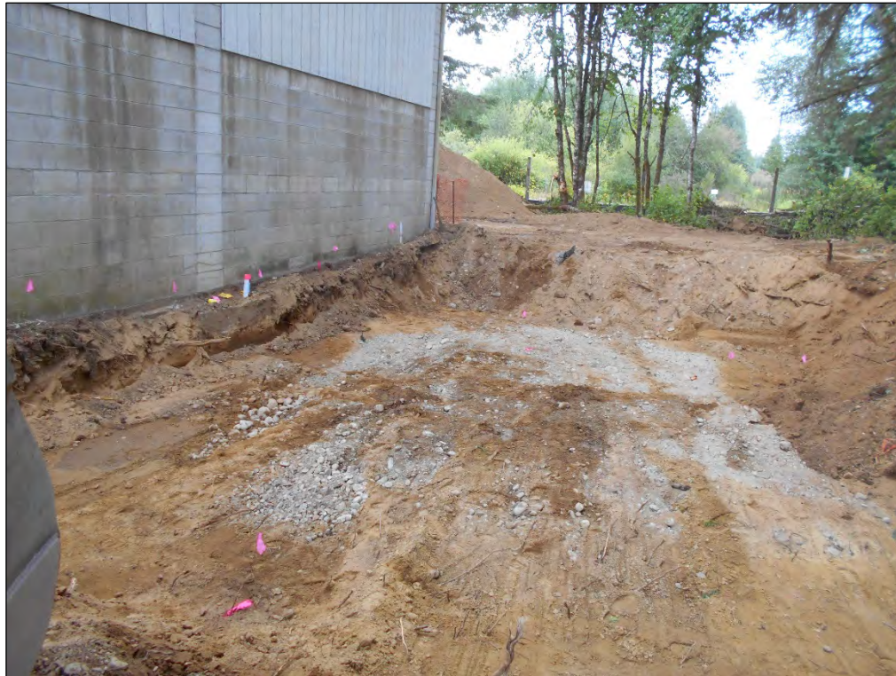
2. Looking northeast at the Site; removal of clean overburden.
