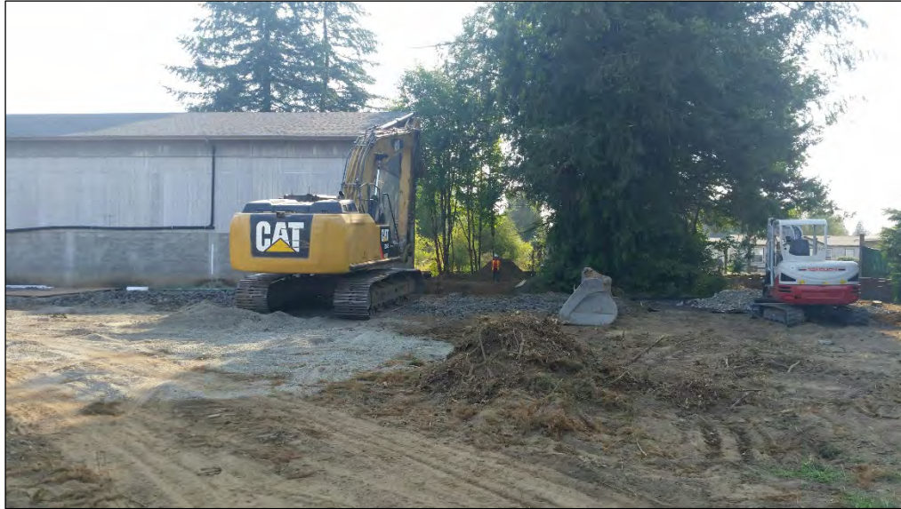
1. Looking east at the Site; beginning excavation activities.
