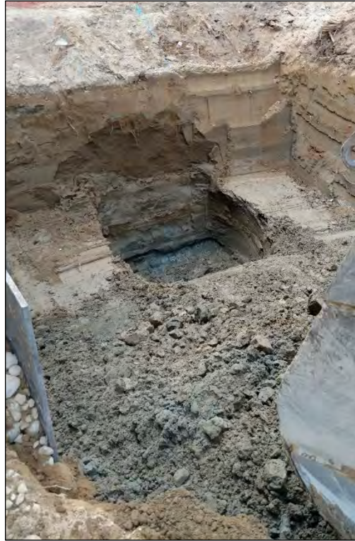
5. Looking east at the Site; reaching final depth at Slot E.
