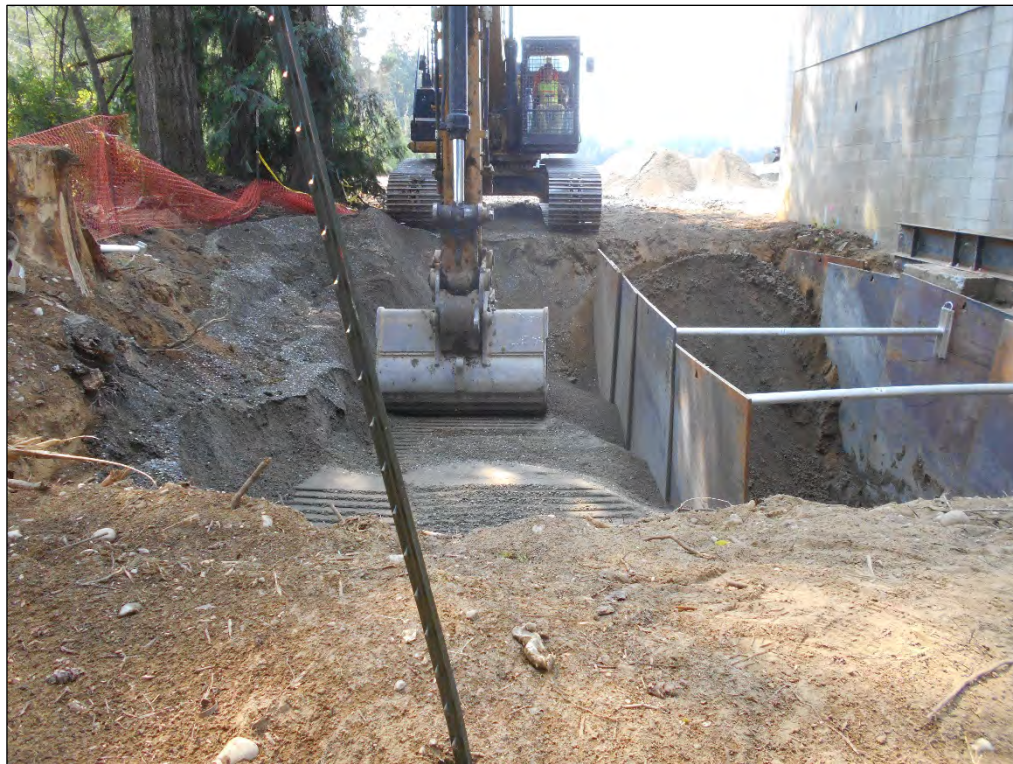
6. Looking west at the Site; slots supported using sheet pile walls.
