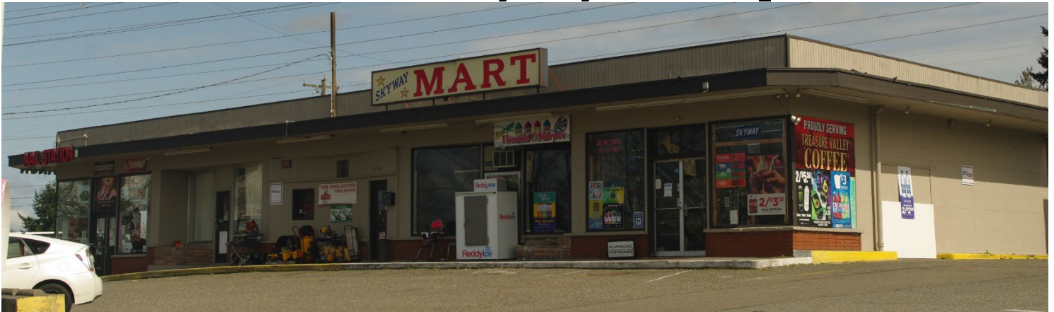
Boathouse Inc Renton Skyway Cleanup Site (12548 Renton Ave. S., Seattle)
