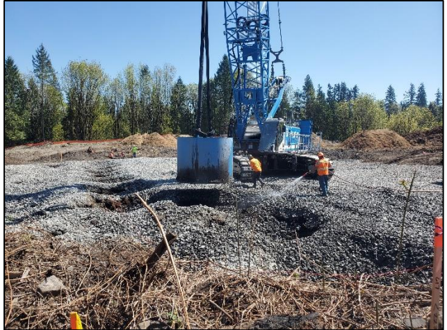
Dynamic compaction at northeast end of detention pond. Looking east.
