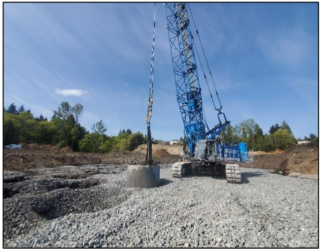
Dynamic compaction at southeast end of detention pond. Looking northwest.
