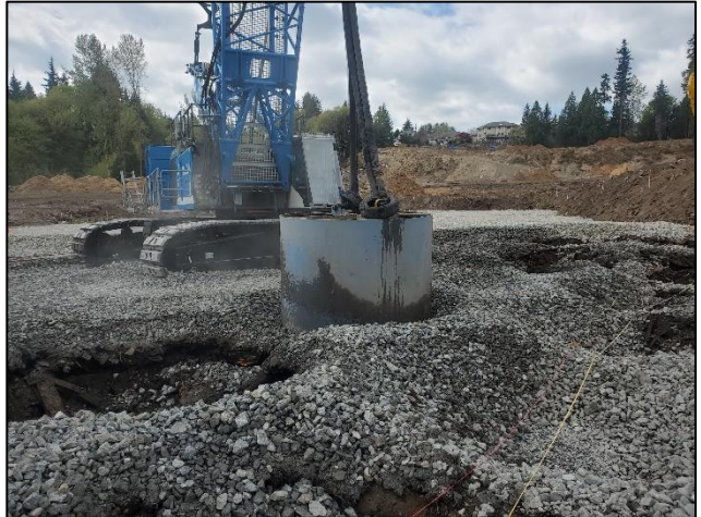
Dynamic compaction at north end of detention pond. Looking southwest.
