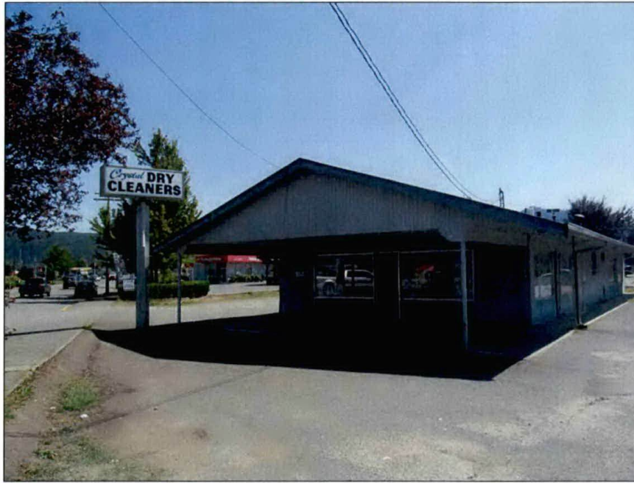
Photograph 1: View of the Site, facing southeast.
