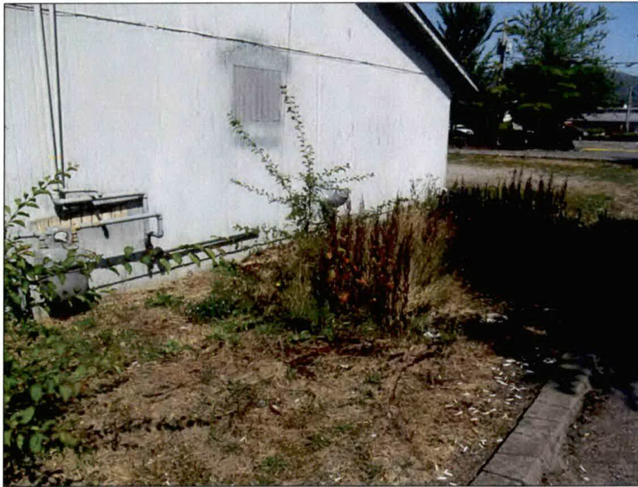
Photograph 17: View of vegetated area south of the building.
