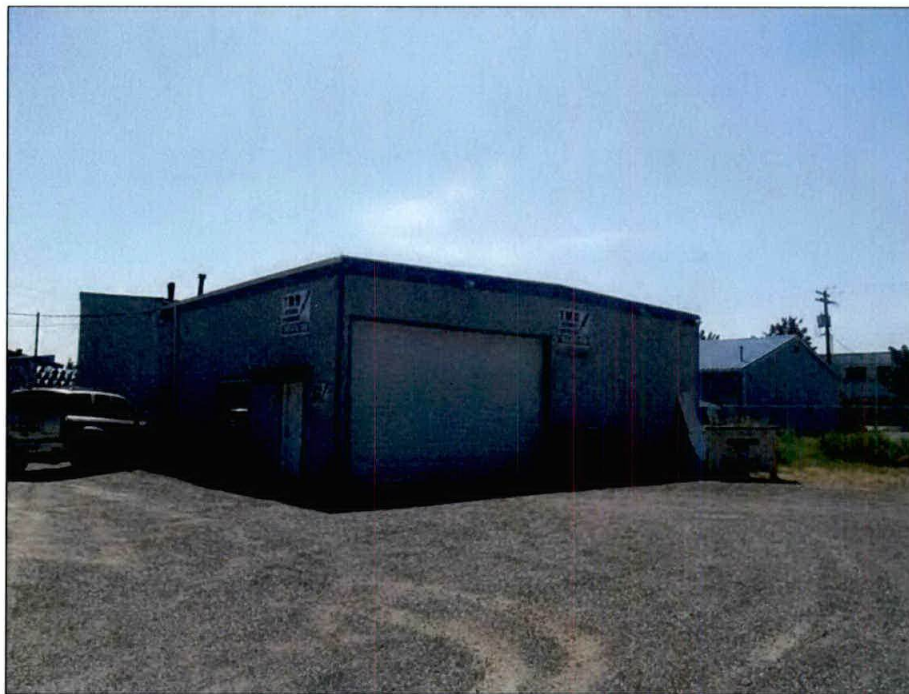
Photograph 7: View of west-adjointing electrical contractor.
