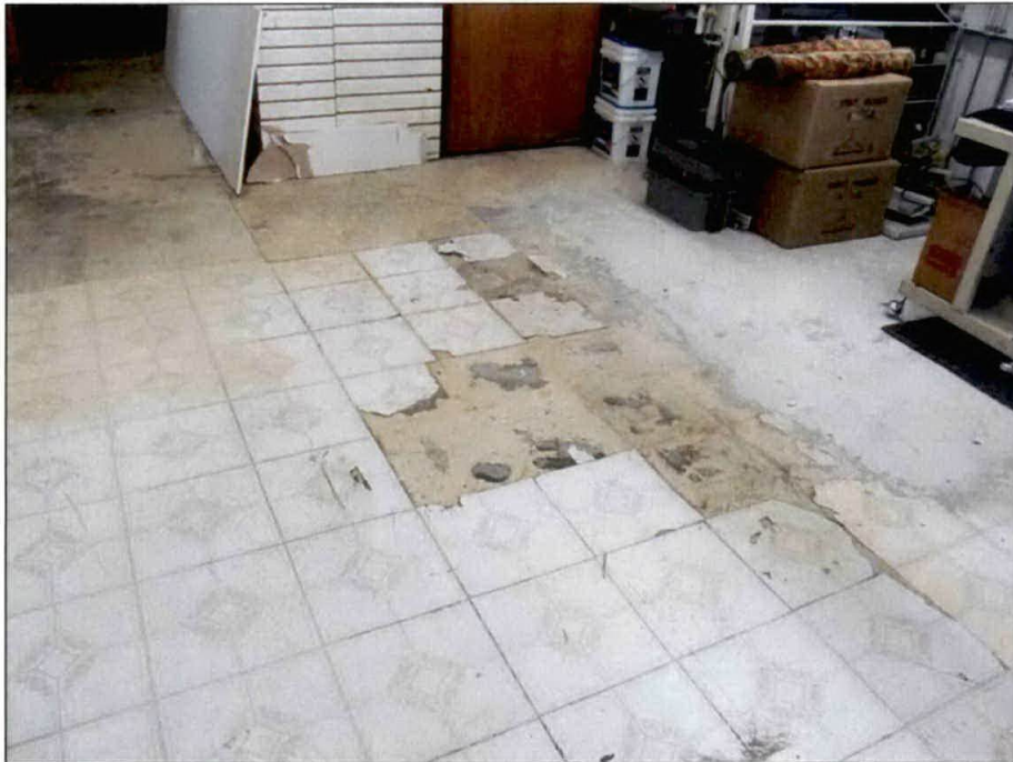
Photograph 14: View of floor near dry-cleaning machine.
