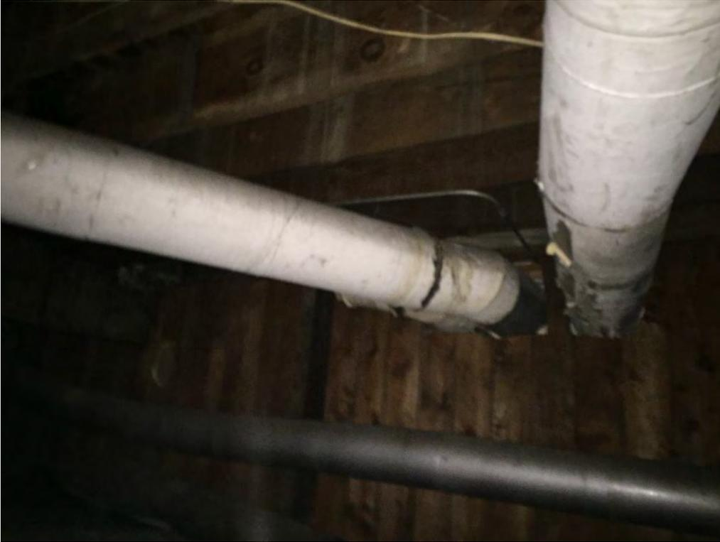
Photo 11: - ACM duct insulation found in the basement of 5021 Rainier Avenue South.
