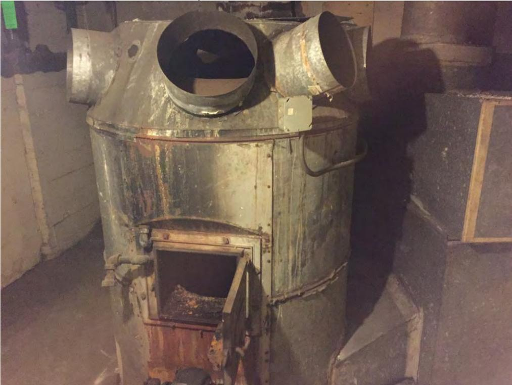
Photo 10: Old boiler observed in the auto repair mechanical room. The white tape is ACM.
