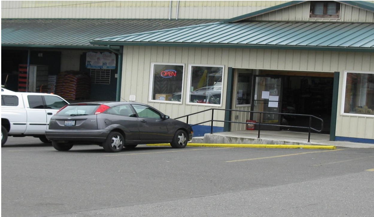
Photo 1: Side of the store and asphalt cap – from the Northwest.
