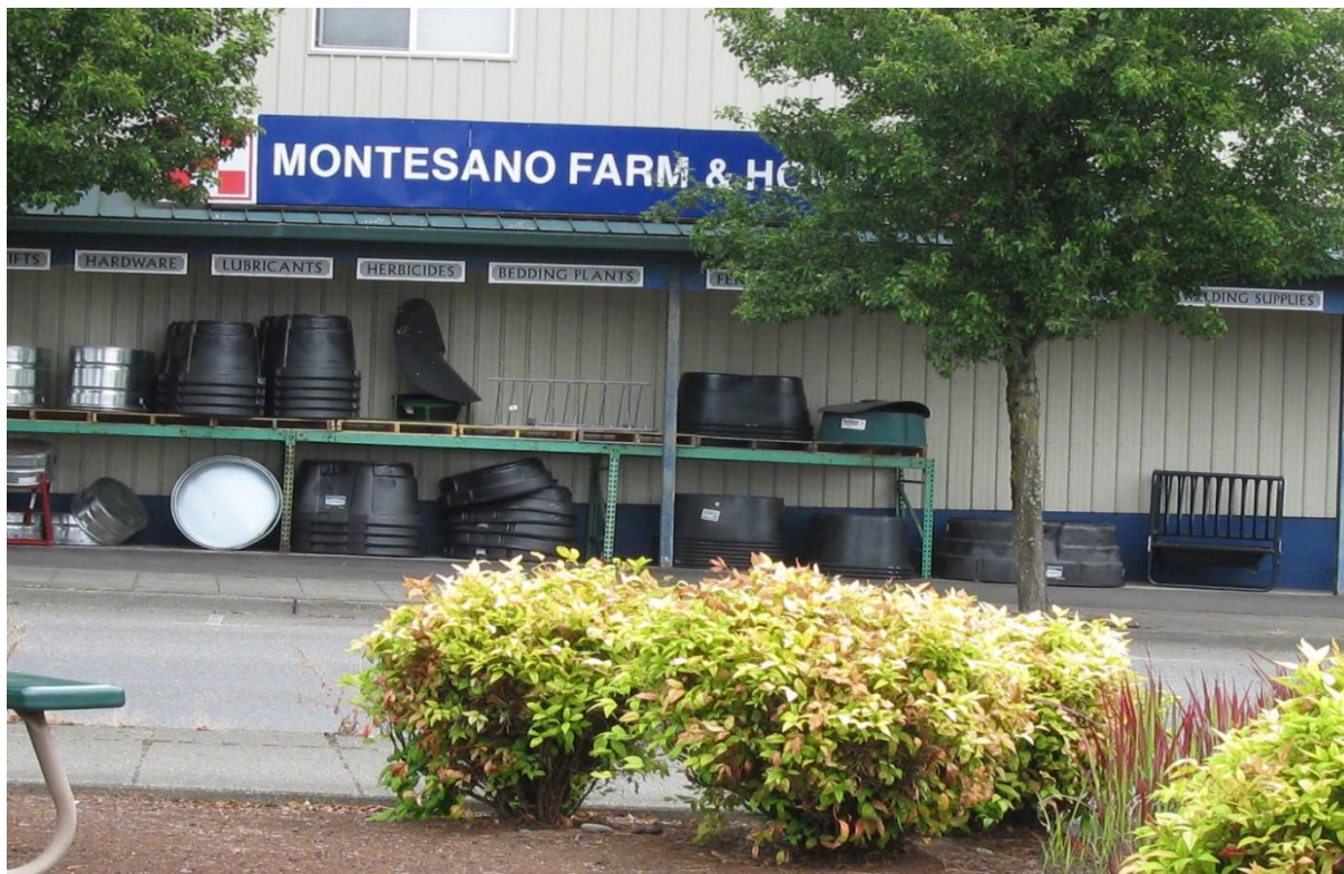
Photo 8: Store building and Main Street – from the Southwest.
