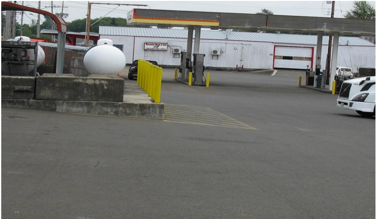
Photo 3: Parking lot/asphalt cap, pump islands and propane above ground tanks –from the West.
