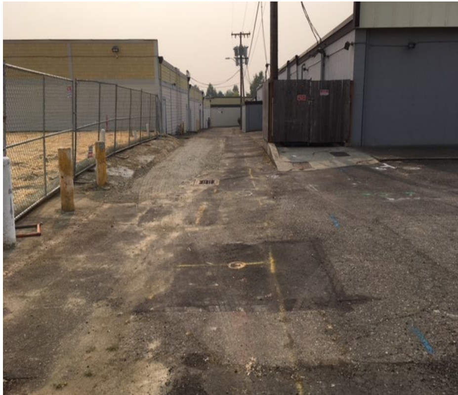
Photo 30 11.15.2018. Alley. Former Building C (fenced) to left. View South.
