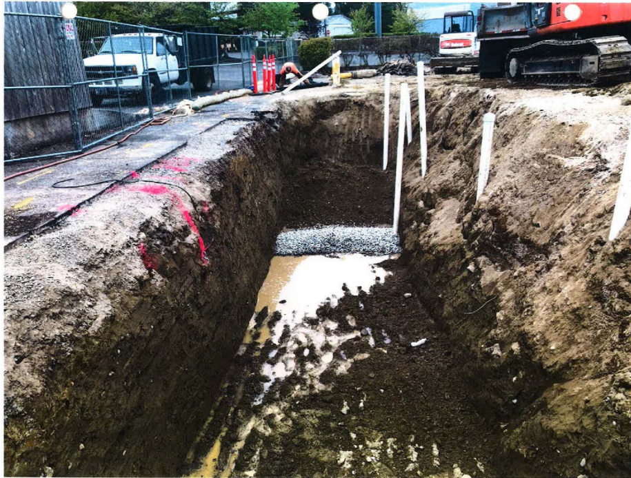
Photo 19 - Setting 4-inch PVC treatment pipe in excavation. View North
