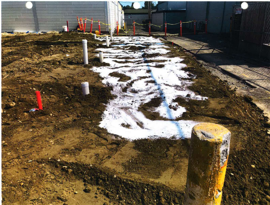
Photo 28 - Applying Klozur to excavated soil in lifts. View South.
