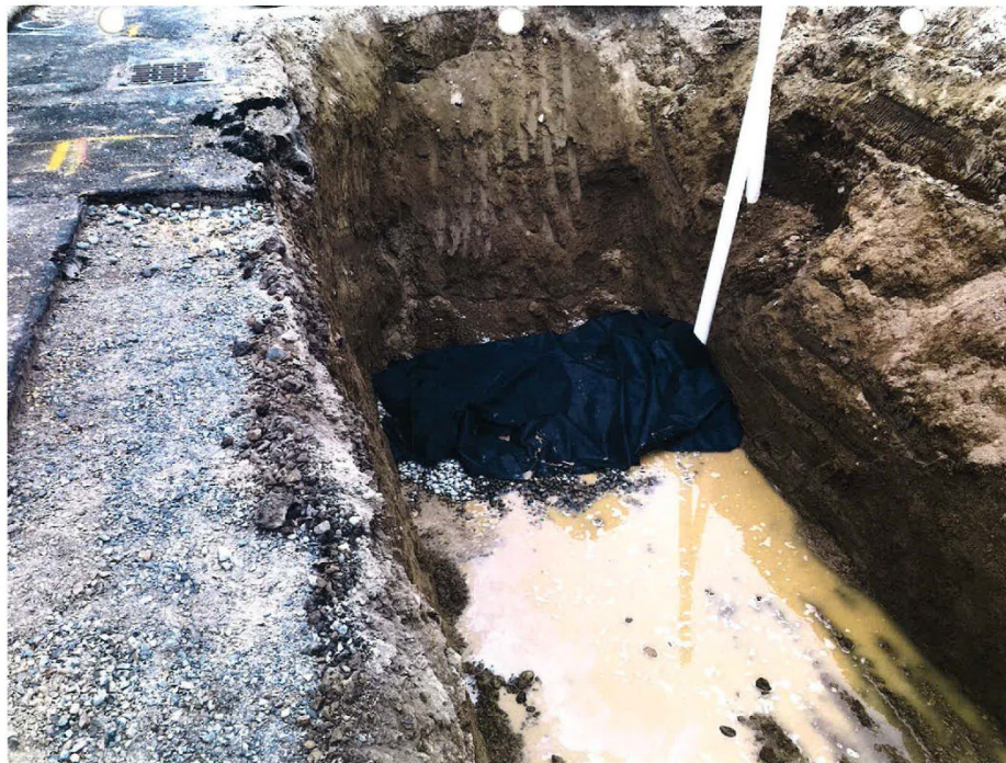
Photo 18 Setting 4-inch PVC treatment pipe in excavation. View North.
