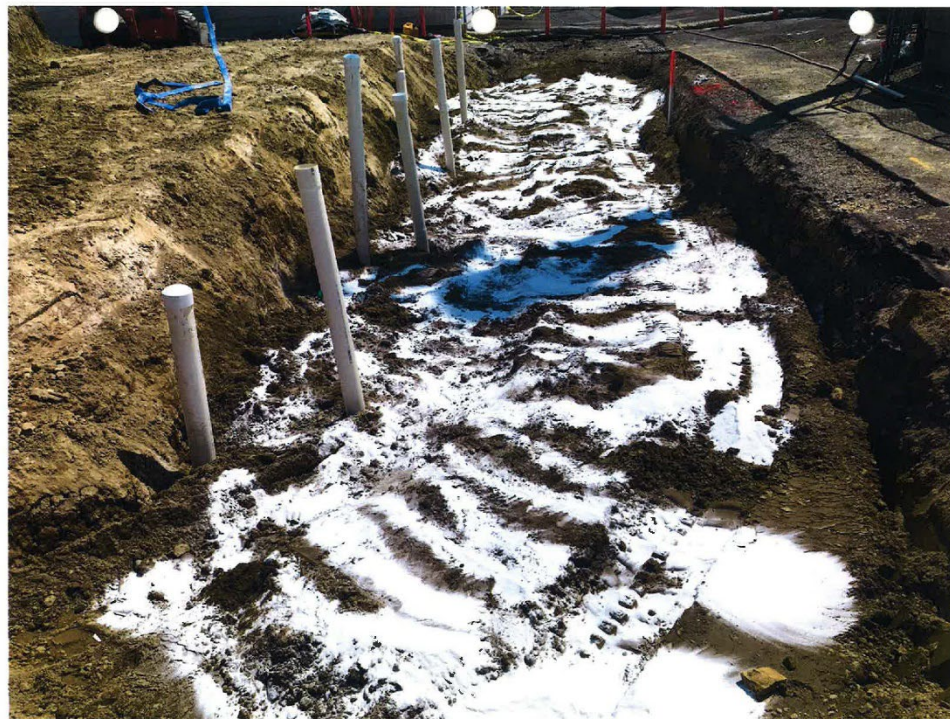
Photo 26 - Applying Klozur to excavated soil in lifts. View South.
