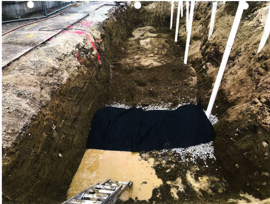
Photo 24 - Setting 4-inch PVC treatment pipe in excavation. View North
