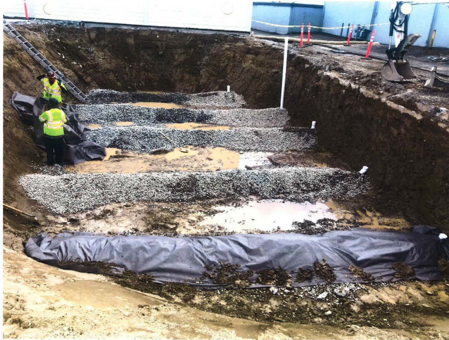
Photo 9 May 11, 2018. PVC treatment pipes bedded in drain rock. View North.
