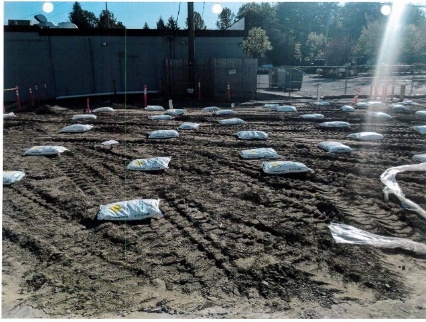
Photo 15 May 12, 2018. Preparing treatment for final excavated soil lift. View West.
