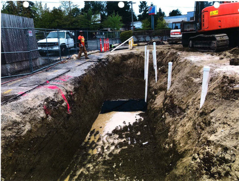
Photo 20 - Setting 4-inch PVC treatment pipe in excavation. View North
