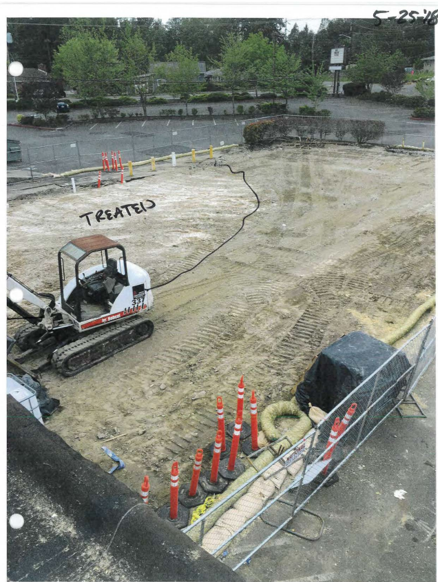
Photo 16 May 25, 2018. View NW of completed soil treatment area from Building B.
