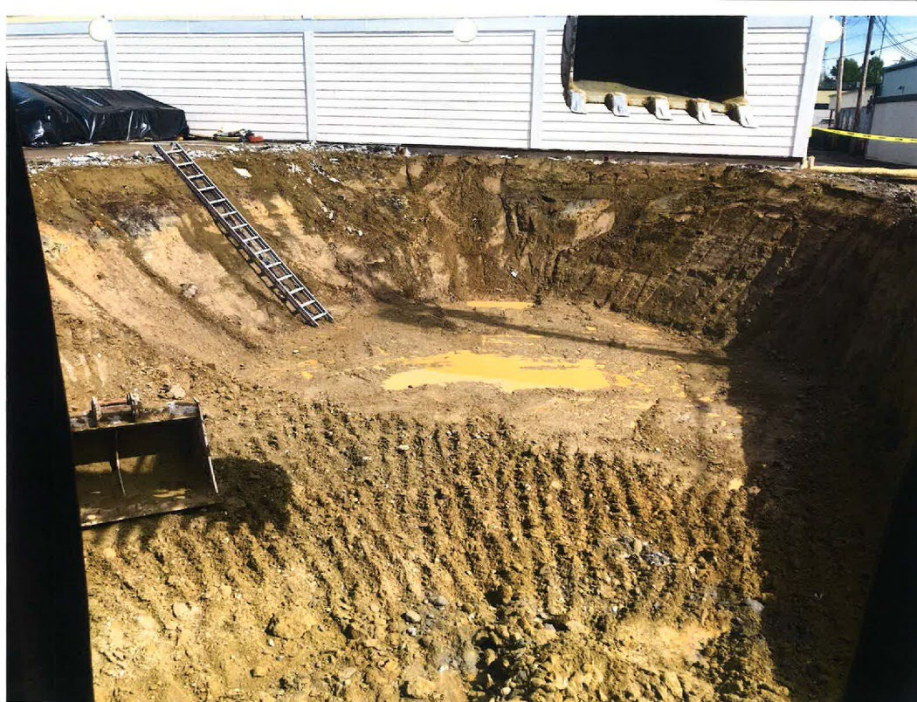
Photo 5 May 10, 2018. Former Building C excavation. View South
