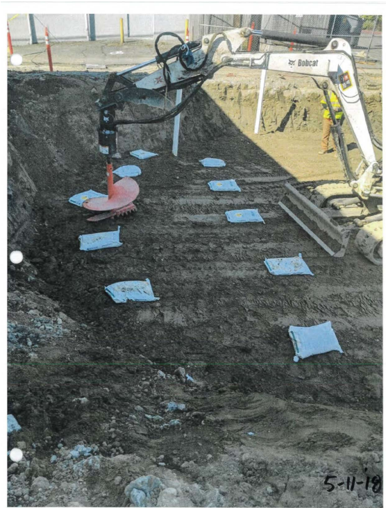
Photo 11 May 11, 2018. Mixing Klozur into excavated soil lift w/ auger head. View W
