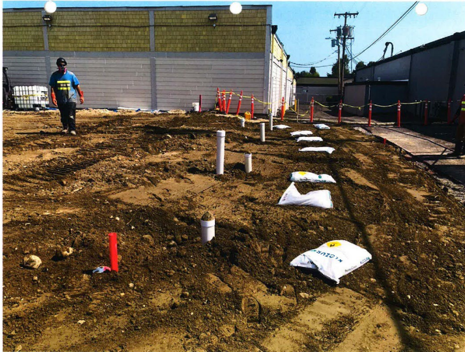
Photo 27 - Applying Klozur to excavated soil in lifts. View South.
