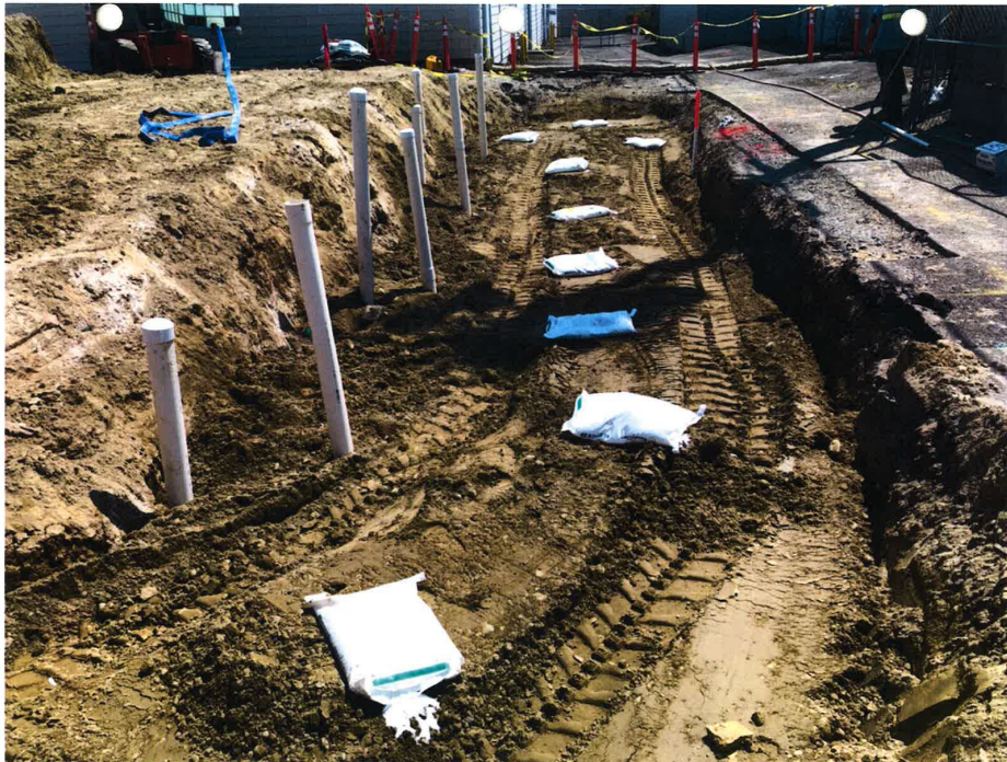
Photo 25 - Applying Klozur to excavated soil in lifts. View South.
