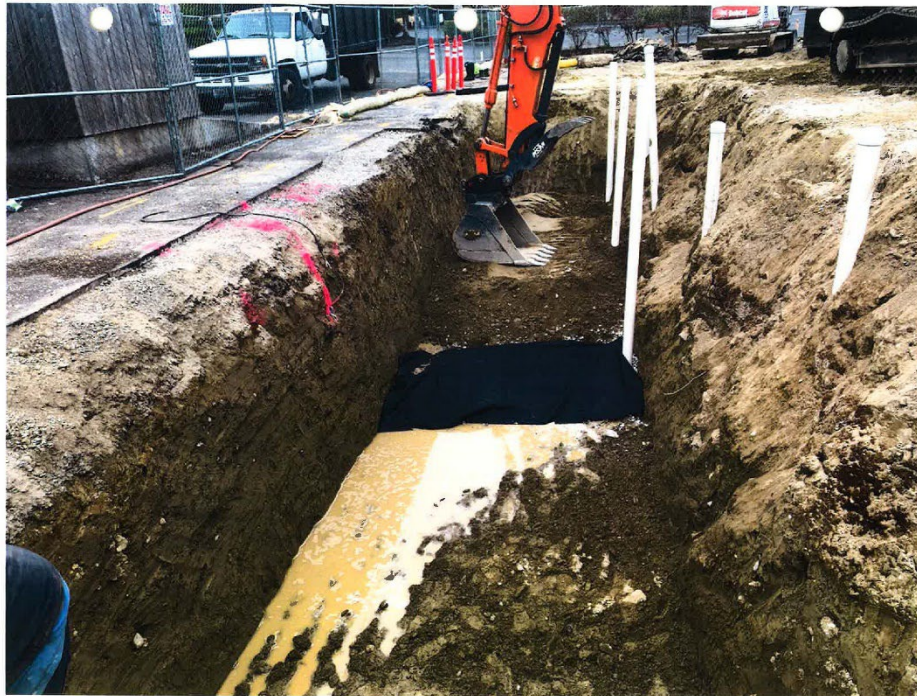
Photo 22 - Setting 4-inch PVC treatment pipe in excavation. View North
