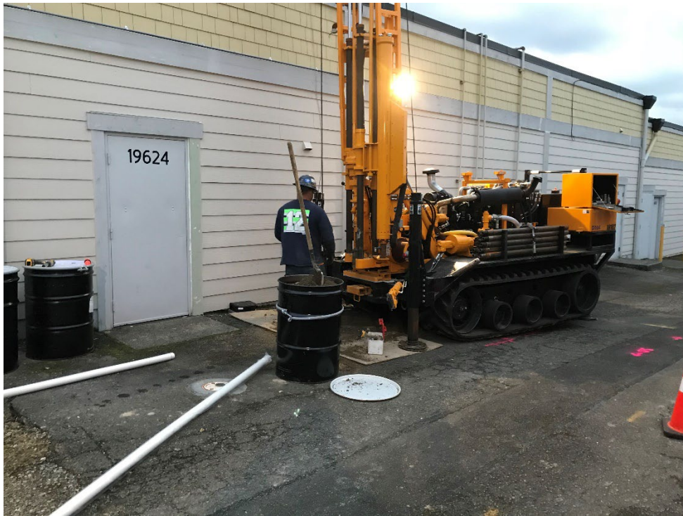
Photo 31 11.15.2018. Installing MW-7A in Alley. View Southeast.
