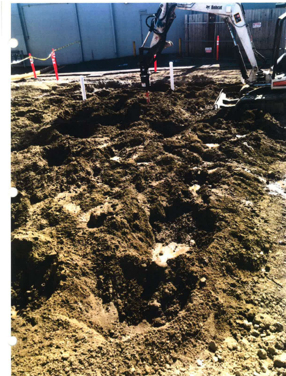
Photo 14 May 12, 2018. Auger mixing NaOH actuator into treated soil. View W
