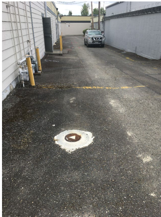
Photo 38 8.12.2020. View S in Alley from MW-7B. Building B to left, D to right
