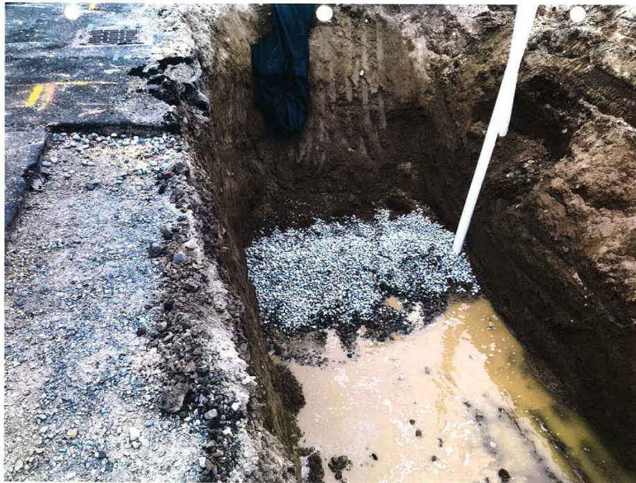
Photo 17 Aug 2018 Alley area soil excavation to approx. 6 feet bgs. View North.
