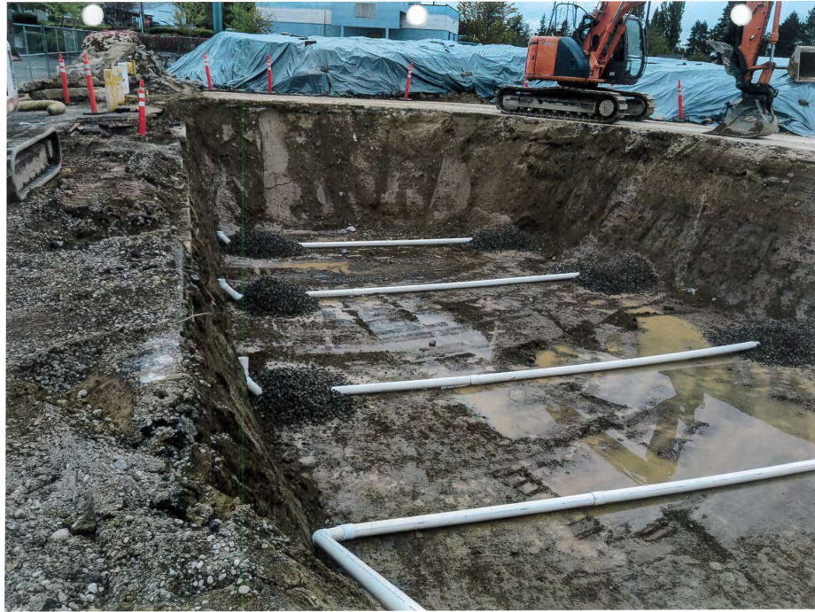
Photo 7 May 11, 2018. Building C excavation with pipes, covered soil pile. View N
