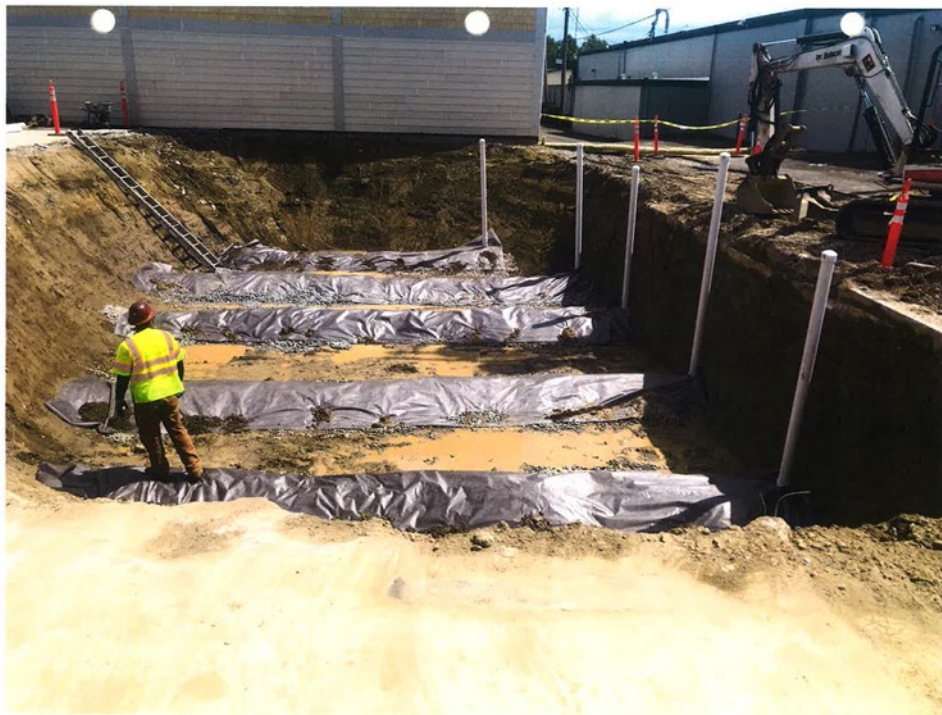
Photo 10 May 11, 2018. PVC pipes & drain rock covered with geotextile. View N
