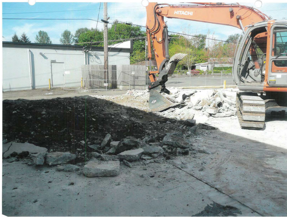
Photo 1 May 2018. Removing concrete slab at Building C excavation. View NW
