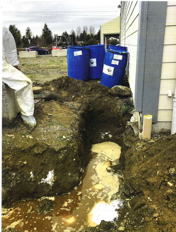
Photo 32 11.23.2019. Trench treatment applications. View East.
