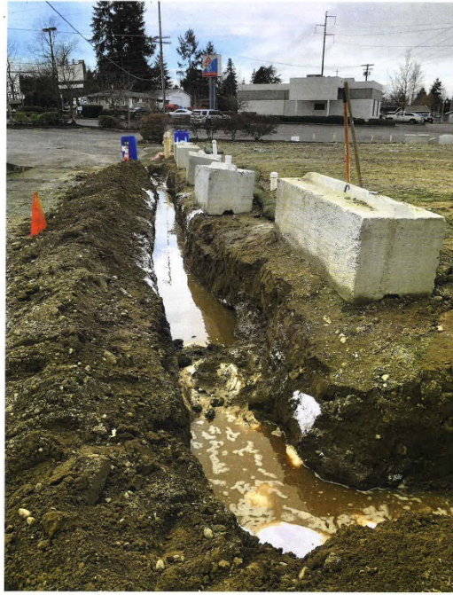
Photo 33 11.23.2019. Trench treatment application. View North.
