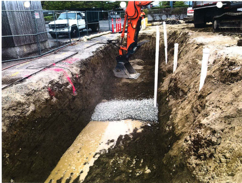
Photo 21 - Setting 4-inch PVC treatment pipe in excavation. View North
