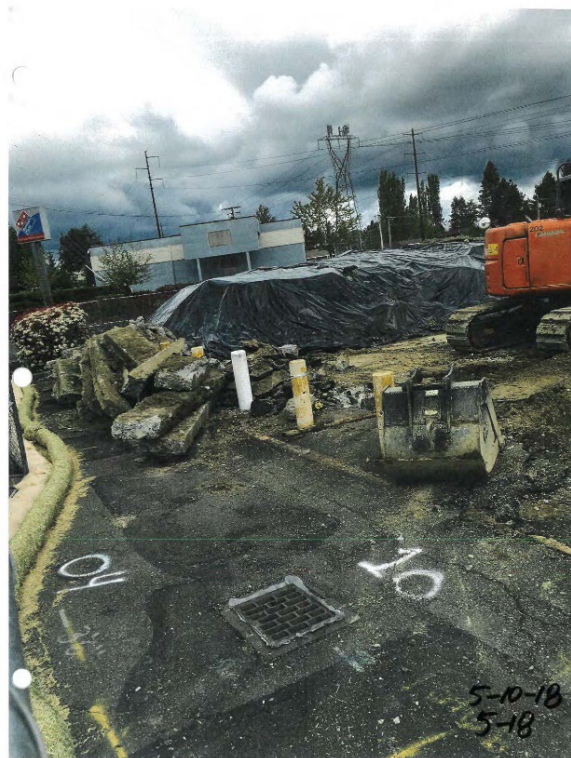
Photo 4 May 10, 2018. Stockpile covered with black plastic. View N
