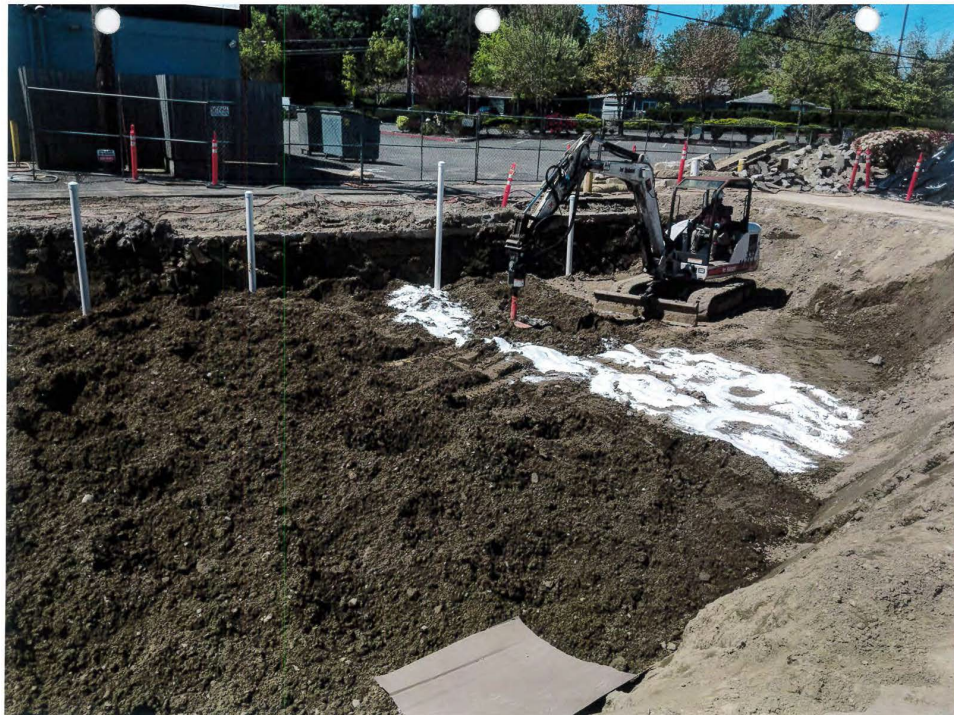
Photo 11 May 11, 2018. Mixing Klozur into excavated soil lift w/ auger head. View W
