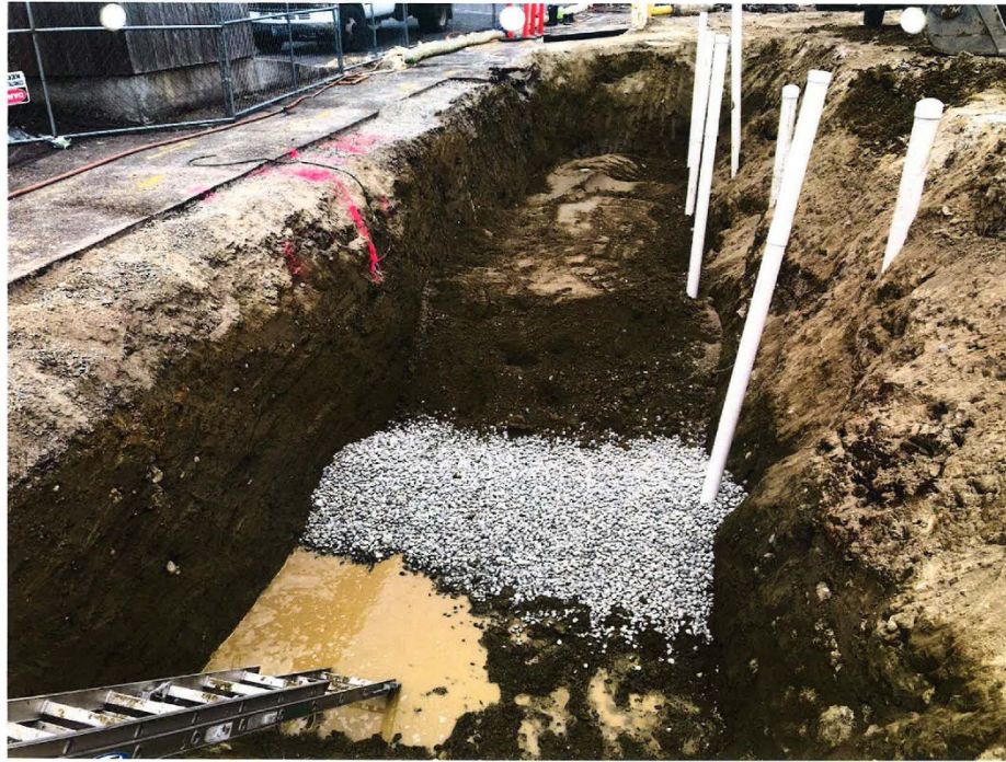
Photo 23 - Setting 4-inch PVC treatment pipe in excavation. View North
