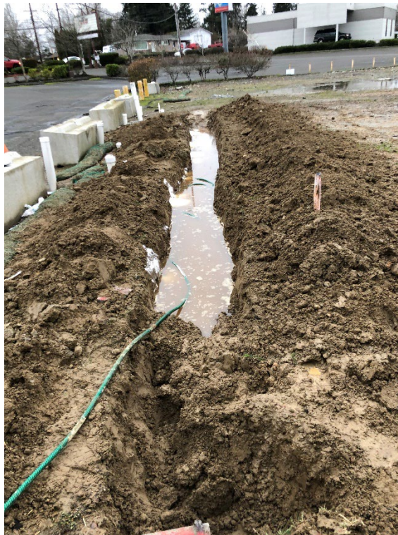
Photo 34 1.27.2020. Additional trench treatment application. View North.
