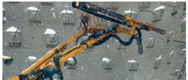
Figure 9: Drain lance installation using excavator
