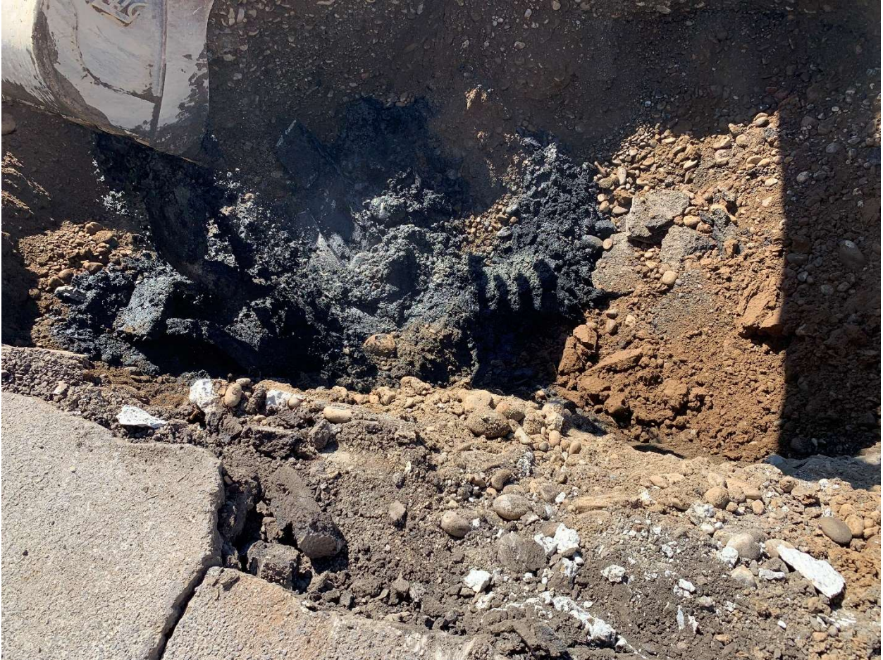
Photograph 13 – Dry Well 1 removed on July 12 2022. Dark stained PCS is evident.
