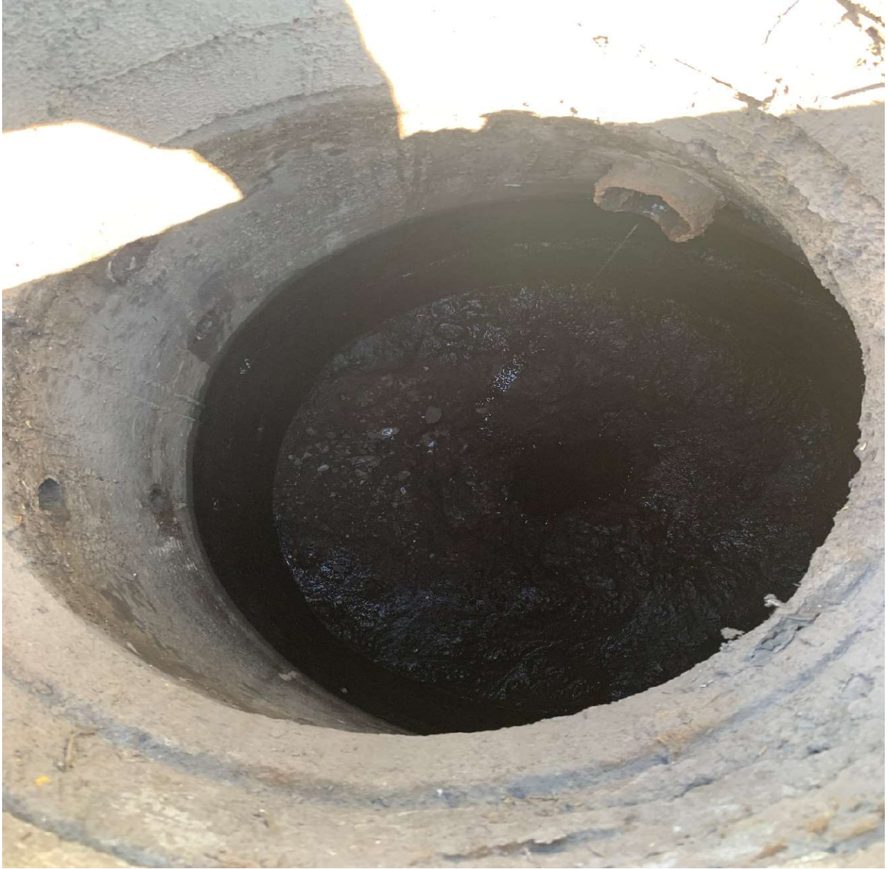
Photograph 7 – View of Dry Well 1 subsequent to liquid removal and before removal.
