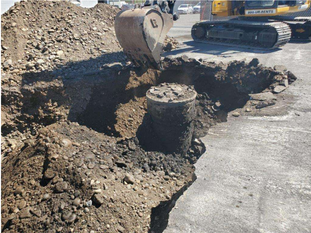
Photograph 15 – Dry Well 2 exposed during PCS excavation on July 13, 2022 (facing SE).
