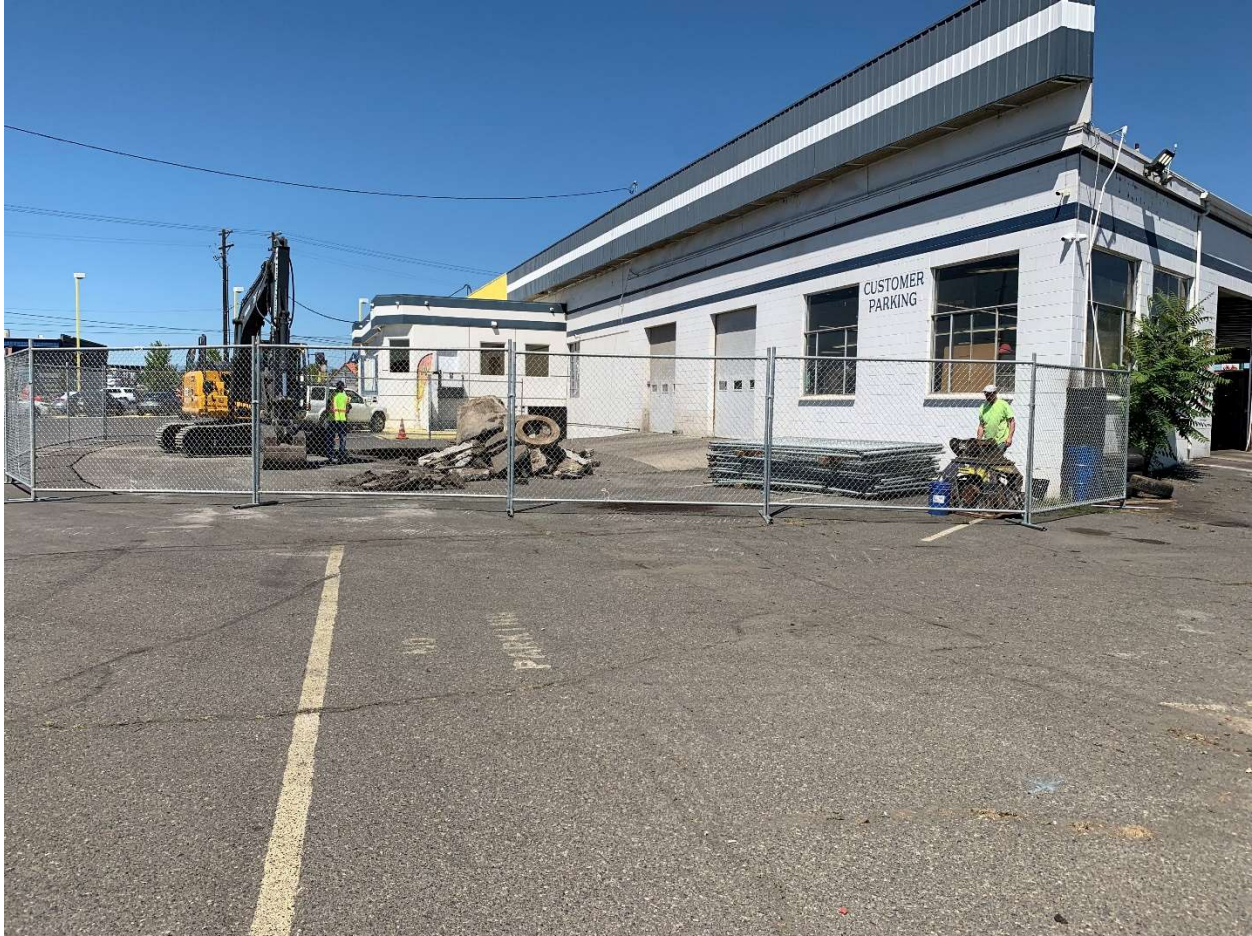
Photograph 15 – Safety fencing erected on July 12, 2022 (facing west).
