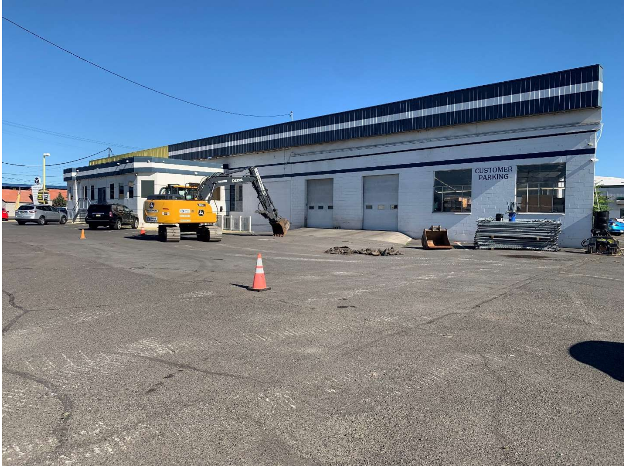
Photograph 6 – Clarke Construction beginning excavation of Dry Well 1 on July 12, 2022 (facing NW).
