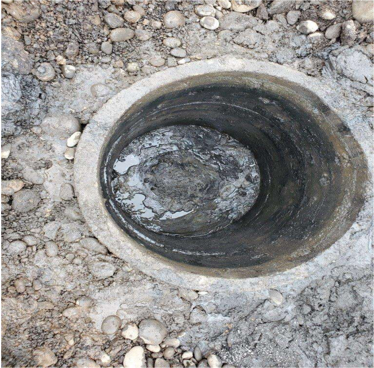
Photograph 5 – Dry Well 2 subsequent to removing liquids and some sediment on July 5, 2022.
