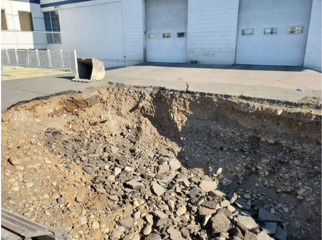
Photograph 18 – Western extent of PCS excavation trench on July 13, 2022 (facing NW).
