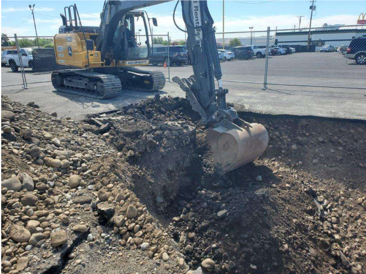
Photograph 18 – Continued excavation toward Dry Well 2 on July 13, 2022 (facing SE).
