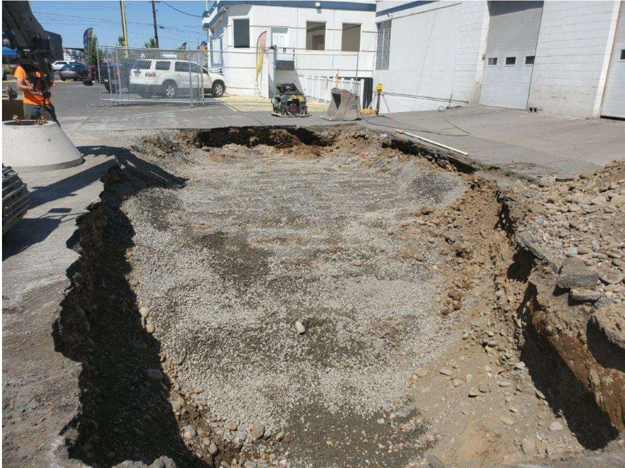
Photograph 19 – Subsequent to receipt of laboratory analysis indicating clean confirmatory soil samples, backfill and compaction on July 14, 2022 (facing west).
