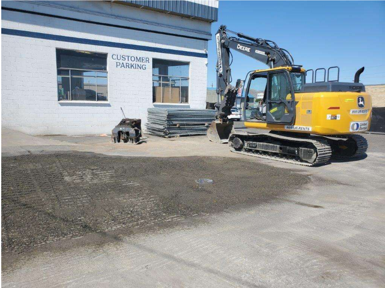
Photograph 22 – View of new dry well installed on July 14, 2022 (facing NE).
