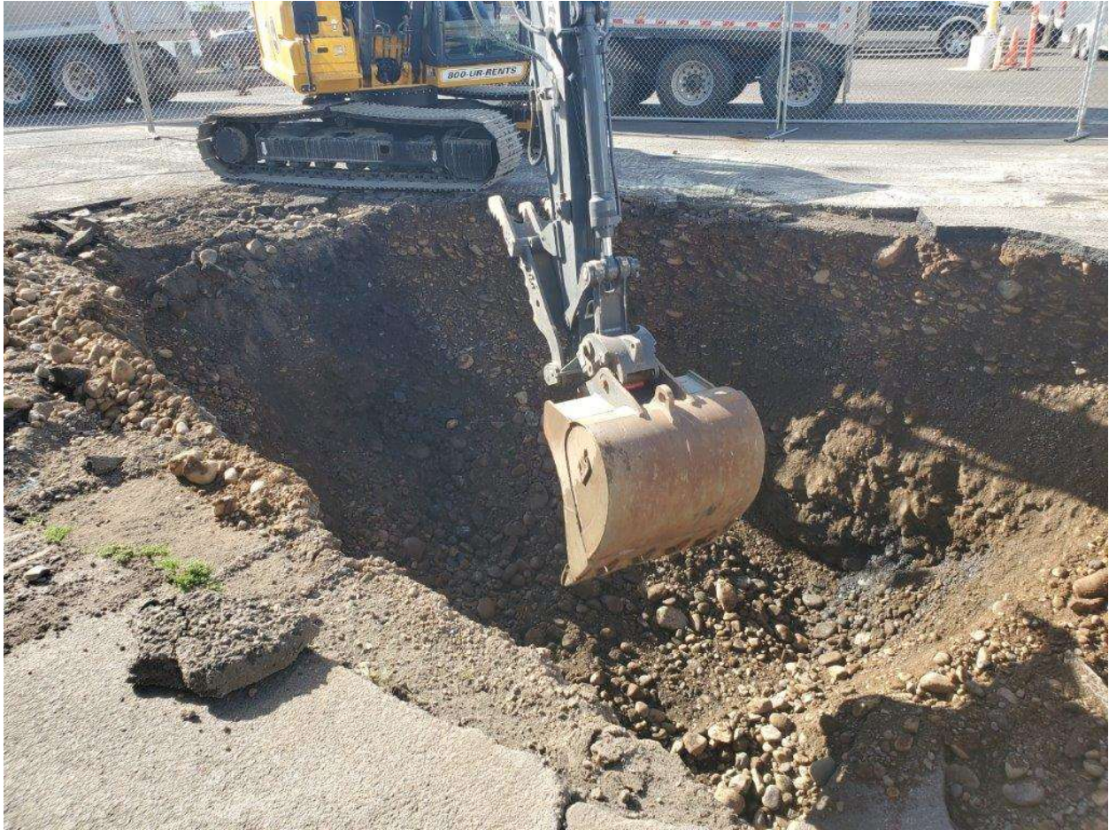
Photograph 17 – Further excavation to east toward Dry Well 2 on July 13, 2022 (facing south).
