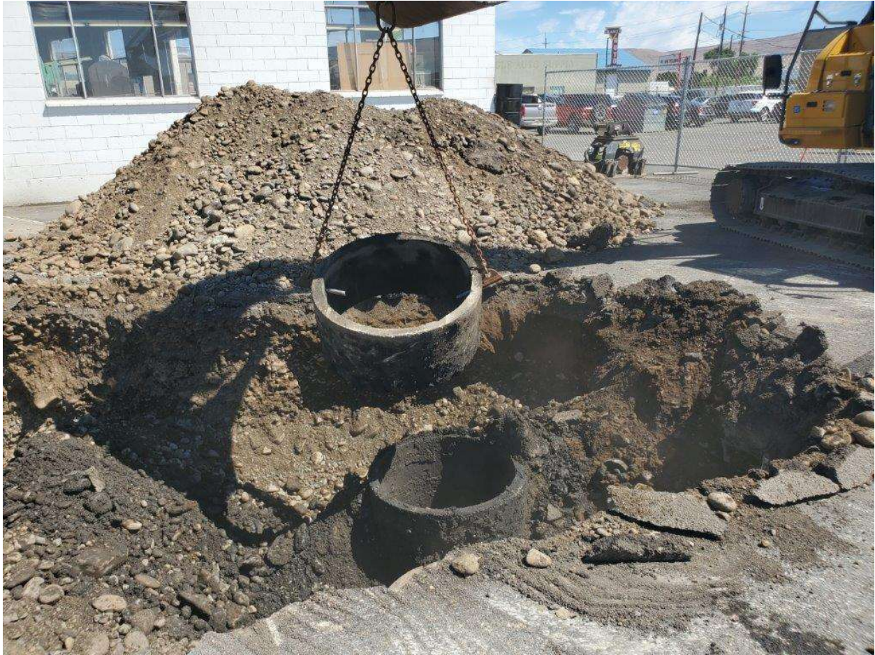
Photograph 16 – Beginning removal of Dry Well 2 on July 13, 2022 (facing NE).
