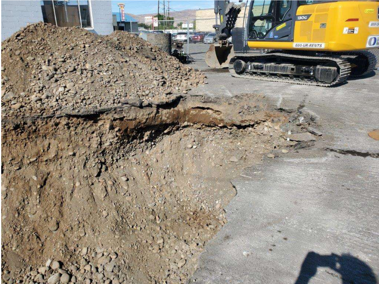
Photograph 17 – Eastern extent of PCS excavation trench on July 13, 2022 (facing NE).
