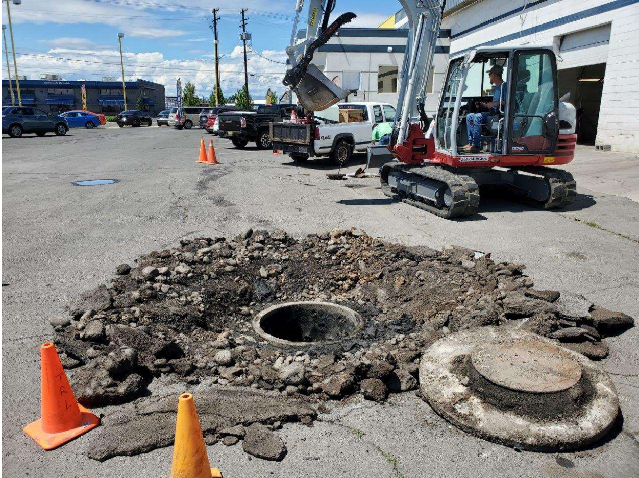
Photograph 2 – Clarke Construction personnel further assessing Dry Well 2 on July 5, 2022 (facing west).
