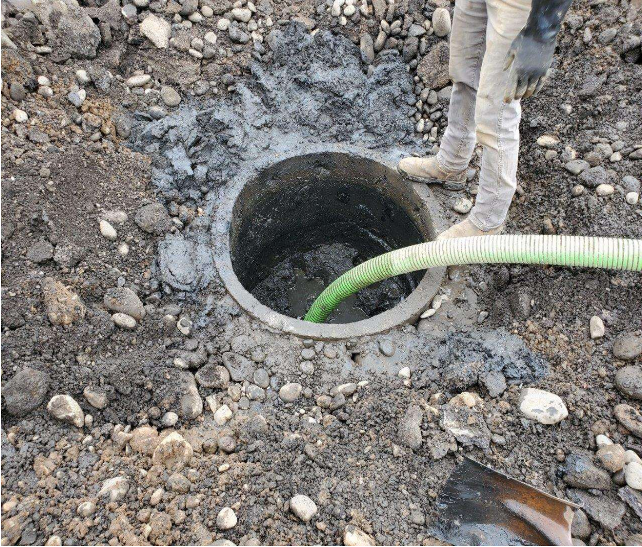
Photograph 4 – Clark Construction personnel removing liquids from Dry Well 2 on July 5, 2022.
