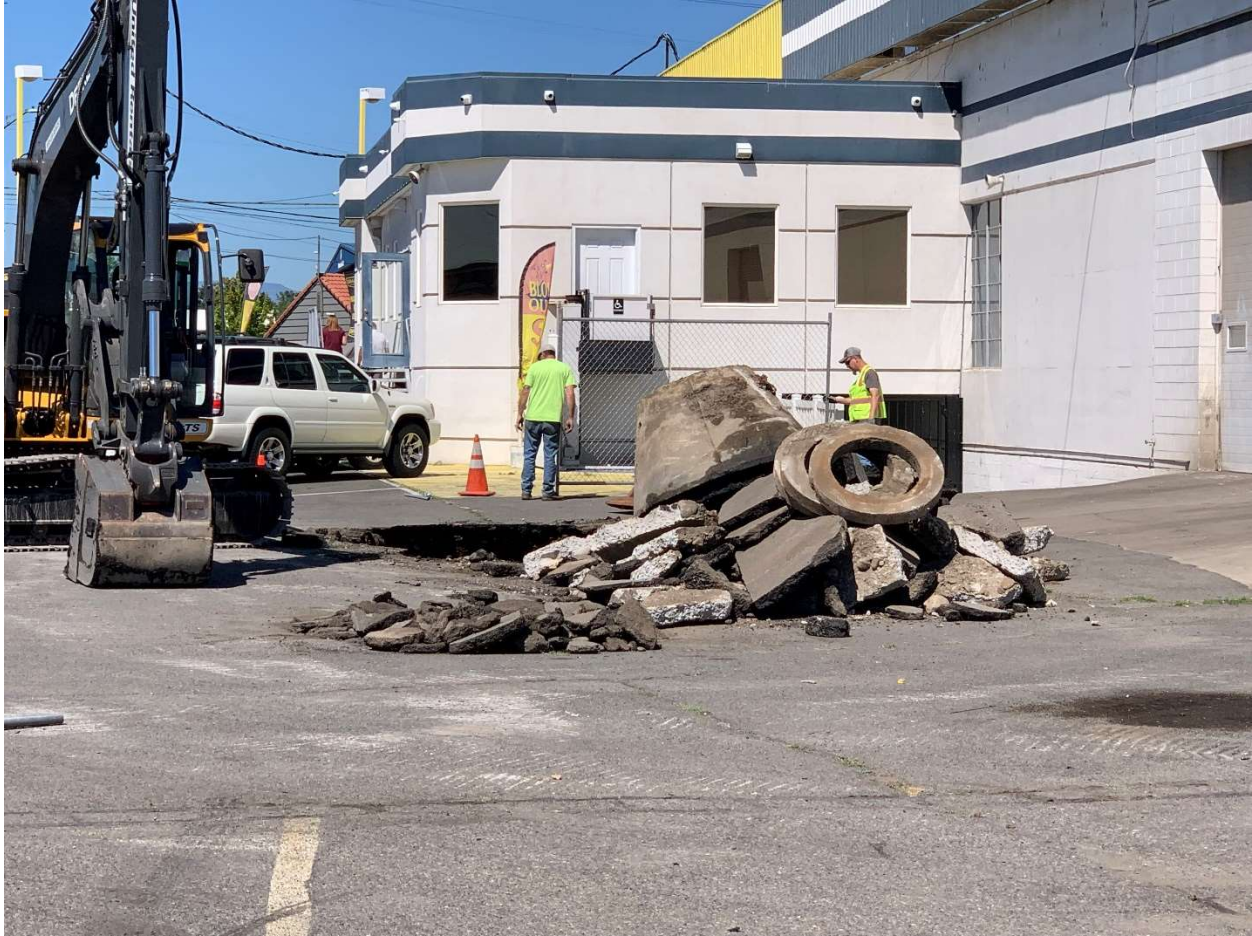
Photograph 14 – Dry Well 1 removed from the ground on July 12, 2022 (facing west).
