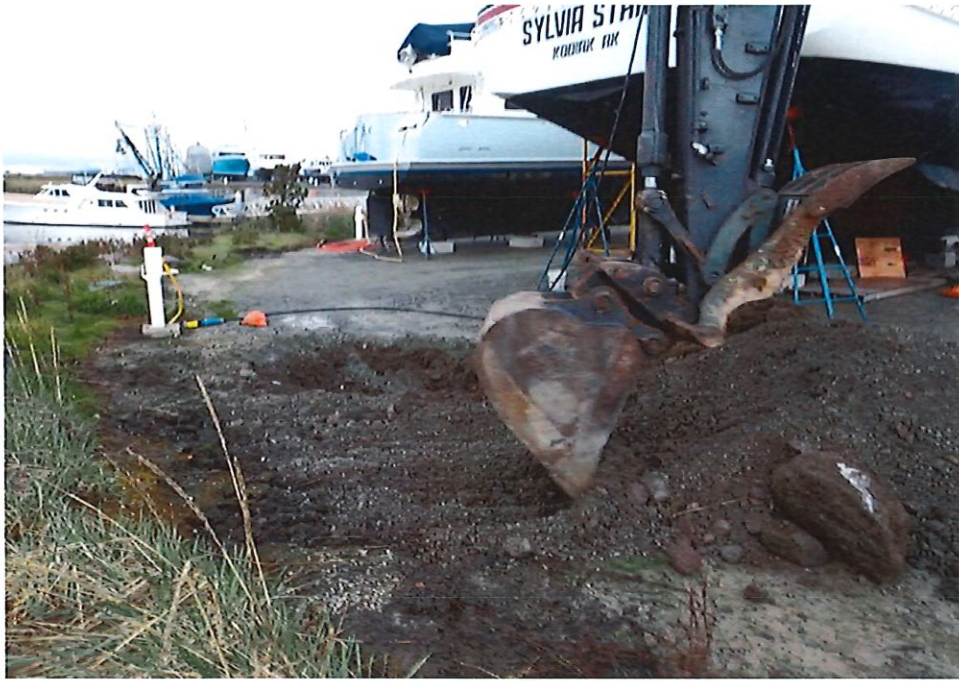
3. Looking south as excavation continues north toward vessel.
