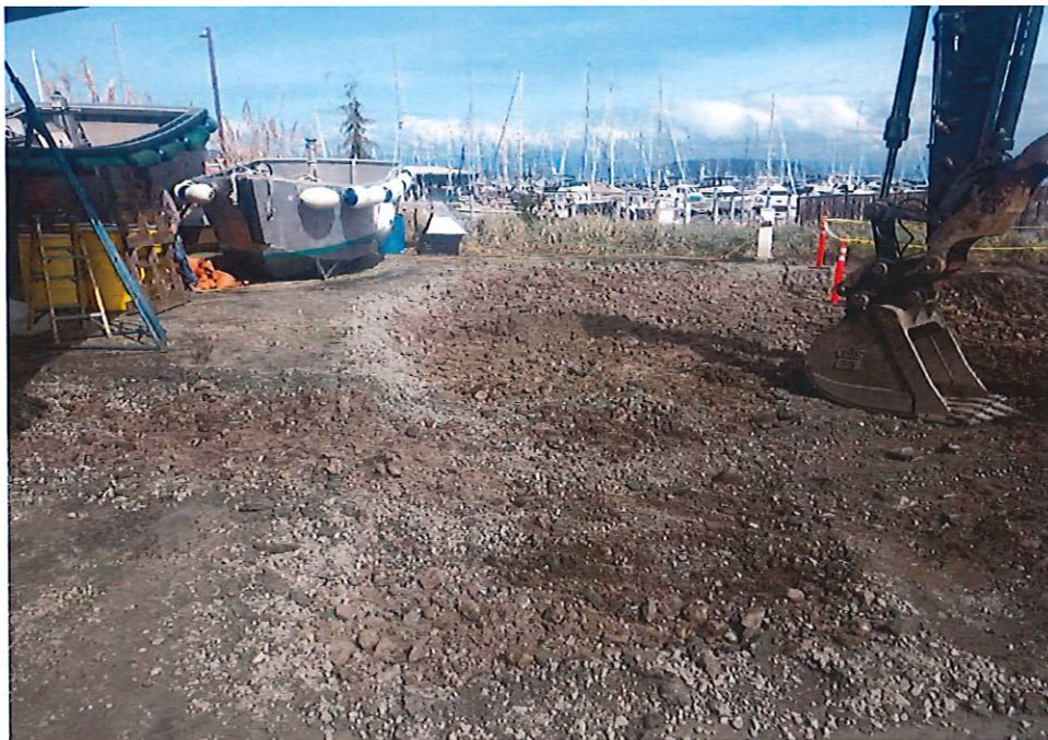
6. Looking east at the final remediation area. Final area measured approximately 61' X 42', in addition to a small 9' X 7' area directly under the spill source.
