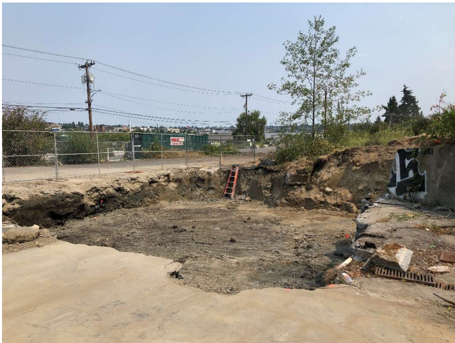
20. CAA-5 excavation complete. View to the northeast. Photograph taken 8/3/2021.
