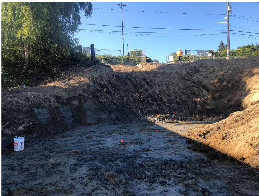
22. CAA-6a floor and south wall PID-screening and sampling (pin flags). View to the south. Photograph taken 7/29/2021.
