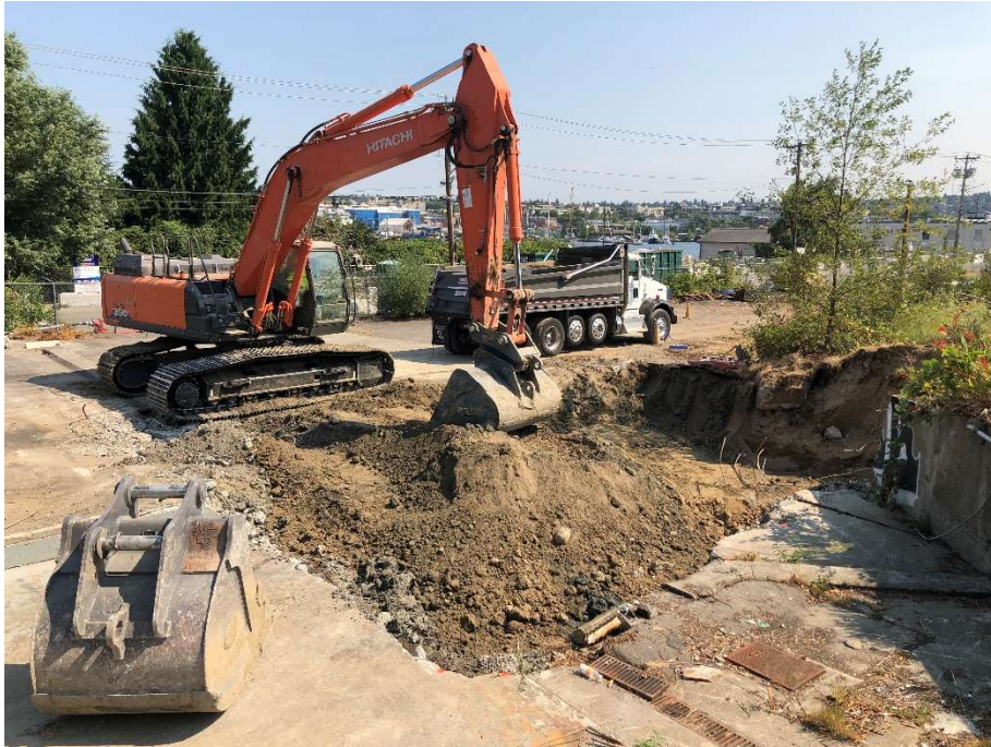
19. Excavating soils at CAA-5. View to the northeast. Photograph taken 8/2/2021.
