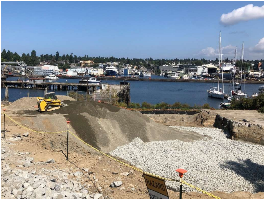
26. CAA-6a. Quarry spall on bottom, adding gravel borrow. View to the north. Photograph taken 8/23/2021.
