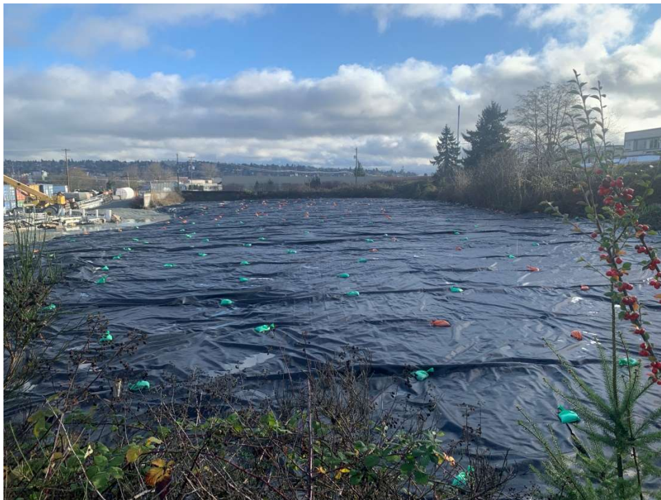
47. Completed SMA Area. View to the east. Photograph taken 12/13/2021.
