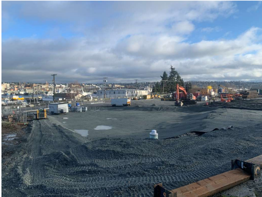
46. Completed CAA-4 surface. View to the south-east. Photograph taken 12/15/2021.
