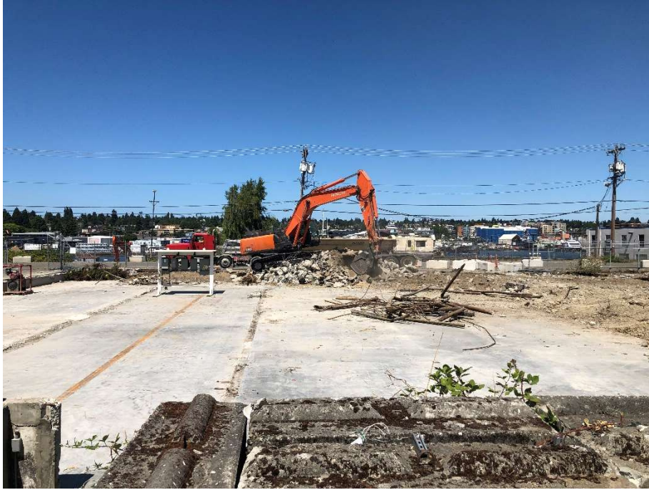
3. Concrete removal at CAA-2 (area preparation). View to the north. Photograph taken 7/29/2021.
