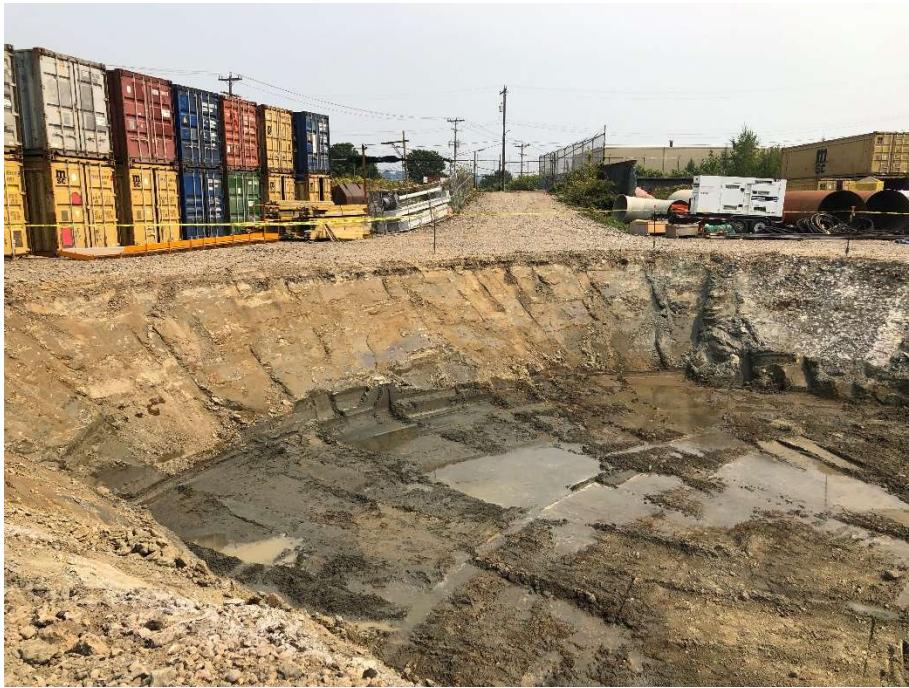
7. CAA-1b excavation. View to the east. Photograph taken 8/13/2021.
