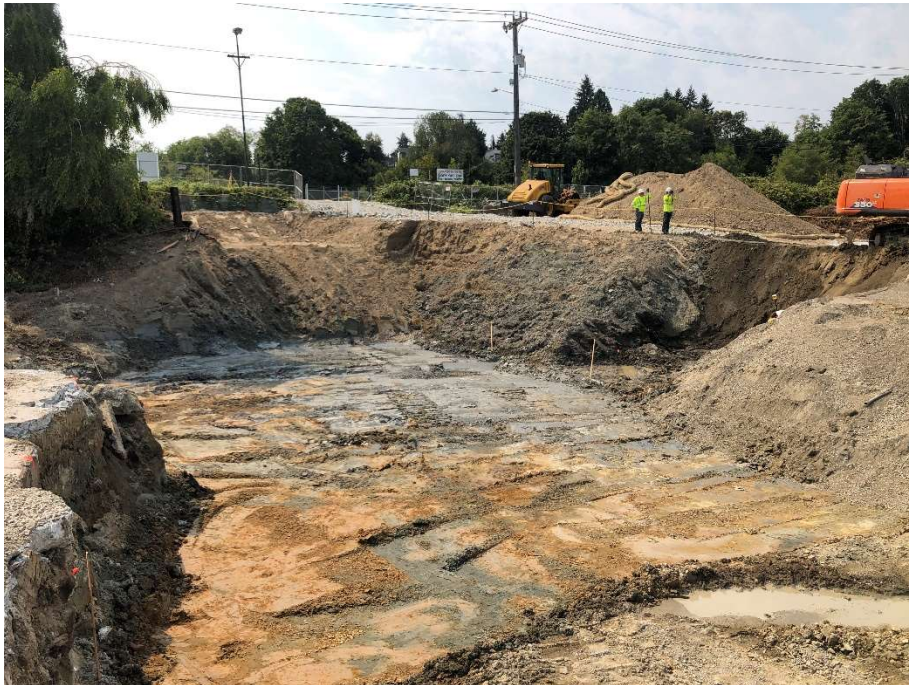
25. CAA-6a excavation underway. View to the south. Photograph taken 8/3/2021.
