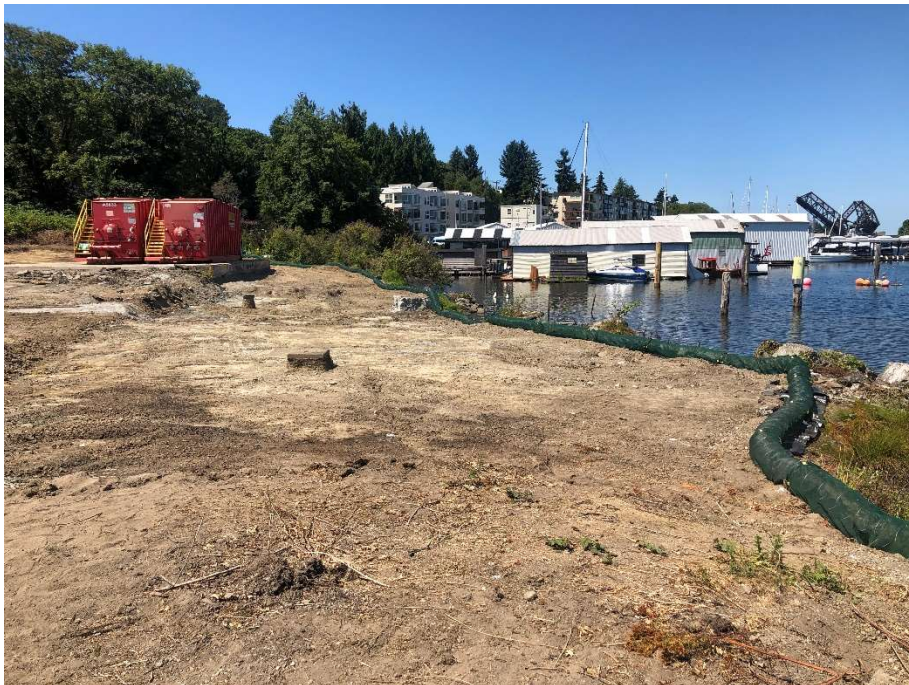
31. CAA-7 post-remedial surfaces. SWPPP BMPs in-place. View to west. Photograph taken 7/23/2021.
