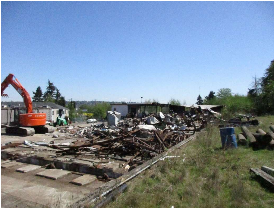
2. Building 2 (Parcel E) demolition underway. View to northeast. Photograph from 4/20/21.
