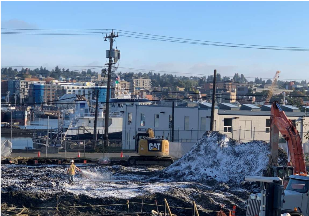
35. CAA-2a odor foam suppressant application (white foam in the photo). View to the south. Photograph taken 9/24/2021.
