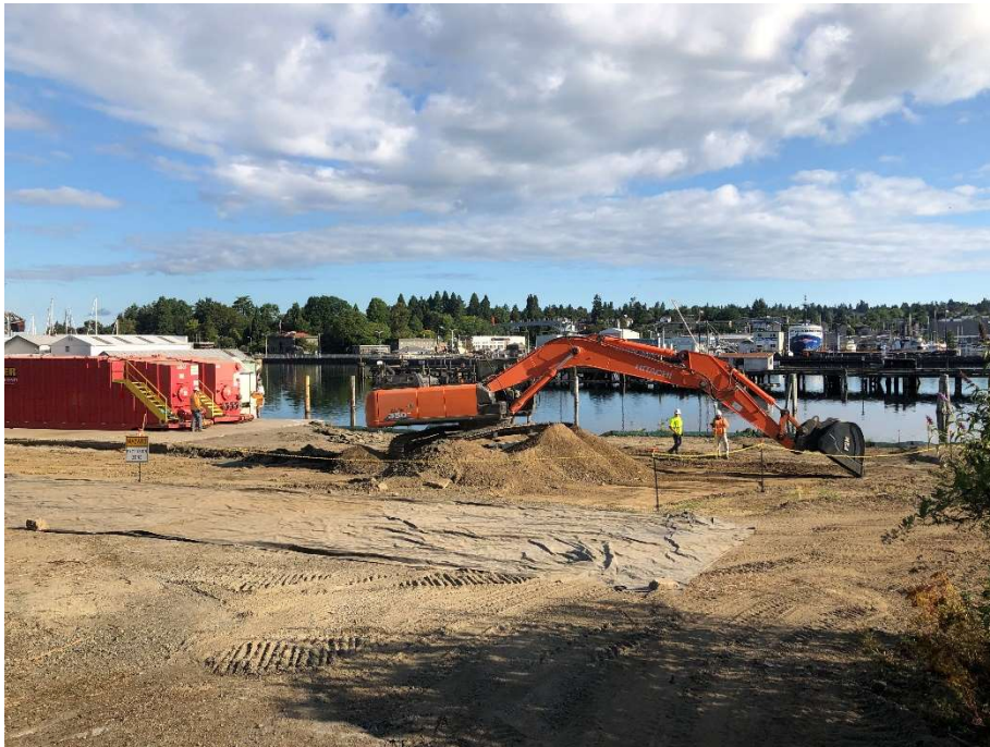
29. Excavating soils at CAA-7. View to the north. Photograph taken 7/22/2021.
