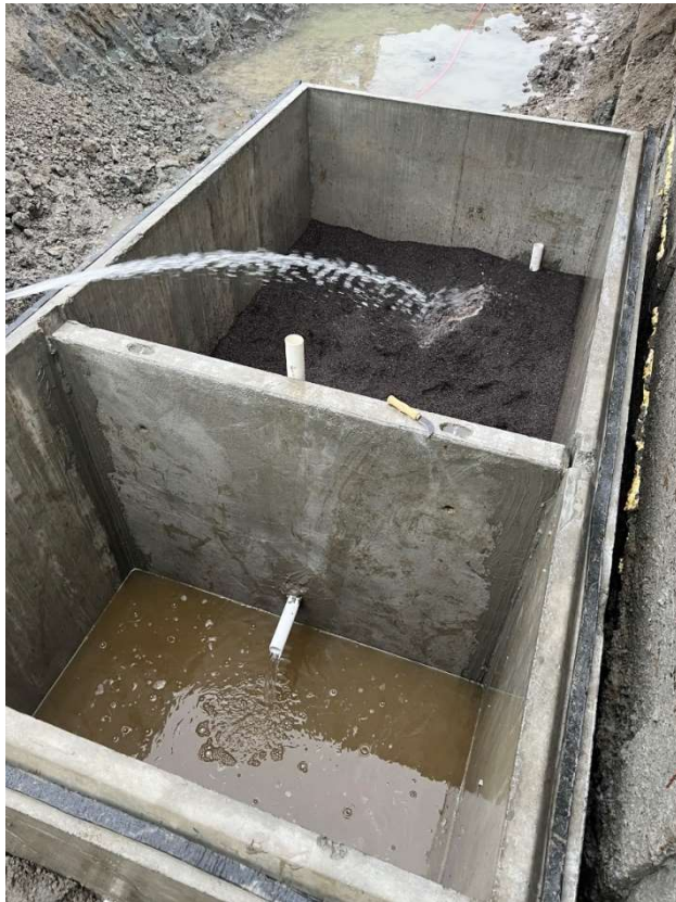
40. CAA-4, saturating gZVI prior to closing concrete vault. Photograph taken 11/11/2021.
