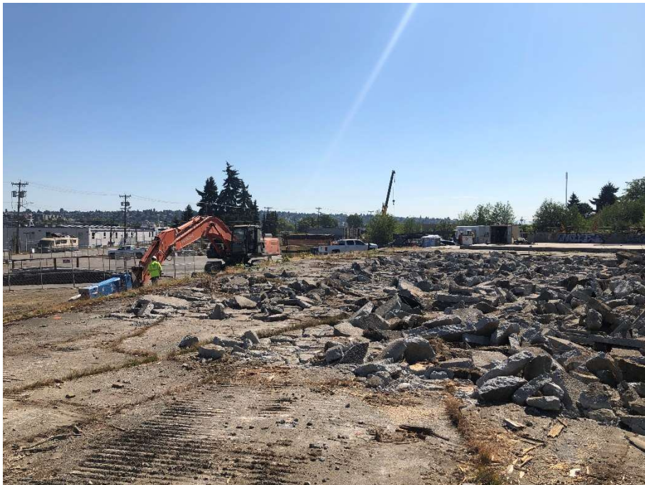
4. Concrete breakup at CAA-4 (former loading dock). View to the east/northeast. Photograph taken 7/29/2021.
