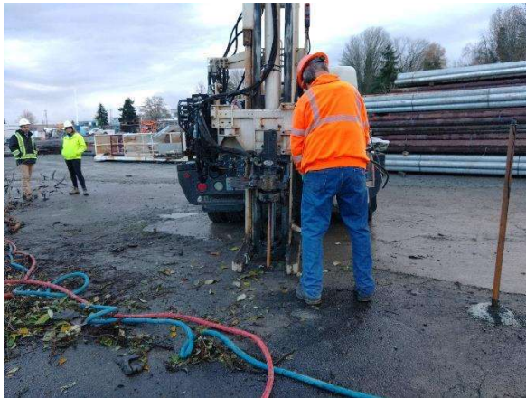
Photo 3: ESN personnel lifting injection rods to specified interval. Southeast view.
