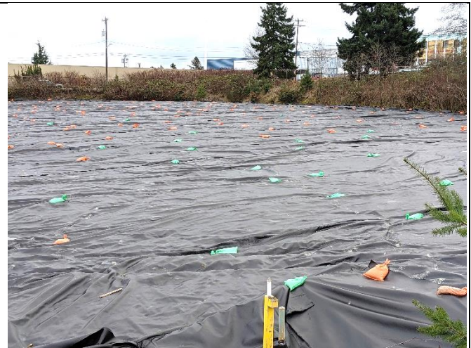
Plate 2: ISS swell management area covered with geotextile.
