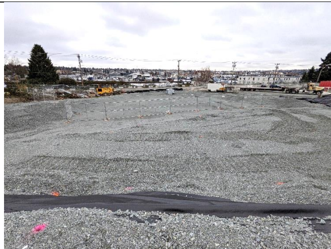
Plate 1: CAA-3 and 4 with permanent erosion control.
