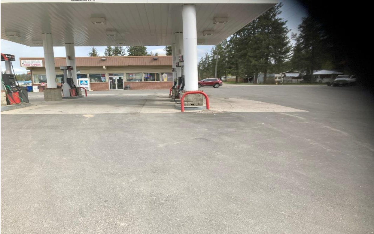
Photo 2: Former Well and Treatment Trench – from the south
