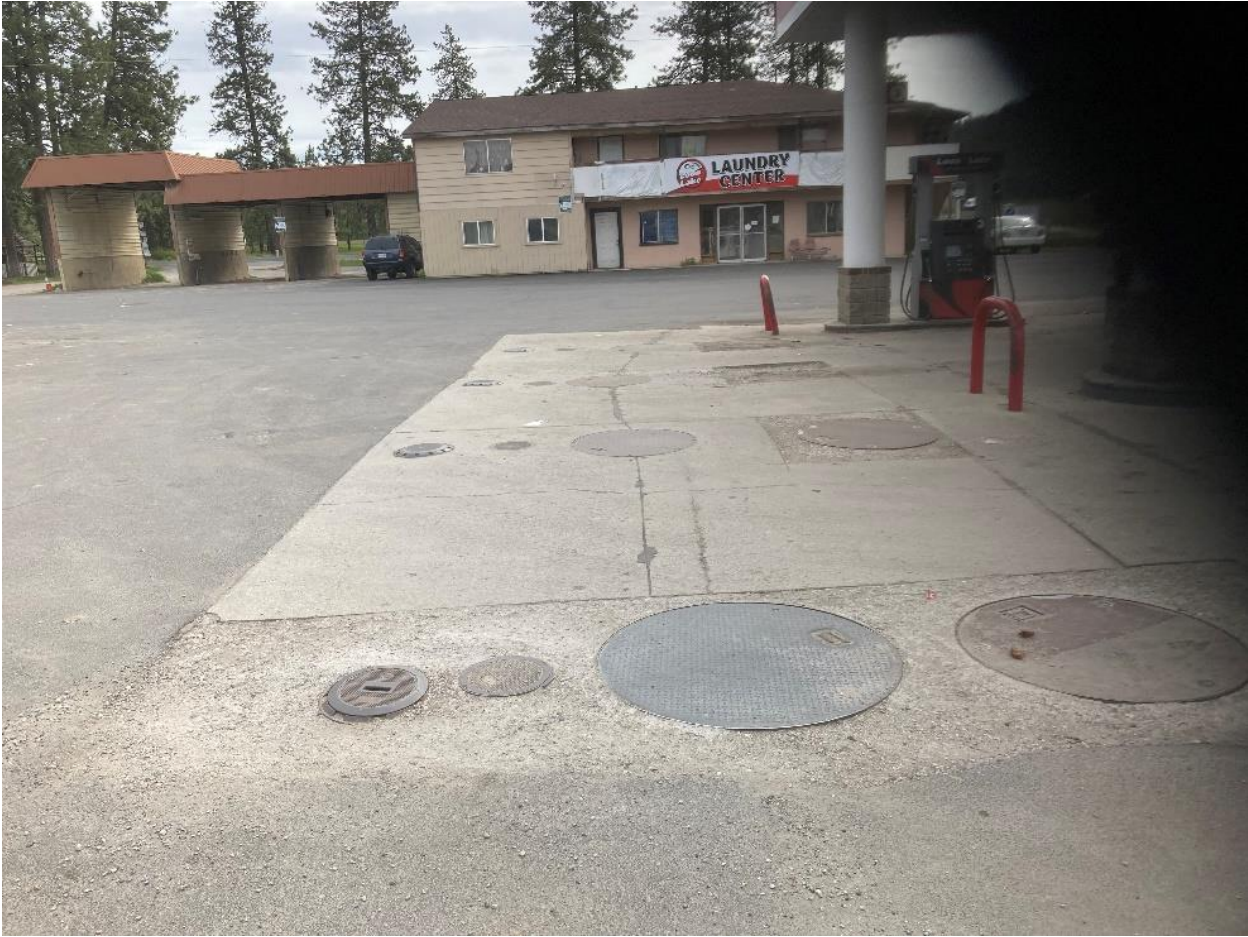
Photo 4: Former Wells and Treatment System Trench – from the south
