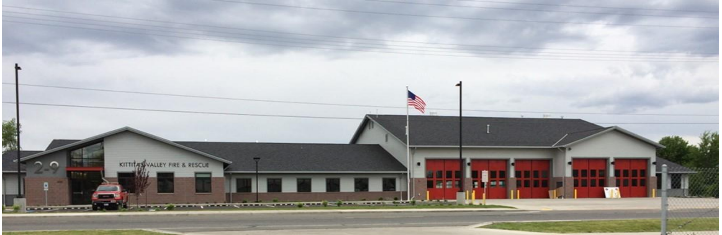
Figure 1. Kittitas Valley Fire & Rescue found an ideal home to serve their community on a brownfield property.
