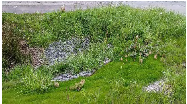
SPPD G-3: New vegetation and rock around culvert
