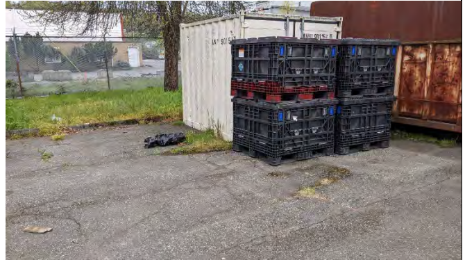
SRDS AC-1: Minor cracking
