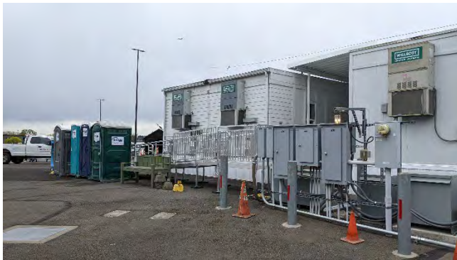
SPPD AC-3: New Buildings, potential cap penetration
