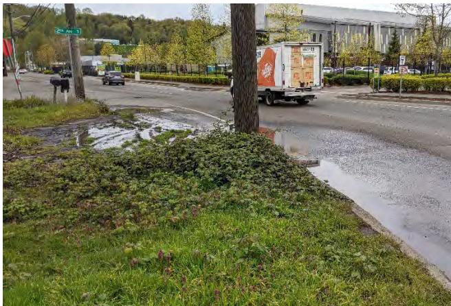
SRDS AC-18: Ponding
