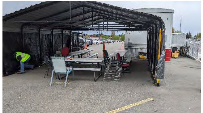
SPPD AC-3: New Buildings, potential cap penetration
