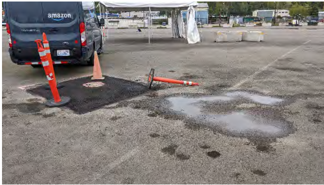
SPPD AC-5: Modification of asphalt
