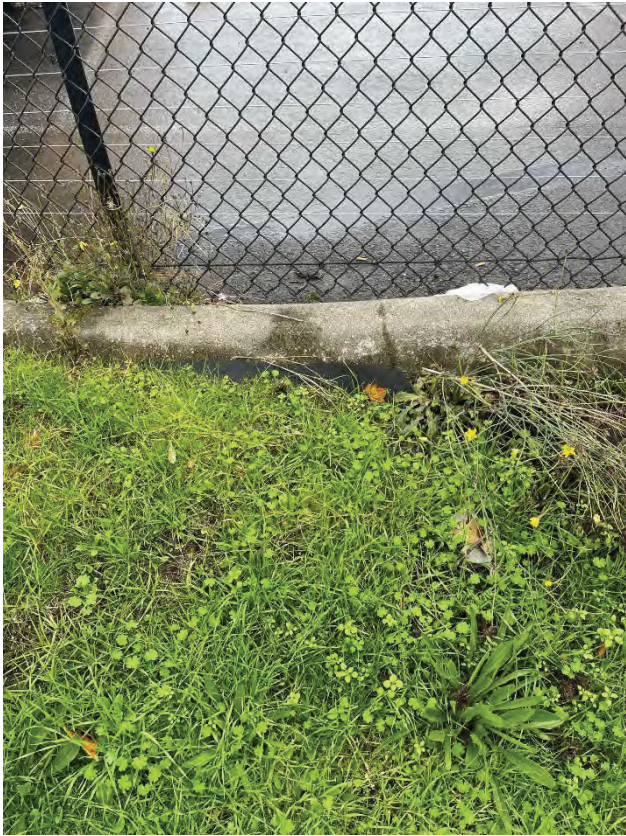
Location 8-1. Exposed Geomembrane
