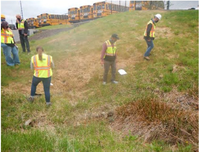
Location 21- 12. Exposed Geomembrane
