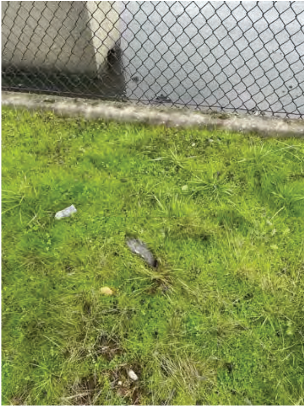
Location 6-1. Exposed Geomembrane
