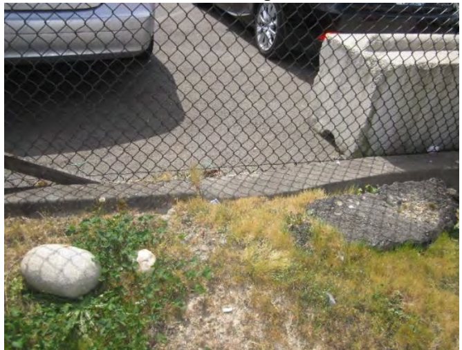
Location 21- 9. Poor Vegetative Cover
