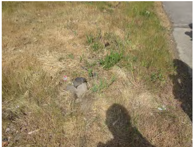
Location 21- 18. Exposed & Damaged Geomembrane
