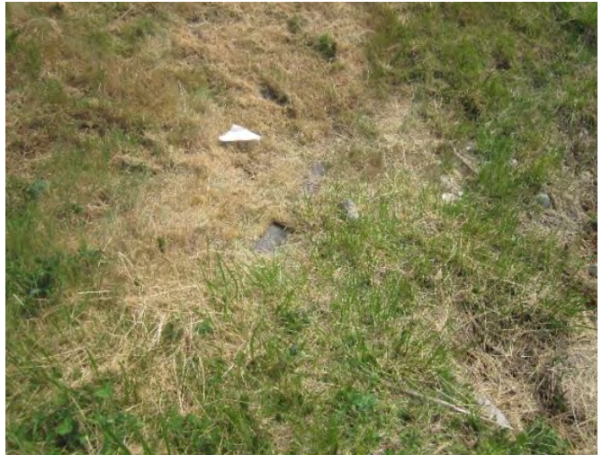
Location 21- 12. Exposed Geomembrane
