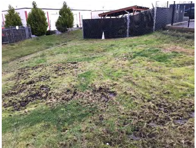
Sparse vegetation as a result of plug aerator
