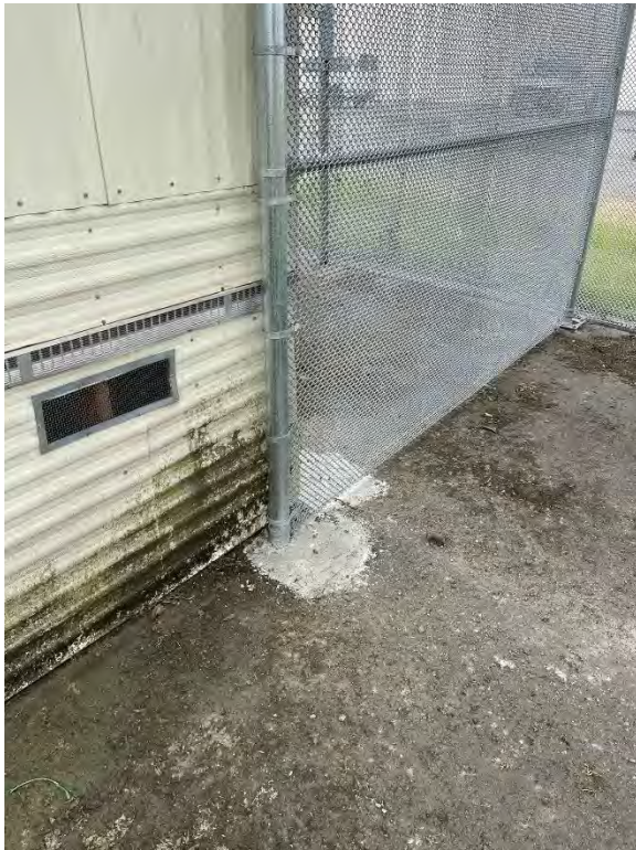
Location 21- 1. Recent Maintenance Activity
