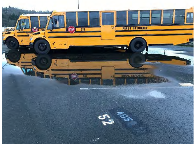
Shallow ponding photographed near 47.5291218, - 122.3298498.
