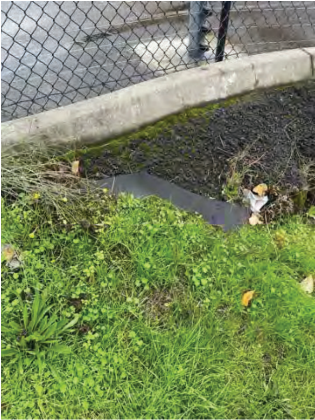
Location 9-1. Exposed Geomembrane
