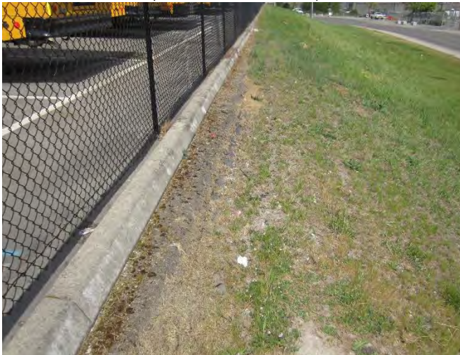
Location 21- 17. Exposed Geomembrane
