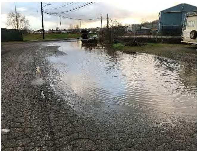
Extensive ponding extending to the north of GP-11 and MW-12. This area is likely ponds after minor rain, too. Photographed facing south.
