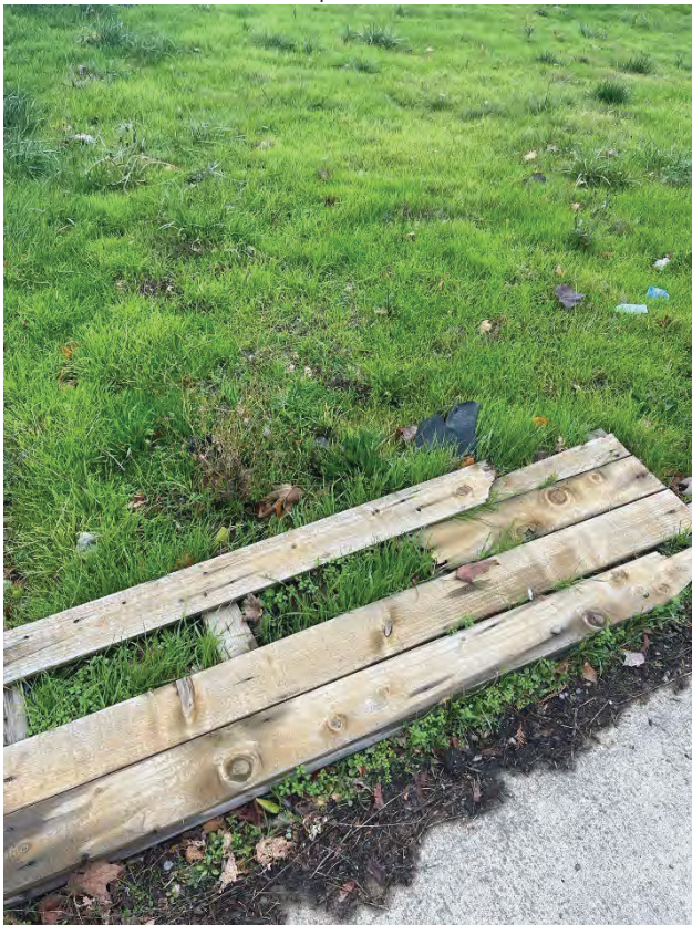
Location 12-1. Exposed Geomembrane
