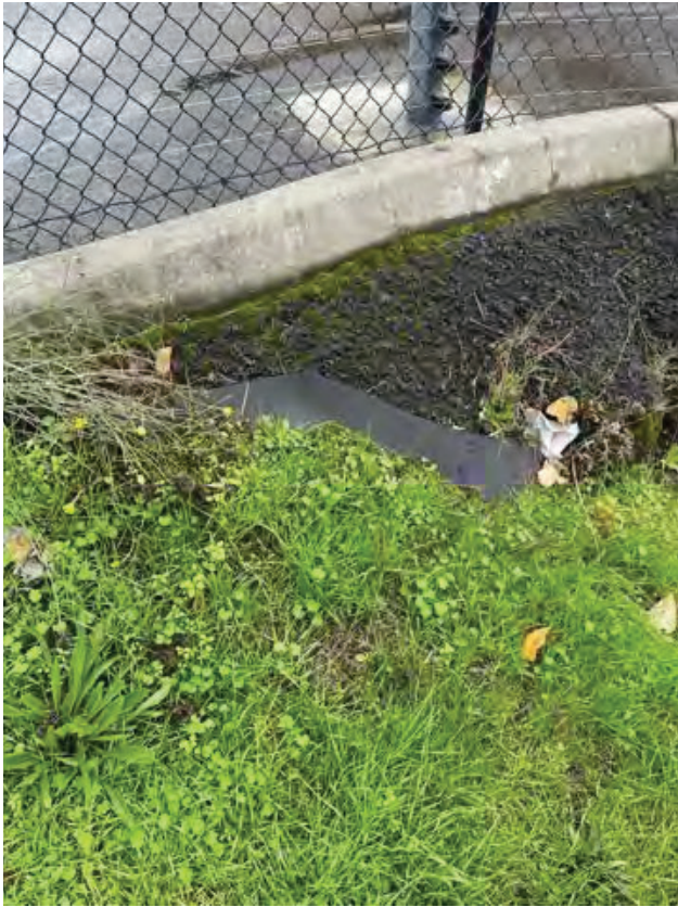
Location 10-1. Exposed Geomembrane
