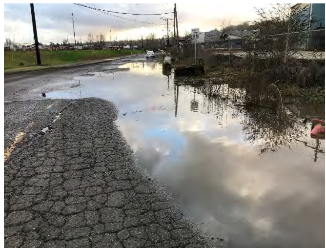
Extensive ponding extending to the north of GP-11 and MW-12. This area is likely ponds after minor rain, too. Photographed facing south.
