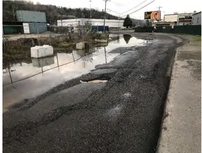
Extensive ponding located near GP-11 and MW-12. This area is likely ponds after minor rain, too. Photographed facing to the north.
