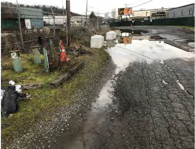
Extensive ponding located near GP-11 and MW-12. This area is likely ponds after minor rain, too. Photographed facing to the north.
