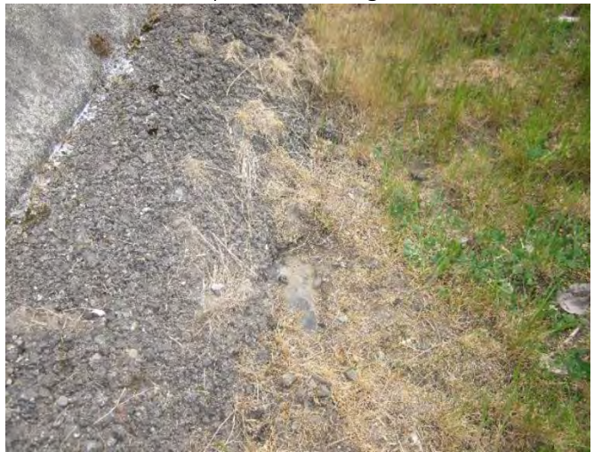
Location 21- 14. Exposed Geomembrane
