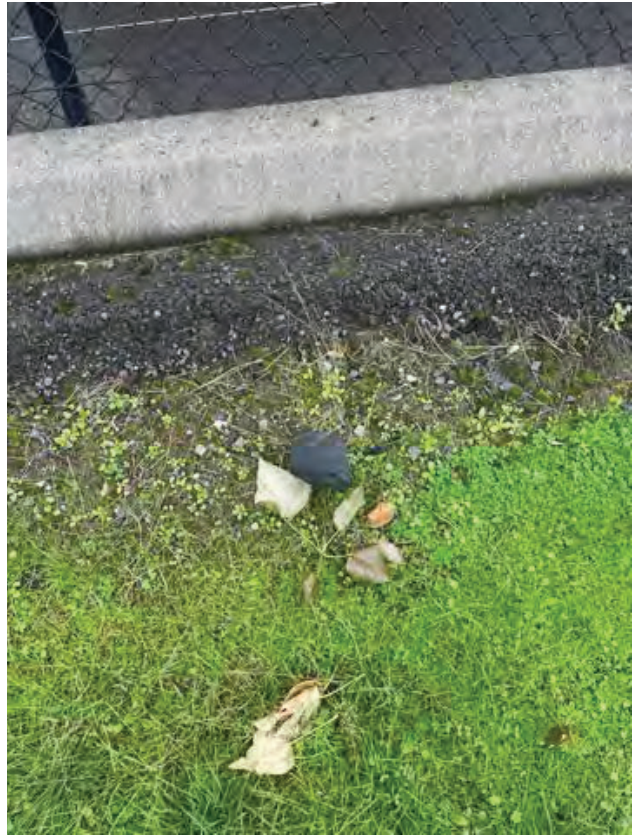
Location 11-1. Exposed Geomembrane
