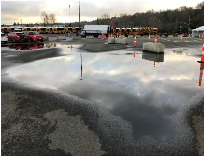
Shallow ponding photographed near 47.5292943, - 122.3321924.
