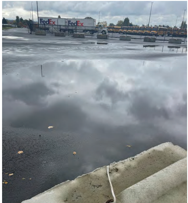
Location 4-1. Pooling/Ponding on Asphalt Concrete View looking South-West from SPPD towards bus lot
