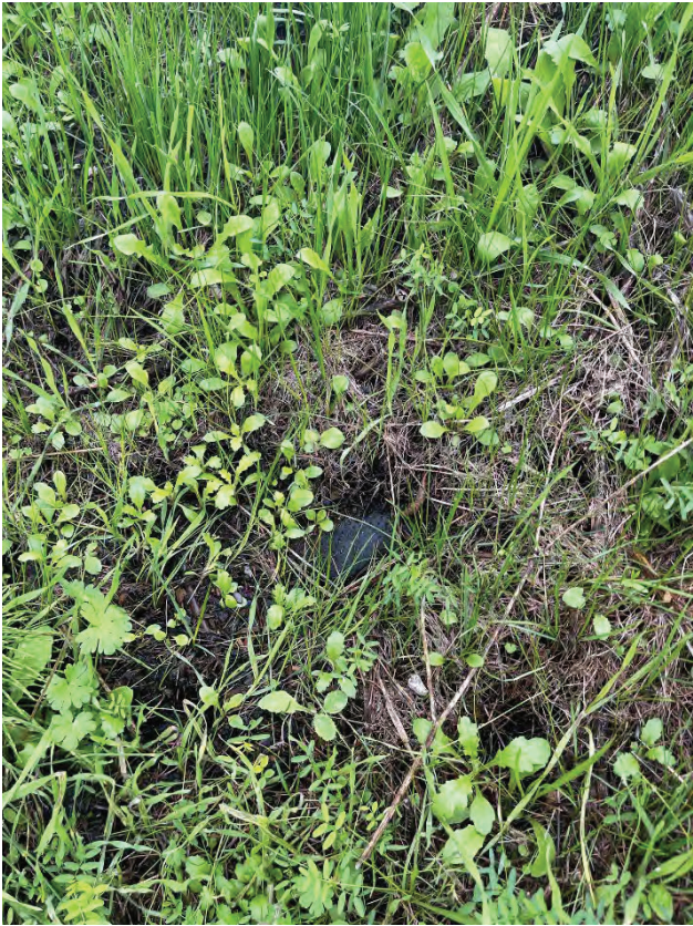
Location 7-1. Exposed Geomembrane
