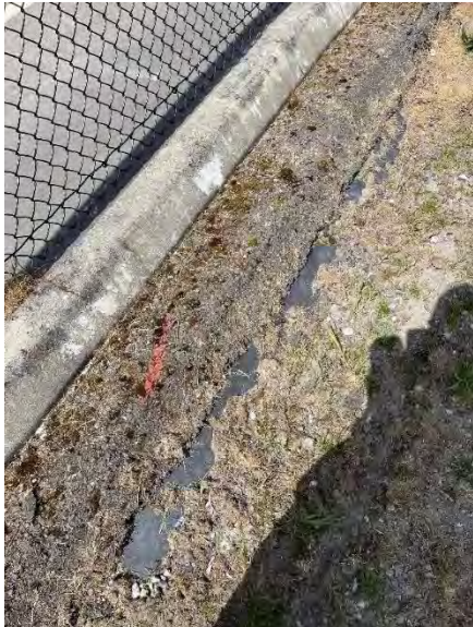
Location 21- 14. Exposed Geomembrane
