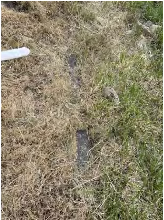
Location 21- 12. Exposed Geomembrane
