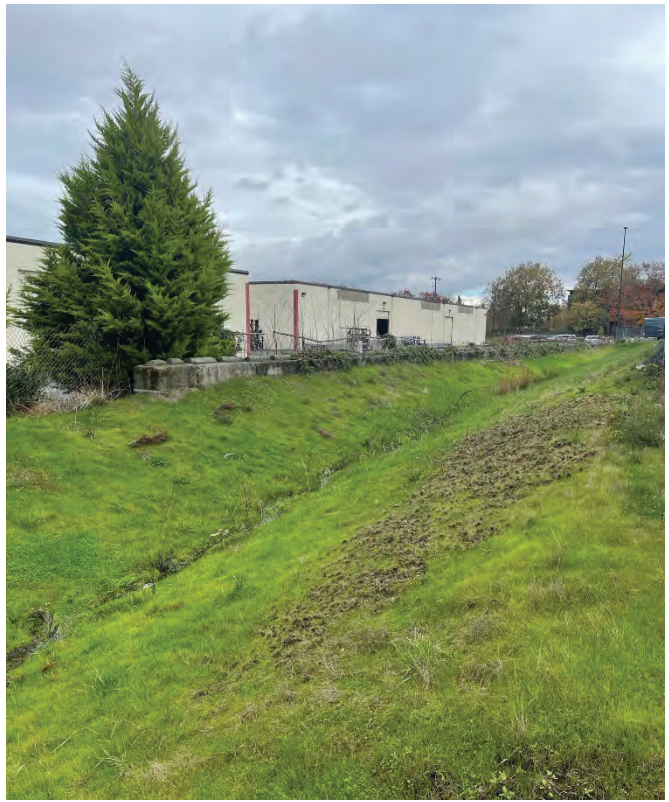
Location 5-1. Poor vegetative cover View looking North-East in vicinity of North swale
