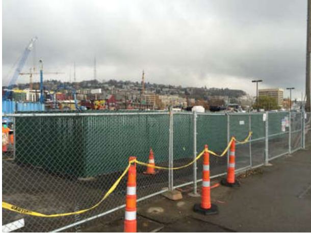
Photo 107 11-14-13: Remediation system compound is installed.
