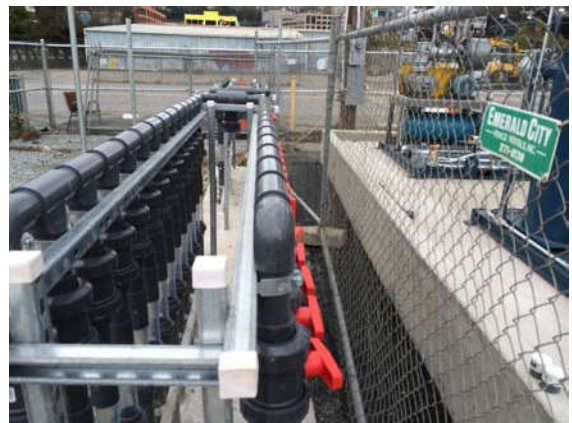
Photo 106 11-13-13: PVC SVE manifold is installed and connected to existing well-piping.
