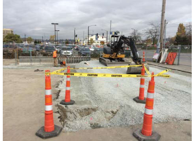
Photo 90 10-30-13: View of sump in southwest corner of foundation, facing north.
