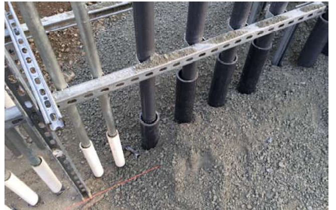
Photo 88 10-30-13: PVC protective sleeves around stub-up piping are secured in gravel foundation.
