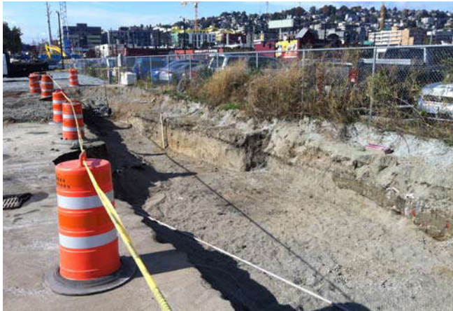
Photo 71 10-10-13: Manifold area trench is excavated.
