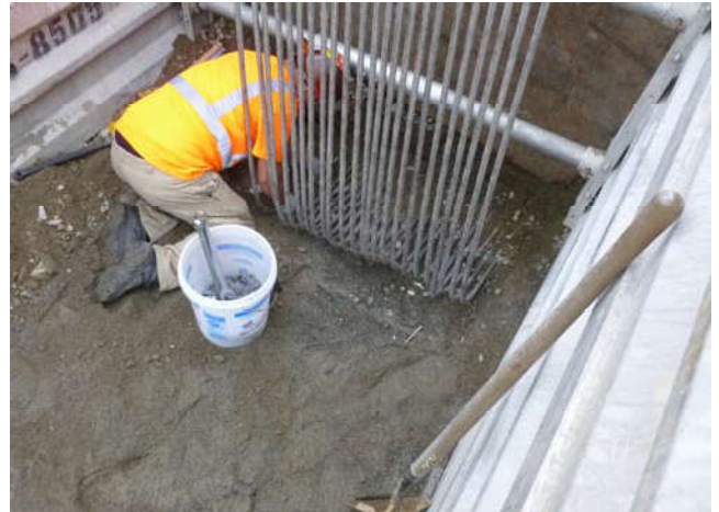
Photo 22 9-9-13: Disconnecting stub-ups from 1" stainless AS well-piping from Westlake Avenue.
