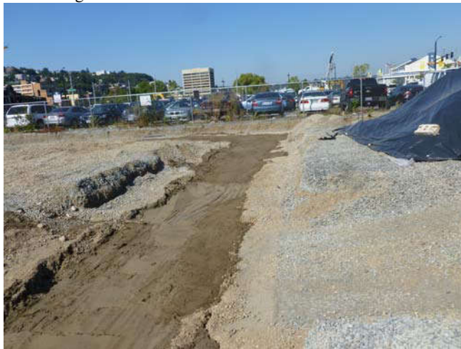
Photo 39 9-12-13: Trench north-adjacent to Mercer Vault after CDF, view facing north.
