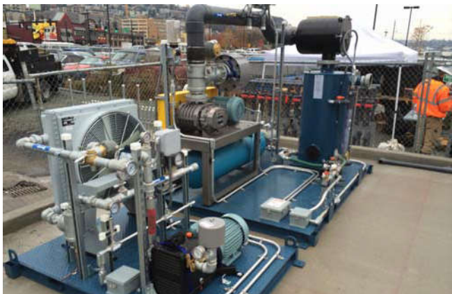
Photo 105 11-12-13: Equipment is placed on pad in accordance with Cardno ERI instruction.
