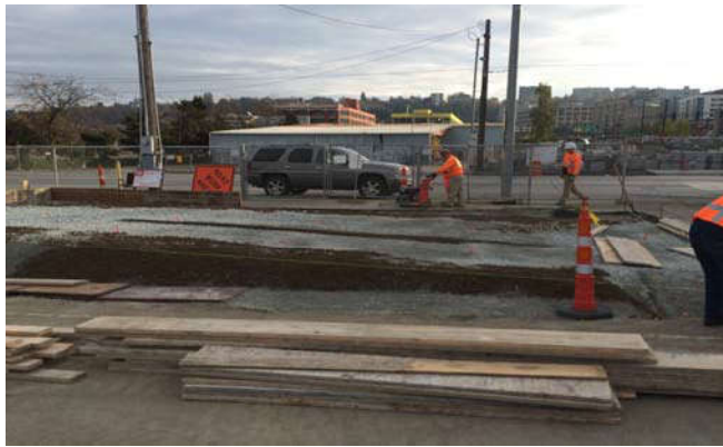
Photo 91 11-1-13: Construction of wood framing for concrete equipment pad form.
