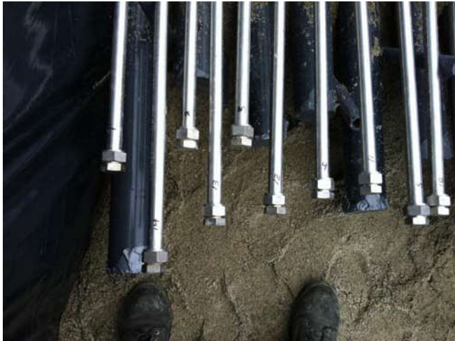
Photo 59 9-27-13: AS piping labeled during connection process after pressure testing.
