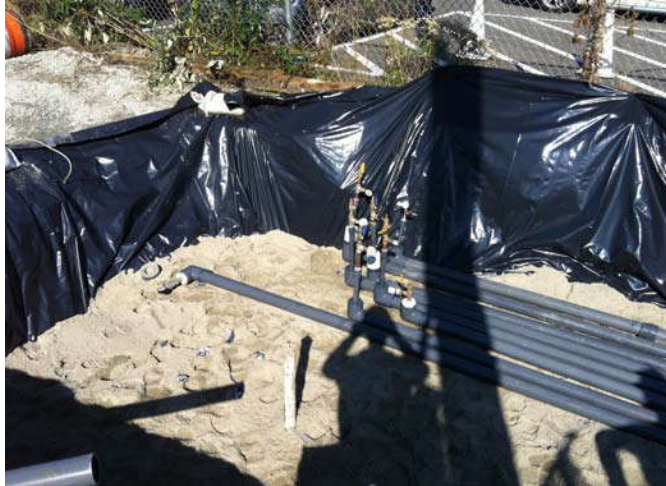
Photo 67 10-4-13: SVE piping is pressure tested.
