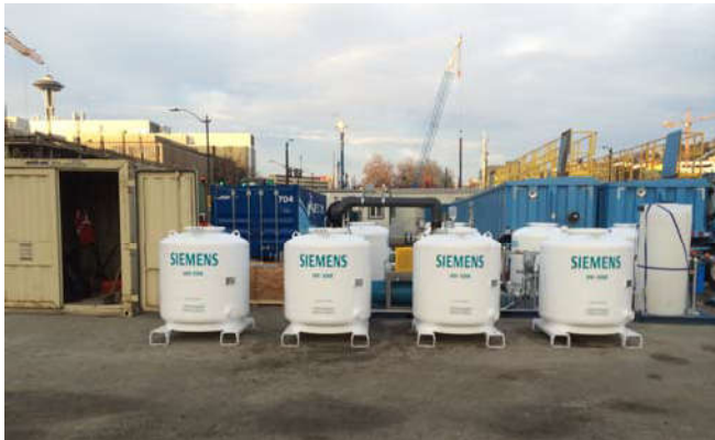
Photo 103 11-11-13: Delivery of remediation system equipment to project site by contractor.
