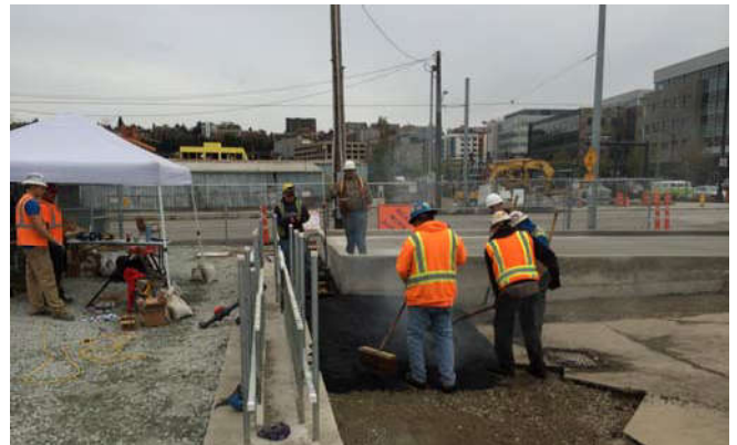
Photo 98 11-6-13: Spreading of asphalt around concrete pad and finished areas.
