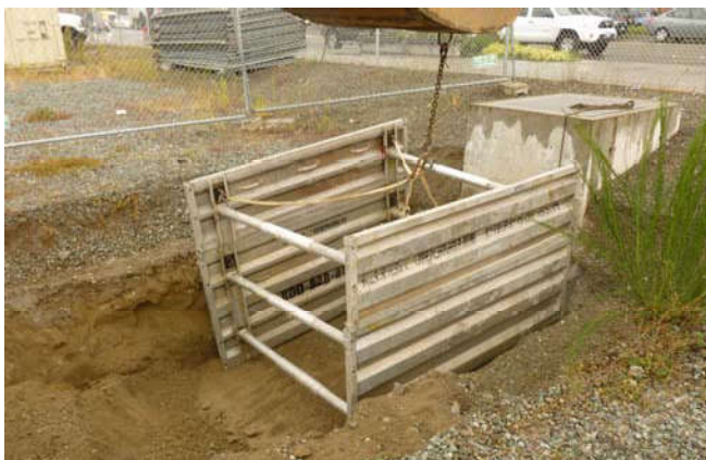
Photo 5 8-29-13: Installing trench box in Mercer Vault trench.
