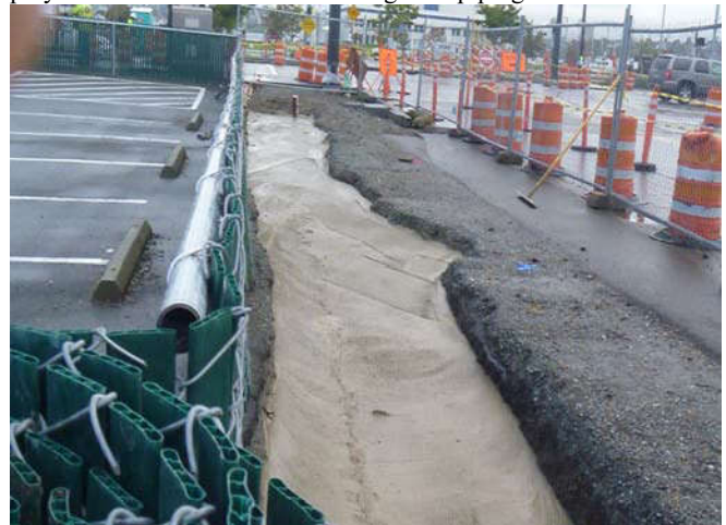
Photo 62 9-30-13: CDF poured over installed well-piping, view facing north on Terry Avenue.
