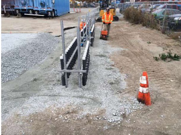
Photo 89 10-30-13: Compacted fill and foundation around stub-up area.
