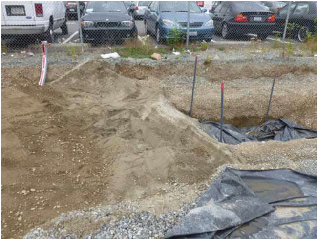
Photo 45 9-17-13: View of temporary termination of well-piping and electrical conduit.
