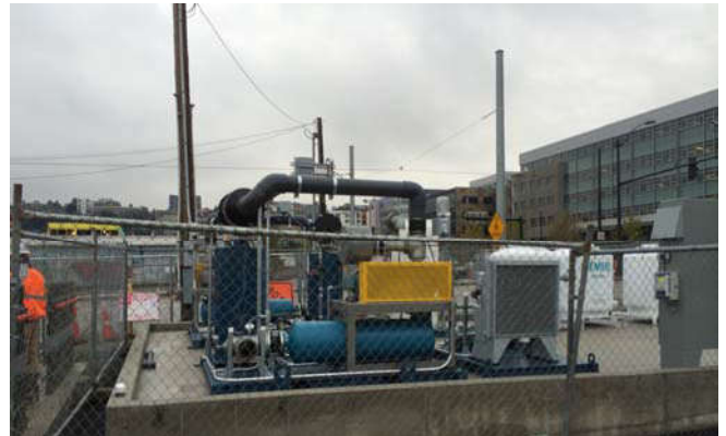
Photo 104 11-12-13: Equipment is transferred onto equipment pad.
