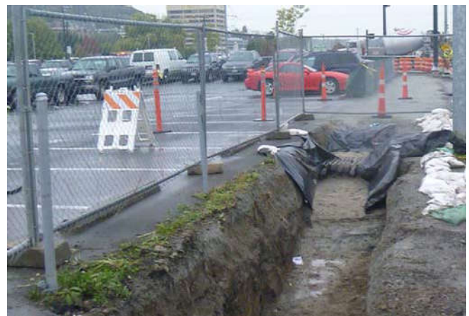
Photo 64 10-2-13: Exposed remediation piping as trench is continued south along Terry Avenue.
