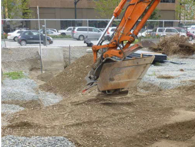
Photo 43 9-17-13: Contractors compacting soil with vibrating plate attachment on excavator.
