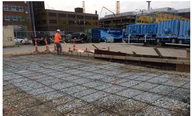
Photo 92 11-4-13: View of concrete form with rebar, preparing for concrete equipment pad.
