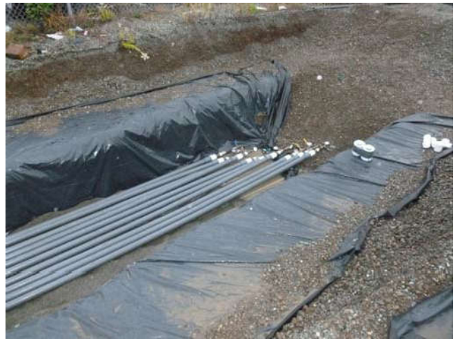
Photo 16 9-6-13: 2" PVC SVE piping from Mercer Vault being pressure tested.
