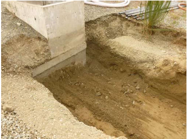
Photo 4 8-28-13: Beginning of trench north-adjacent to Mercer Vault
