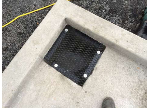
Photo 108 11-15-13: Stormwater sump in southwest corner of concrete pad.
