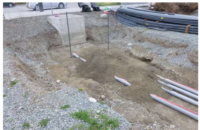
Photo 42 9-17-13: Backfilling activities begin in Mercer Vault trench over installed electrical conduit.
