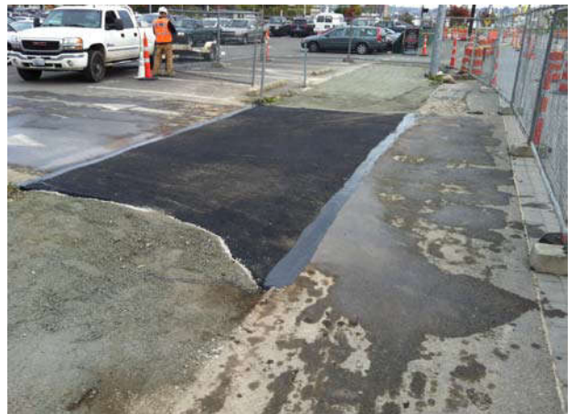
Photo 70 10-10-13: Driveway of parking lot where trenching occurred is restored.
