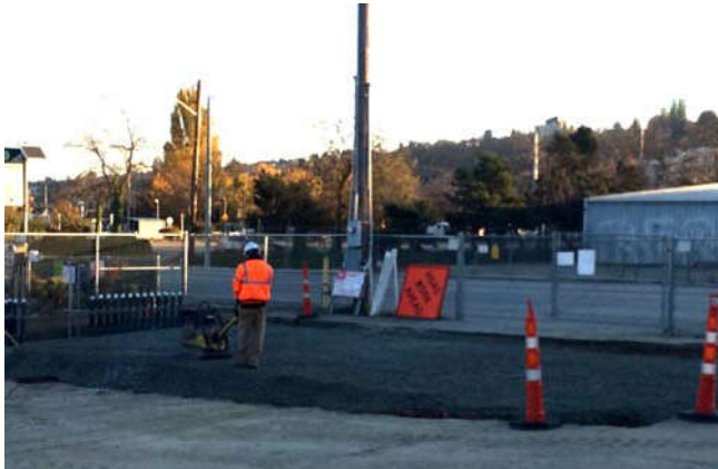
Photo 87 10-29-13: Asphalt foundation for equipment pad compacted with plate-compactor.
