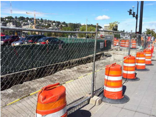
Photo 50 9-24-13: Trenching is continued south along Terry Avenue, view facing northwest.
