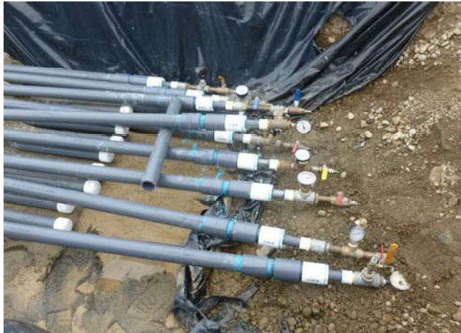
Photo 21 9-9-13: 2" PVC piping for Mercer Vault SVE well-piping being pressure tested.
