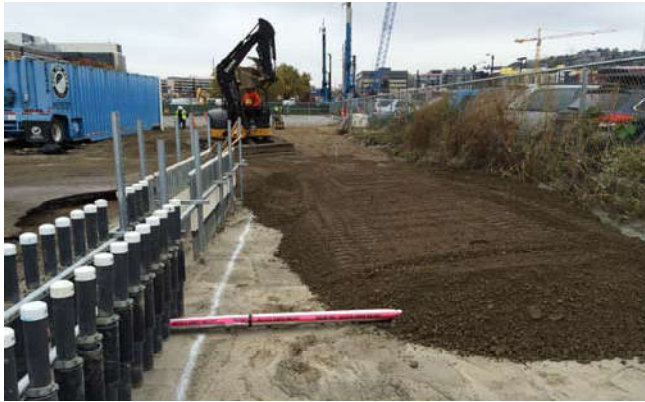
Photo 85 10-25-13: Backfilling of stub-up area.
