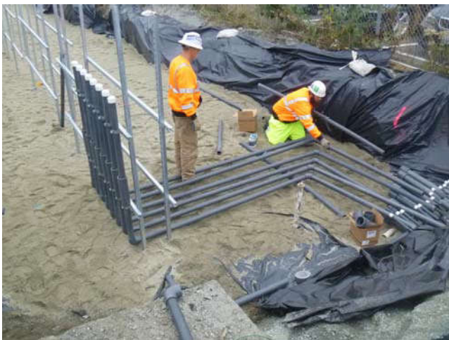
Photo 75 10-17-13: Begin well piping stub-ups from Terry Avenue for manifold connection area.
