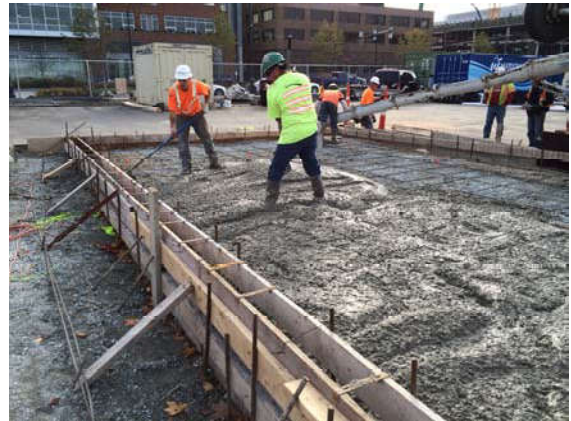
Photo 94 11-4-13: Pouring and spreading concrete into wood frame.
