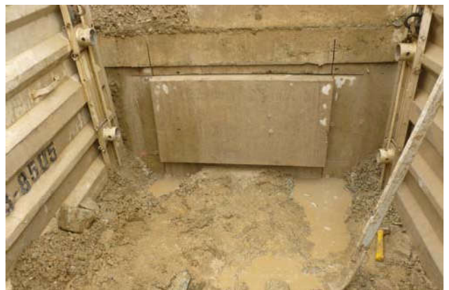
Photo 6 8-29-13: Concrete window cut into north wall of Mercer Vault.
