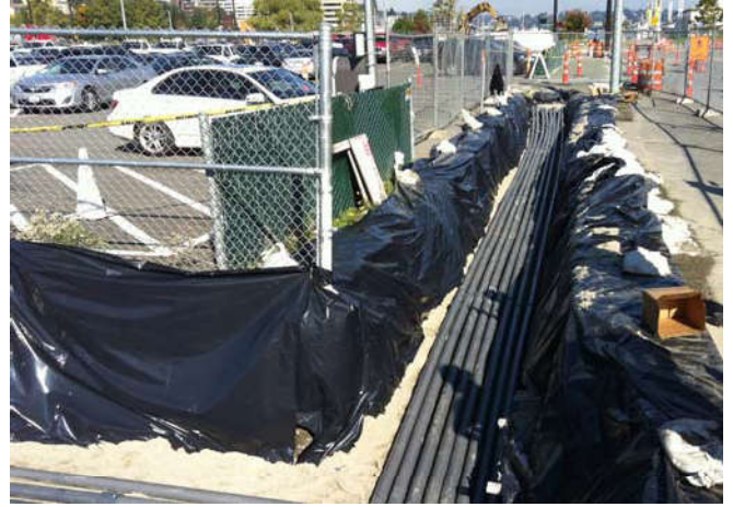
Photo 66 10-4-13: SVE piping is laid in sand-bedded trench leading into project site.
