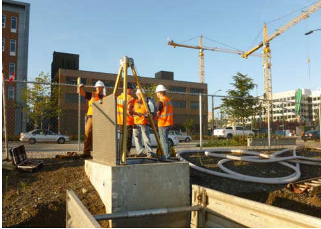
Photo 7 8-29-13: Preparing for confined space entry into Mercer Vault.
