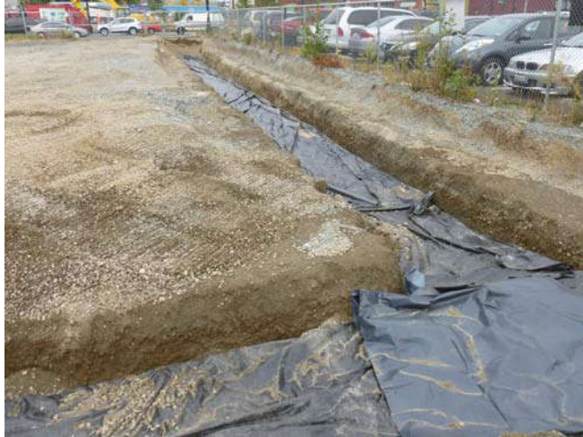
Photo 37 9-12-13: Well-piping and sand backfill is wrapped in poly-liner, view facing northwest.
