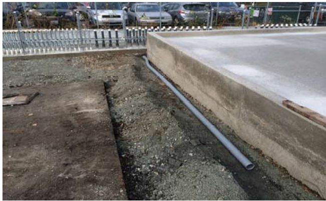
Photo 97 11-5-13: Electrical conduit extended along west side of concrete equipment pad.
