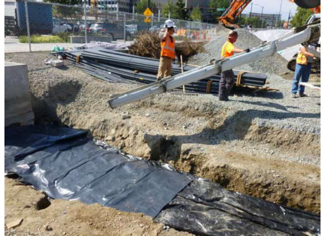
Photo 38 9-12-13: Preparing to pour CDF over wrapped well-piping adjacent to Mercer Vault.
