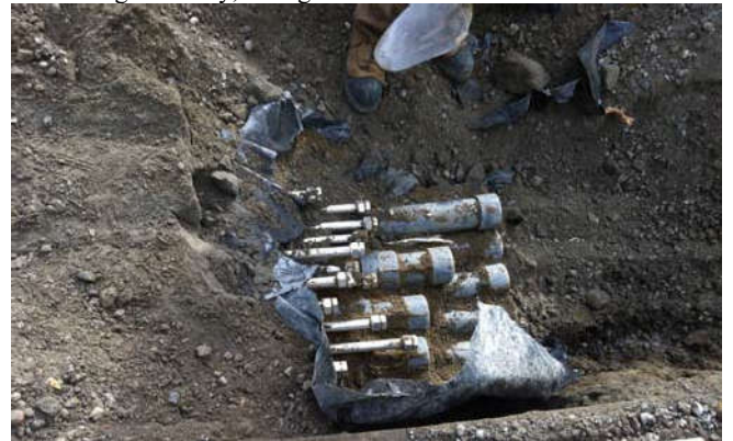
Photo 49 9-24-13: Existing AS and SVE well-piping is un-earthed at the north end of Terry Avenue and labeled according to Cardno ATC documentation.
