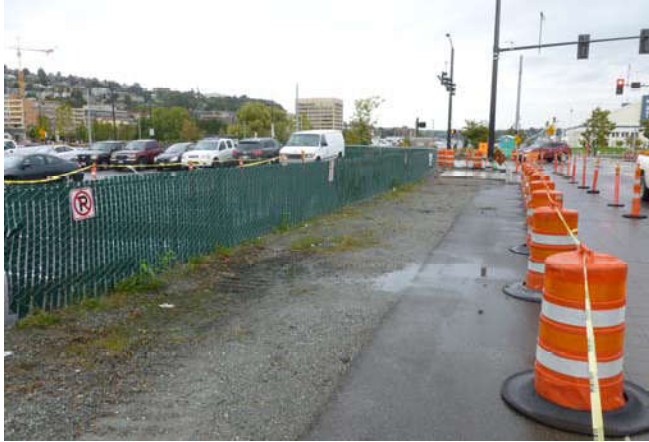
Photo 46 9-23-13: View of Terry Avenue right-of-way before beginning trenching activities, facing north.
