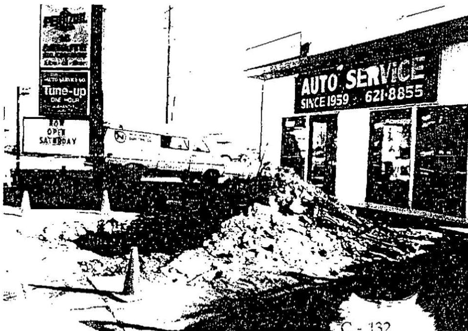
Plate 16. Exploratory hole adjacent to Westlake Avenue. Discovered an abandoned fuel line, but no tank
