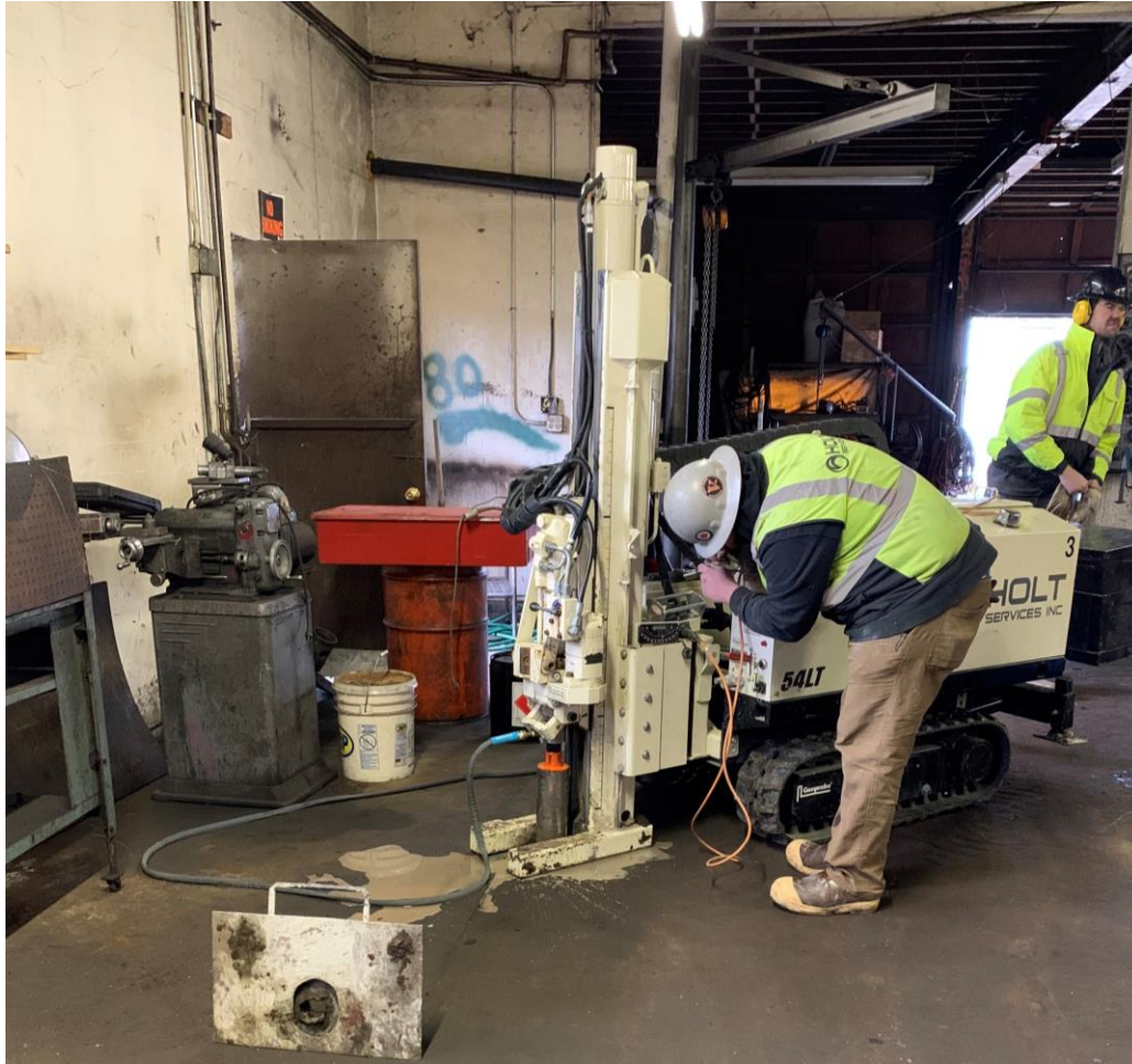
Photo 7: Positioned facing south inside the garage. Drilling of boring B-4.
