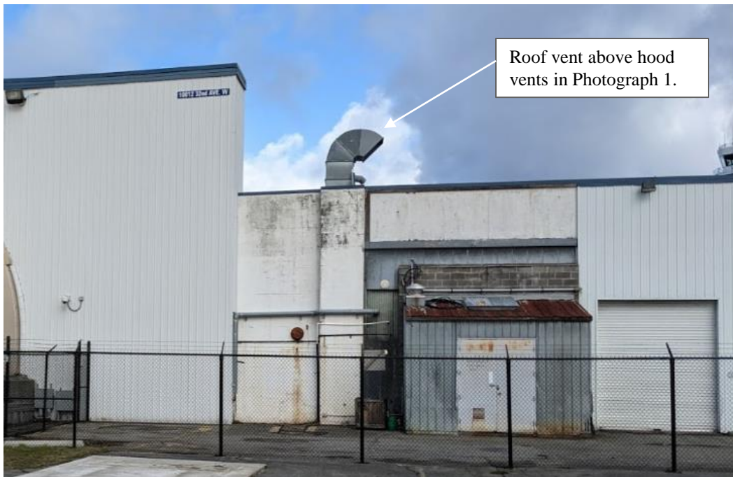
Photograph 2. C-1 Building roof vents above the equipment workshop area. Small metal shed attached to building also pictured.
