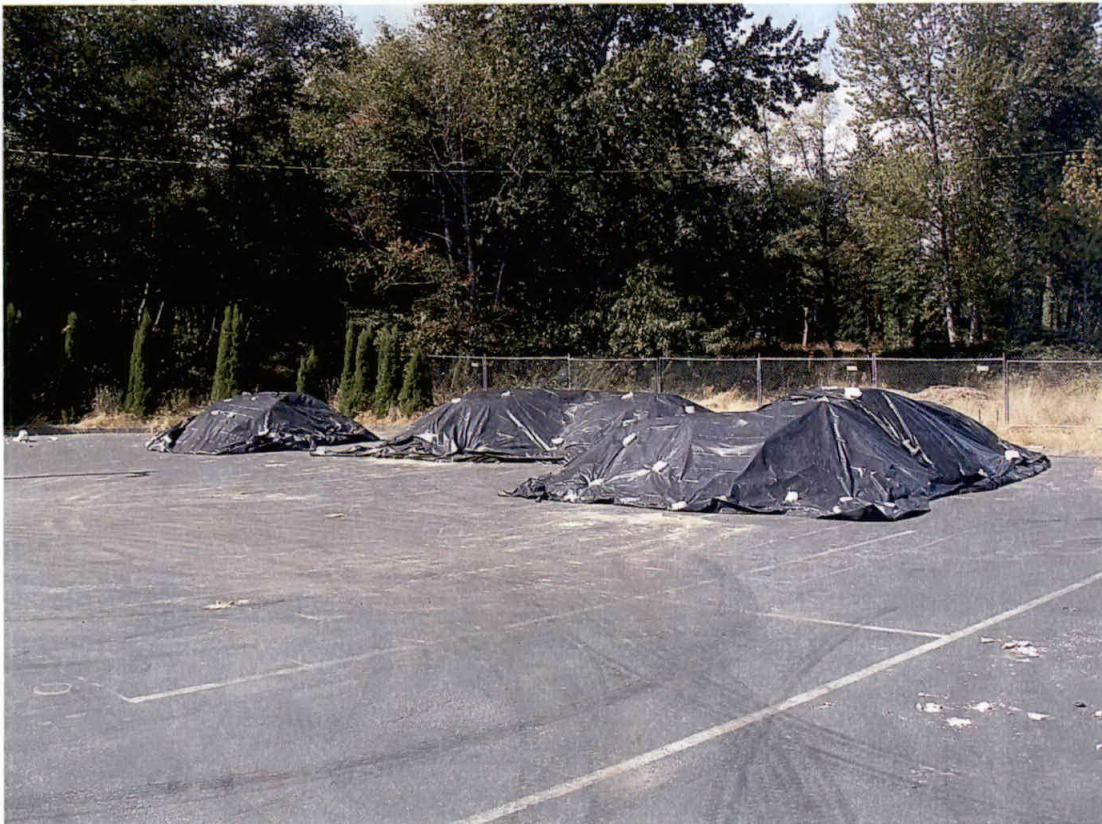
Photo 8. View looking northwest showing the four covered soil stockpiles pending transportation and offsite disposal.
