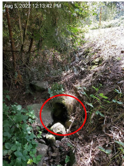
B. Terminal outfall (red circle) for King County MS4, drains to private residences
