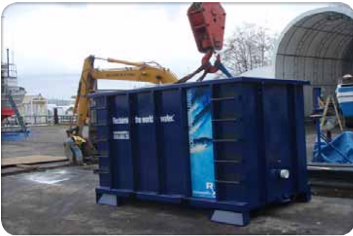
Installation of an Aquip 50 system
