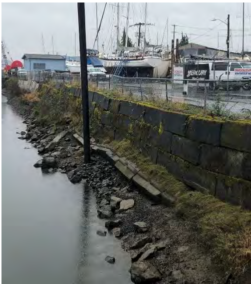
Photograph 1. Ecology block wall along SPM riverbank, looking south.
