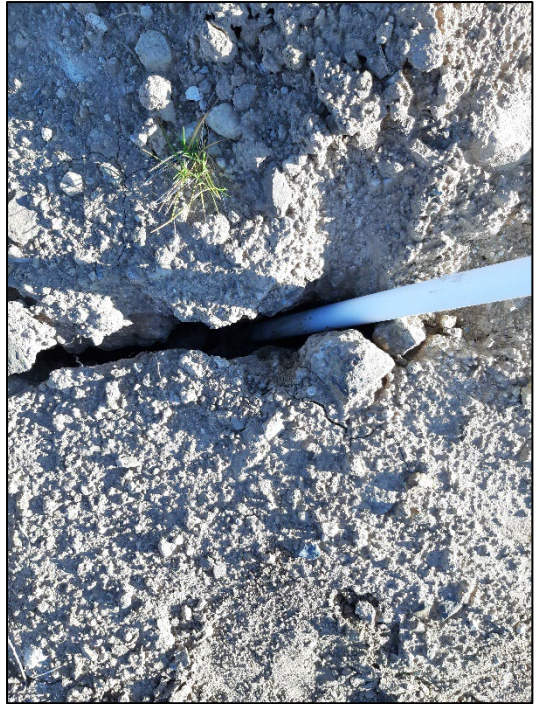
Photo 2: View of sampling down the vent at location A-1. December 8, 2021
