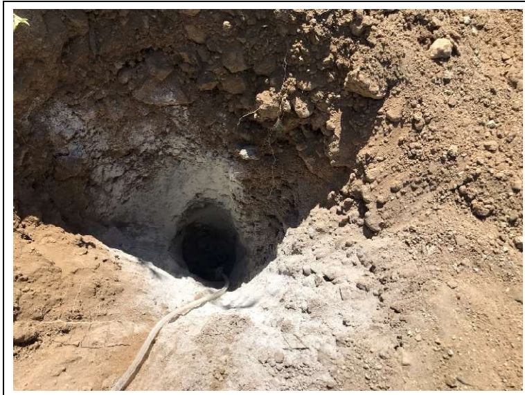
Placing bentonite seal onto the temporary vapor probe
