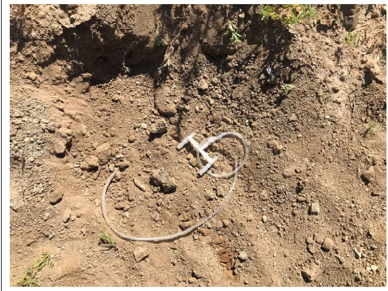
Vapor probe after placing cover back over the top.
