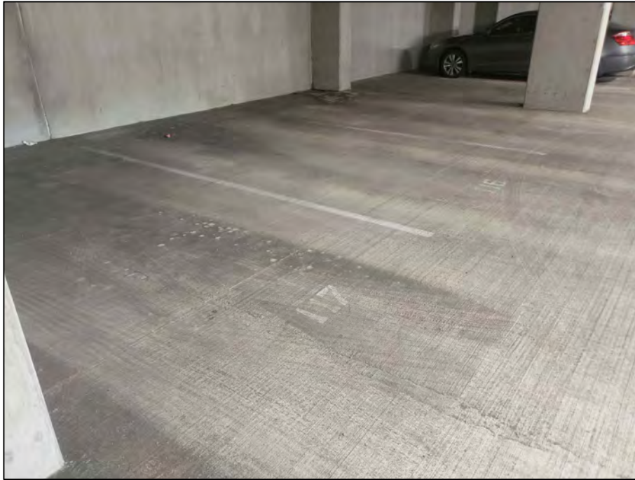
Photograph 1: View looking northwest at the garage floor slab overlying Area 1.
