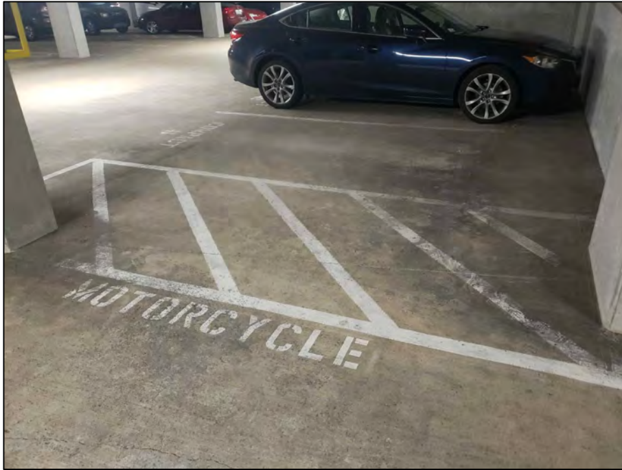
Photograph 3: View looking east at the garage floor slab overlying Area 2.
