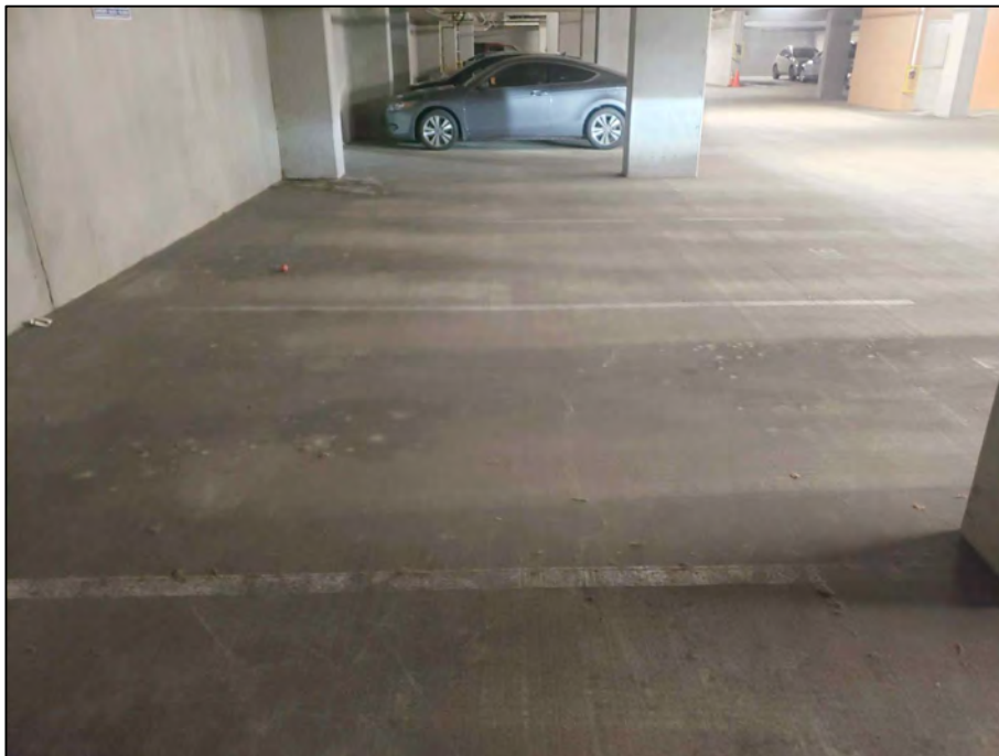
Photograph 2: View looking north at the garage floor slab overlying Area 1.
