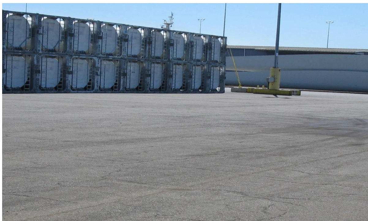
Photo 6. Former plant area and engineered asphalt cap/current storage area—from the East.
