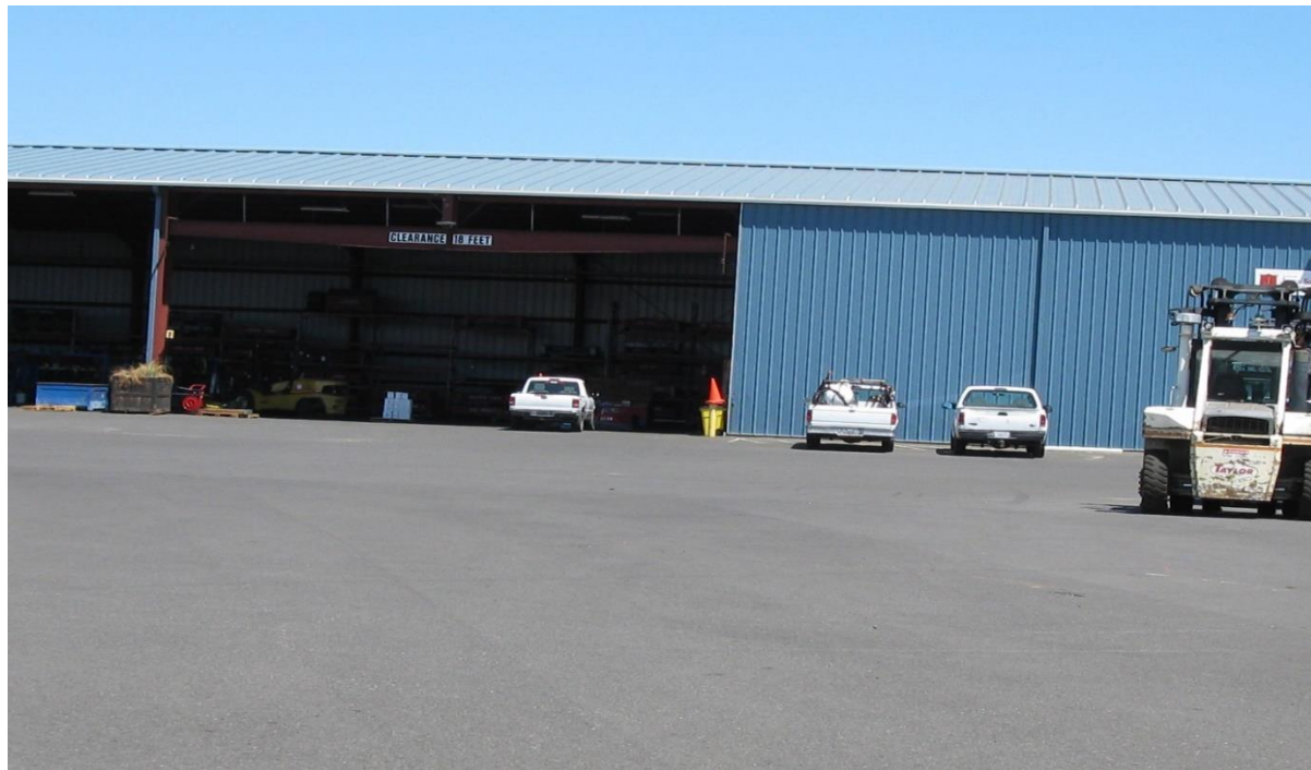
Photo 1. Former pond area and engineered asphalt cap and new building—from the Southeast.
