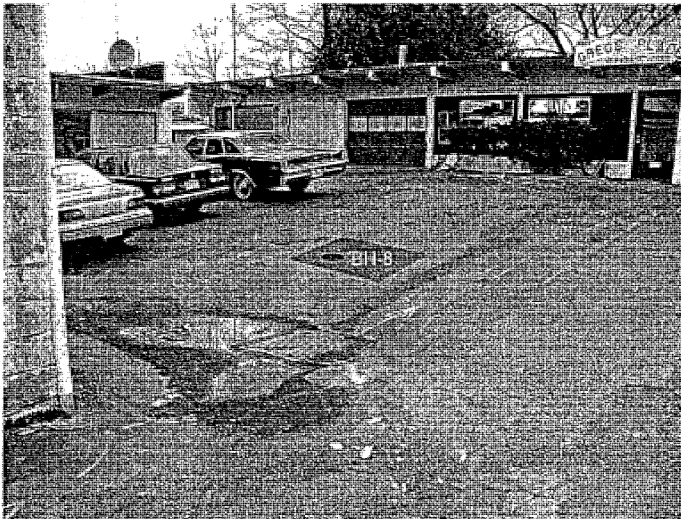
Photograph NO. 2: Gregs Place Auto Body Shop. Borehole BH-8 is in center of photograph. View looking northwest. (See various utility markings on pavement.)
