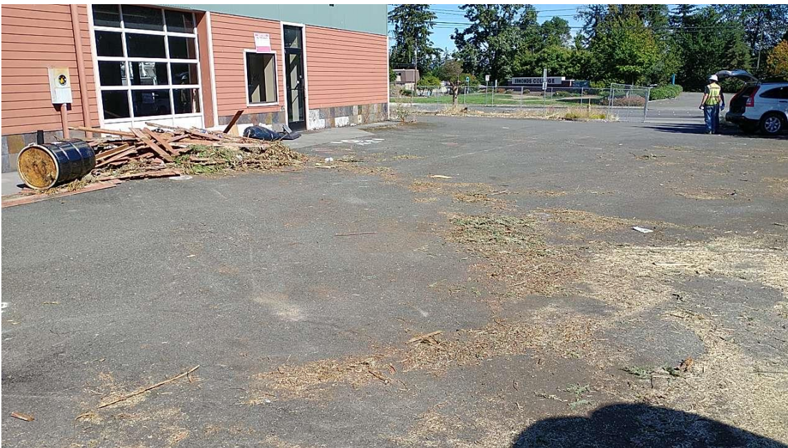
Stockpiles of boards and 55-gallon drum. Facing north.
