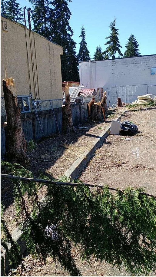
Tree removal. Facing West.
