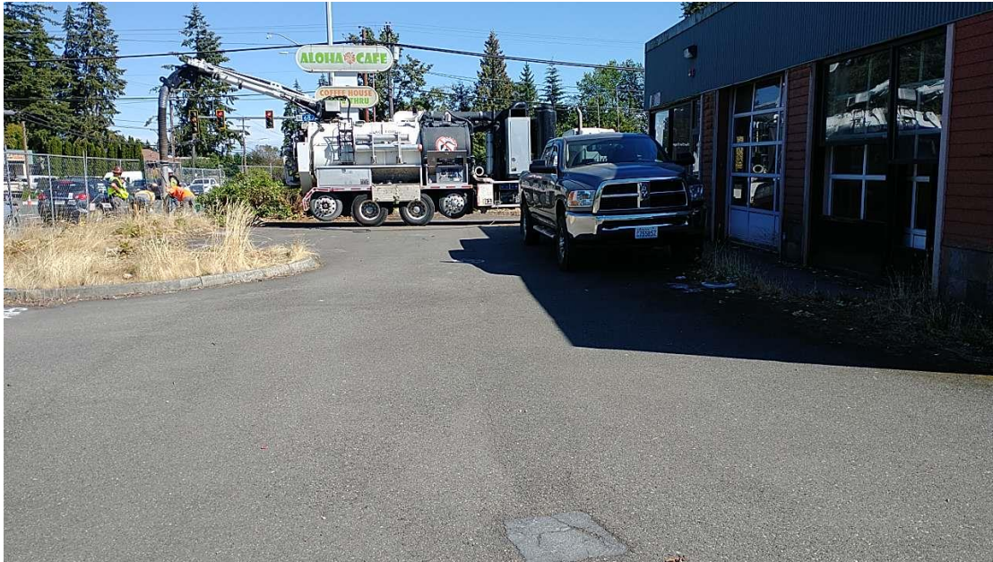
Potholing activities. Facing west.
