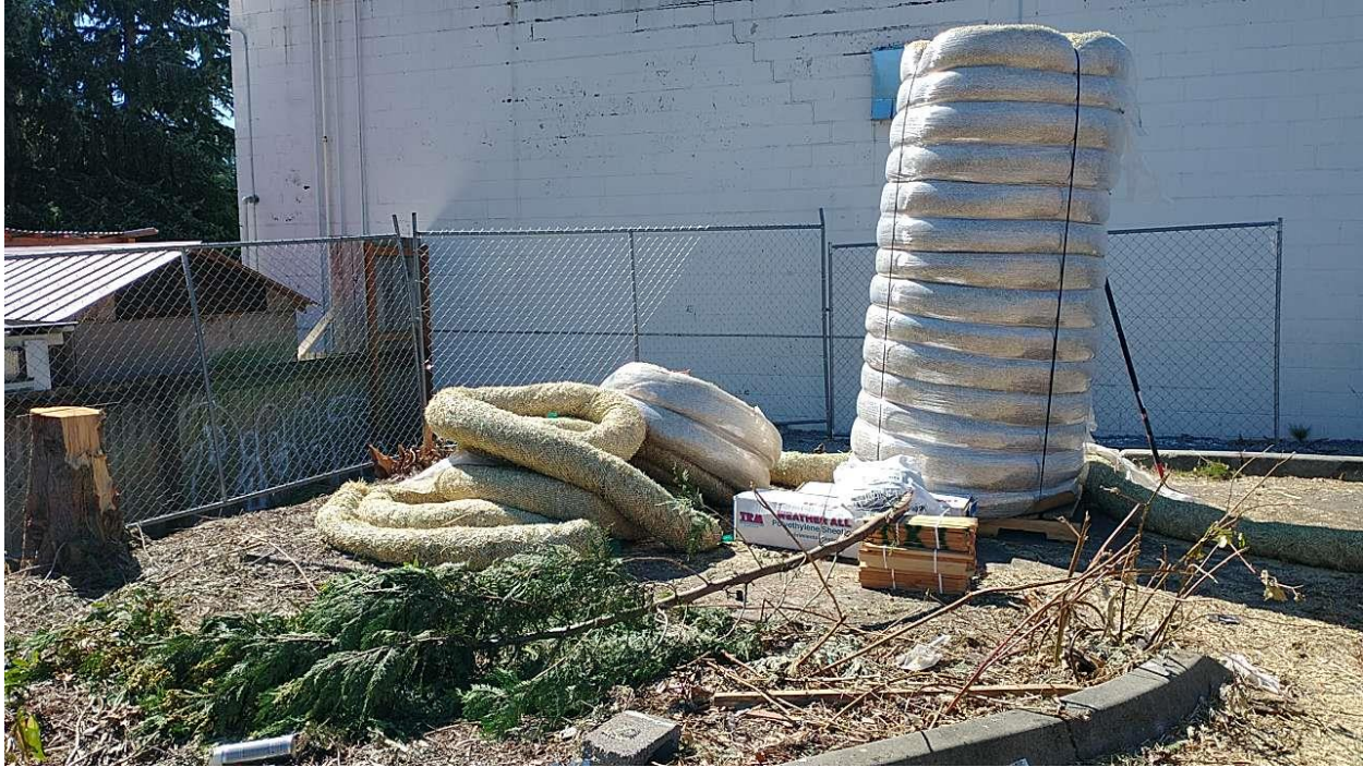
Erosion control materials in southeast corner of site.
