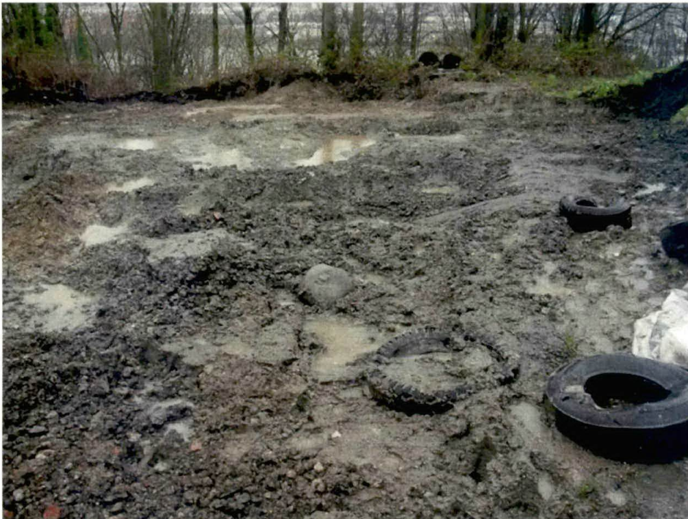
Photograph #22 - 2/3/06 – Showing removed gravel where trucks had been loading.
