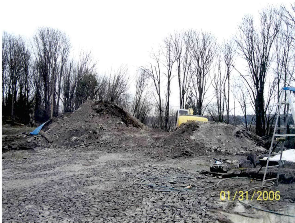
Photograph #13 – View of the west side of the pile.
