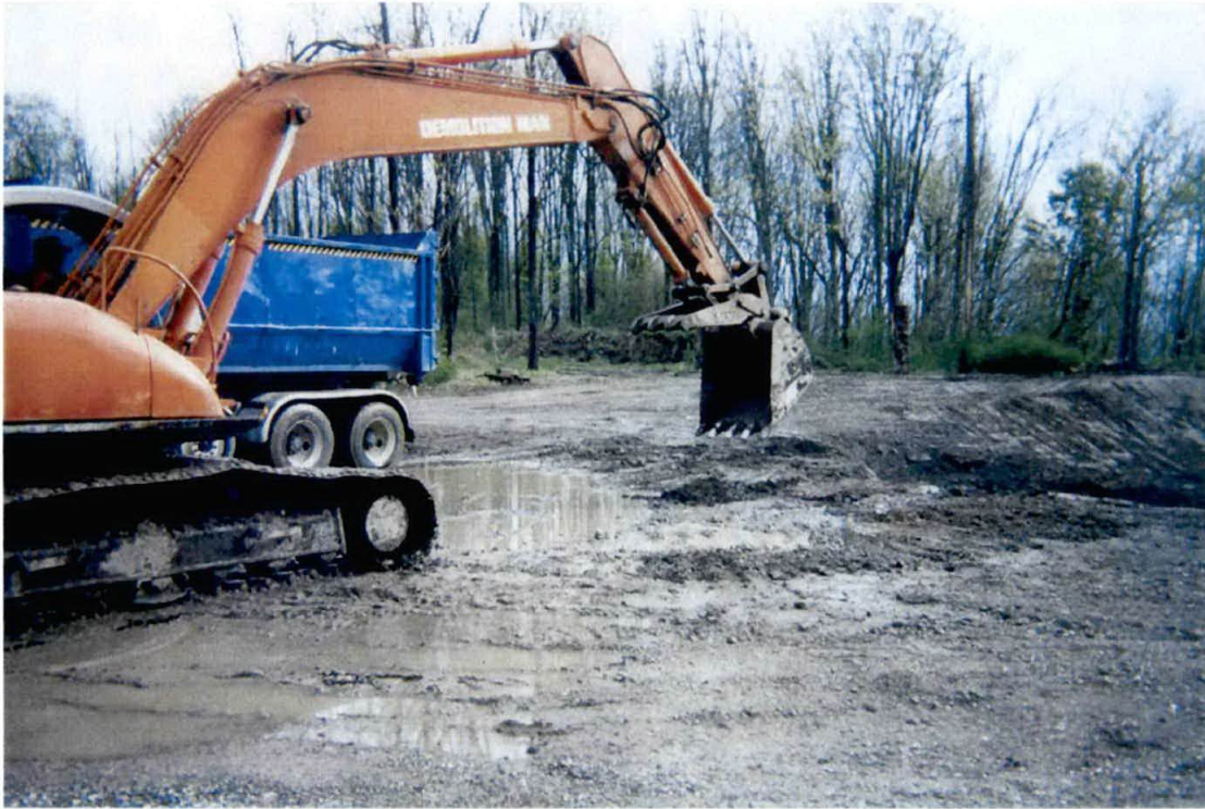
Photograph #21 – Final removal of CKD material after grading.
