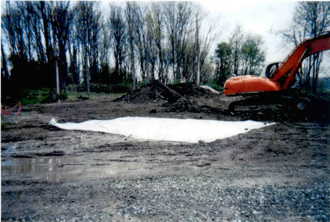
Photograph #5 – View during preparation for excavating CKD material showing plastic sheeting.
