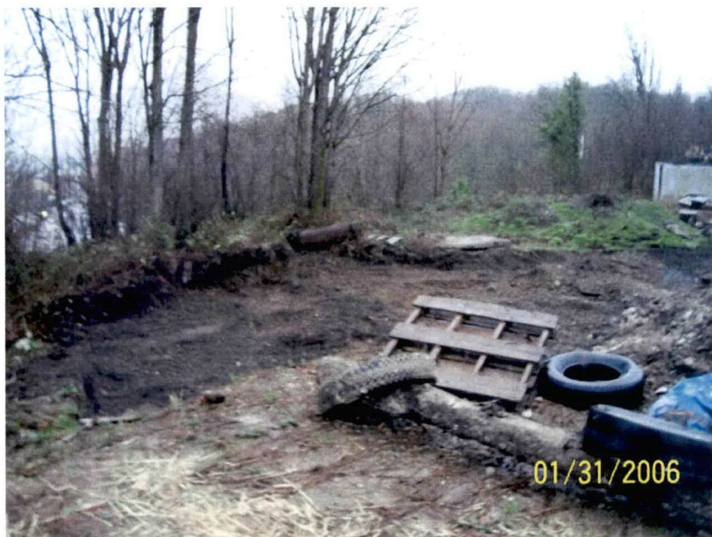
Photograph #12 – Showing completed removal of the east side of pile.
