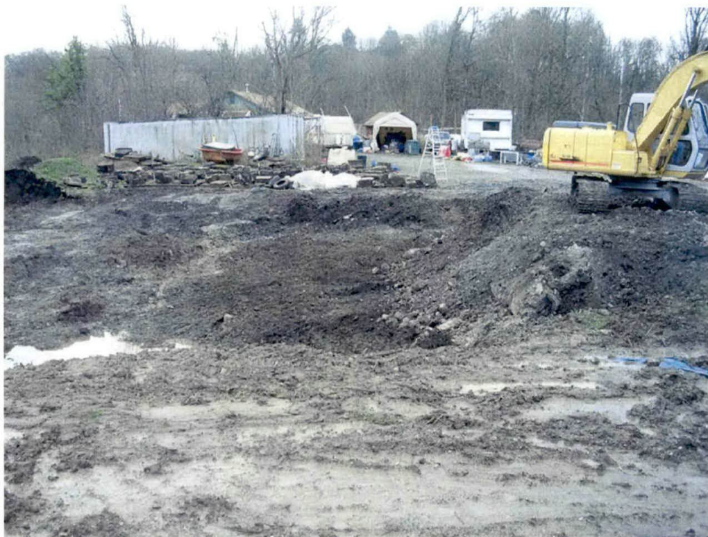
Photograph #19 - 2/2/2006 – View looking south across the pit showing reminder of pile.
