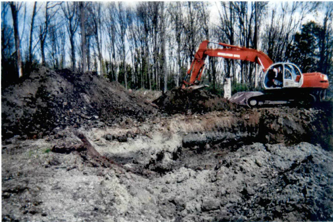
Photograph #8 – View showing stockpile of excavated battery casing material.
