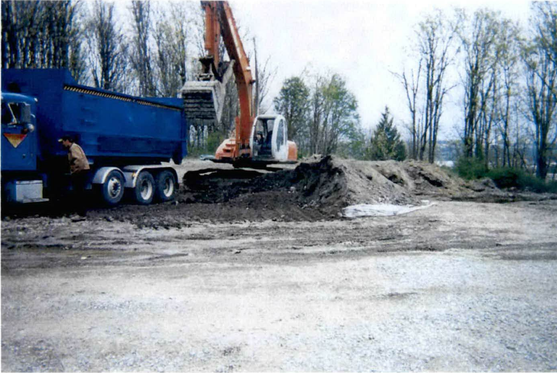
Photograph #19 – Further removal.
