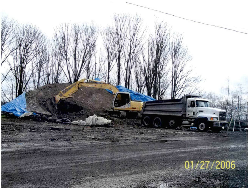
Photograph #5 – Further removal of pile.
