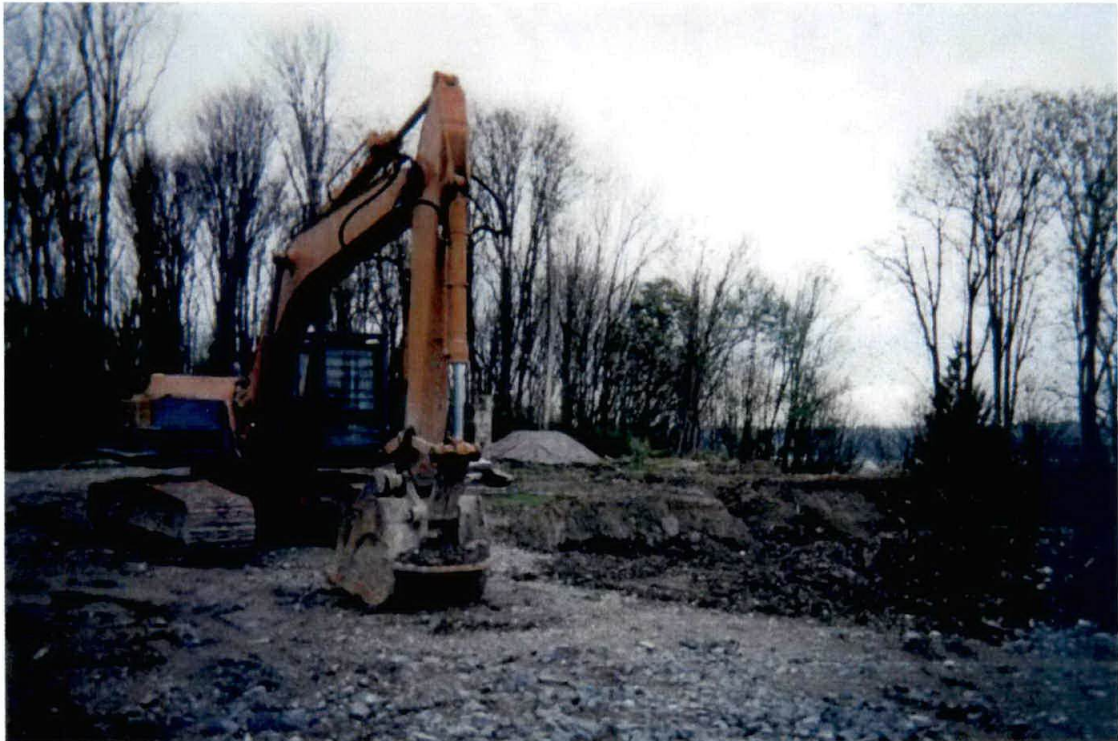
Photograph #6 – View during excavation of battery casing material showing excavator.
