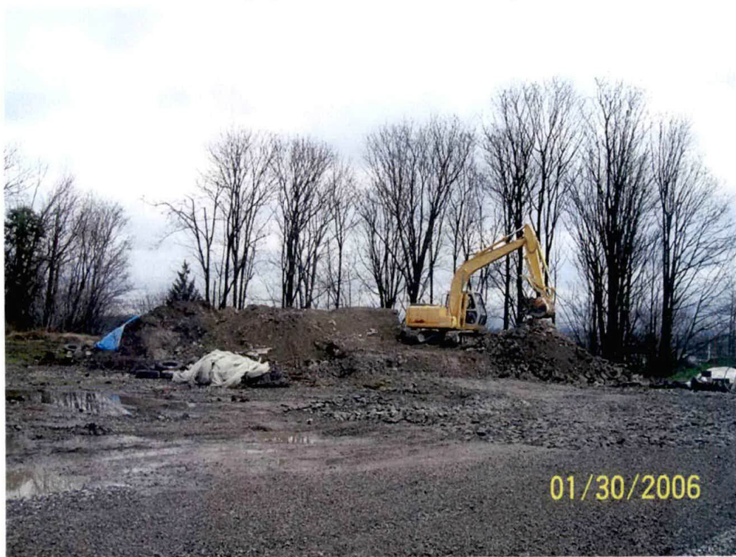
Photograph #6 – Progression of removal.
