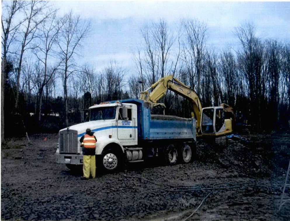
Photograph #17 - 2/2/2006 – Loading dump truck with pile material.
