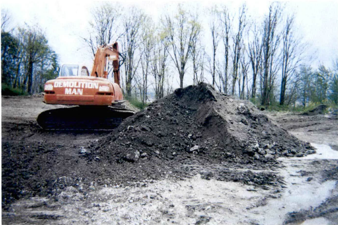
Photograph #18 – Further removal of CKD material.
