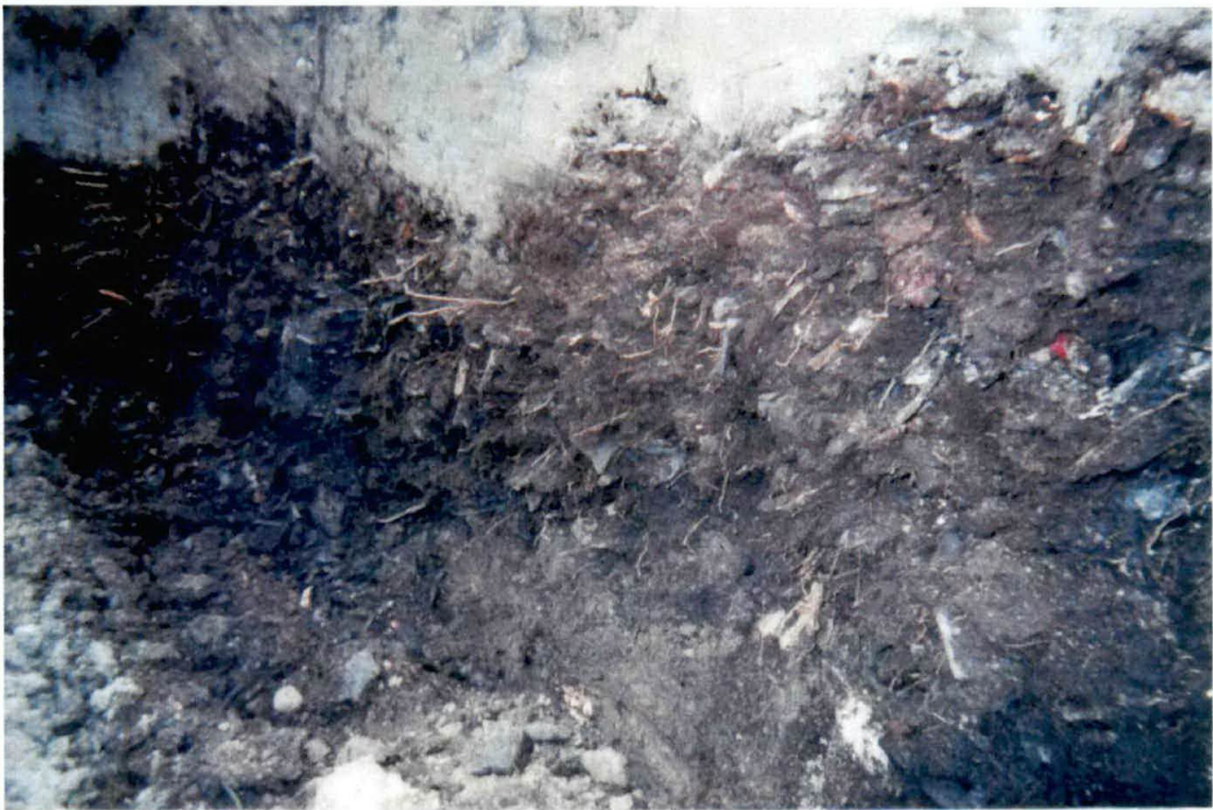
Photograph #4 – View during excavation of battery casing material and wood debris.
