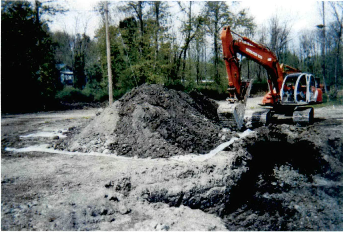
Photograph #11 – Excavation completed of the CKD material.
