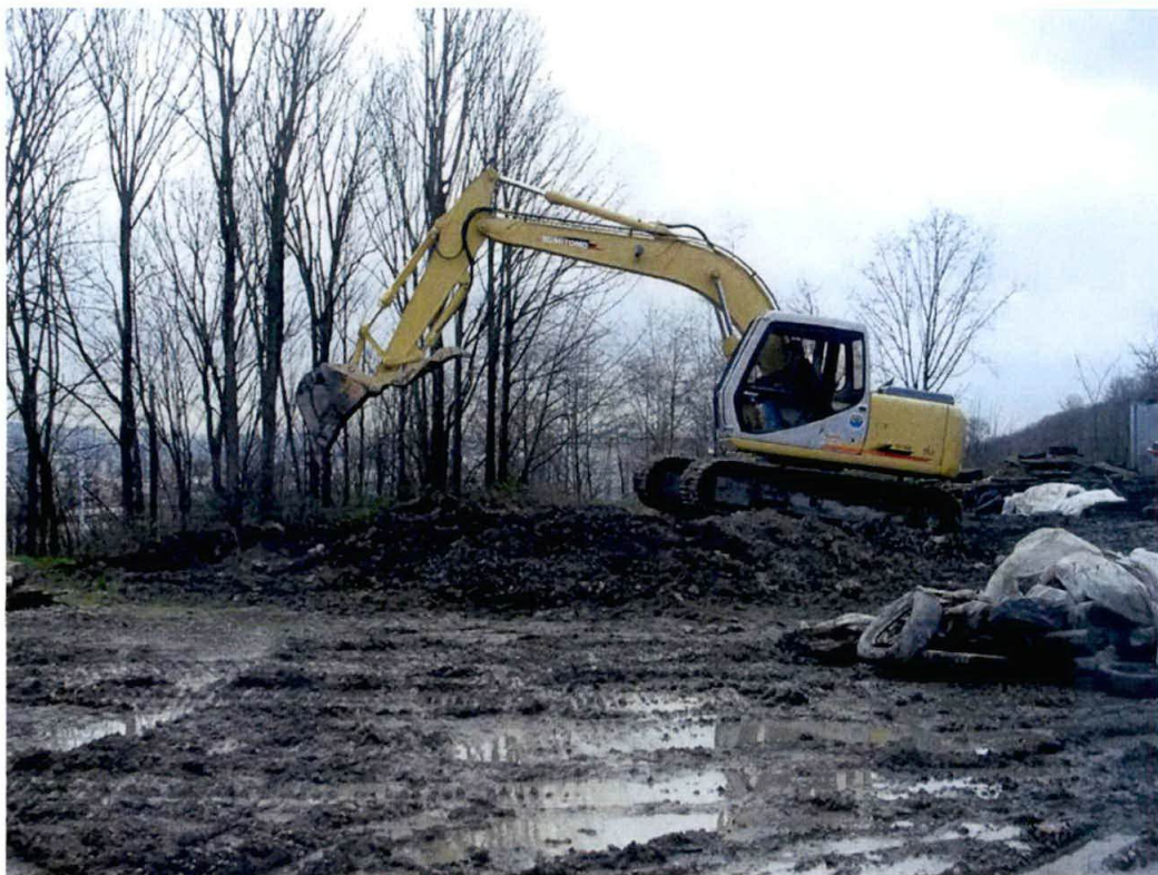
Photograph #16 - 2/2/2006 – Further removal of pile.
