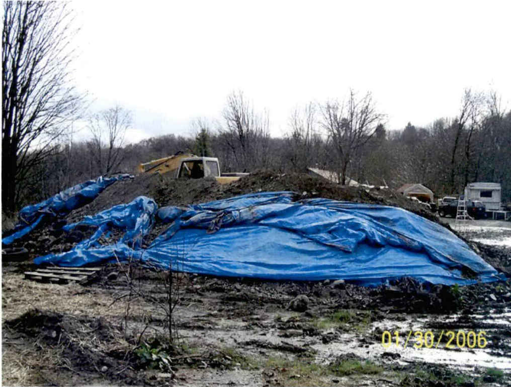
Photograph #7 – Side view of pile
