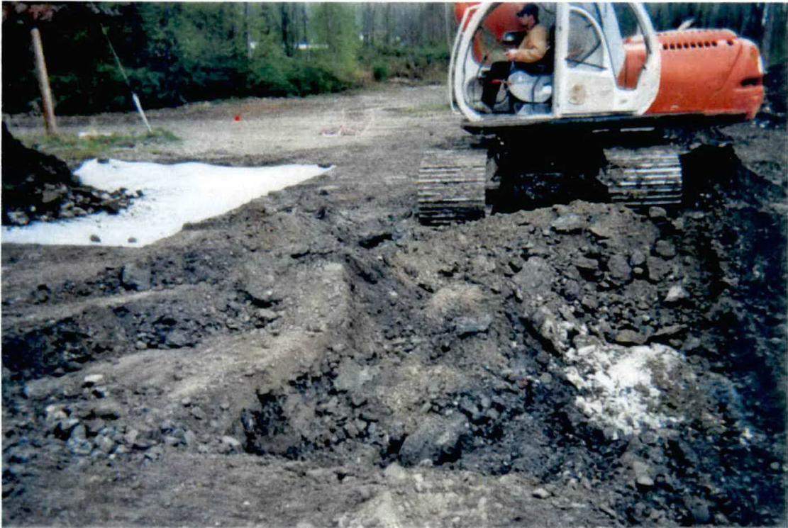
Photograph #7 – View during excavation of CKD material.
