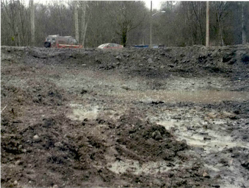
Photograph #21 - 2/3/2006 – Showing west side of excavated cavity.
