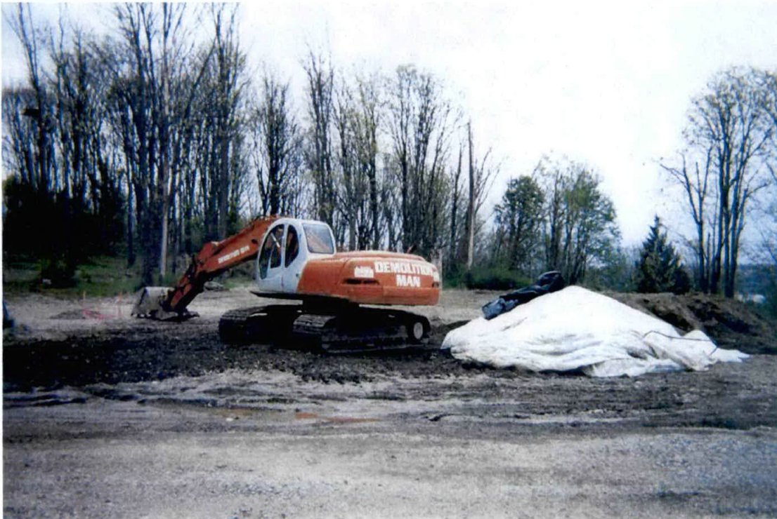
Photograph #20 – Small pile of CKD material left to be removed on Friday April 14, 2006.
