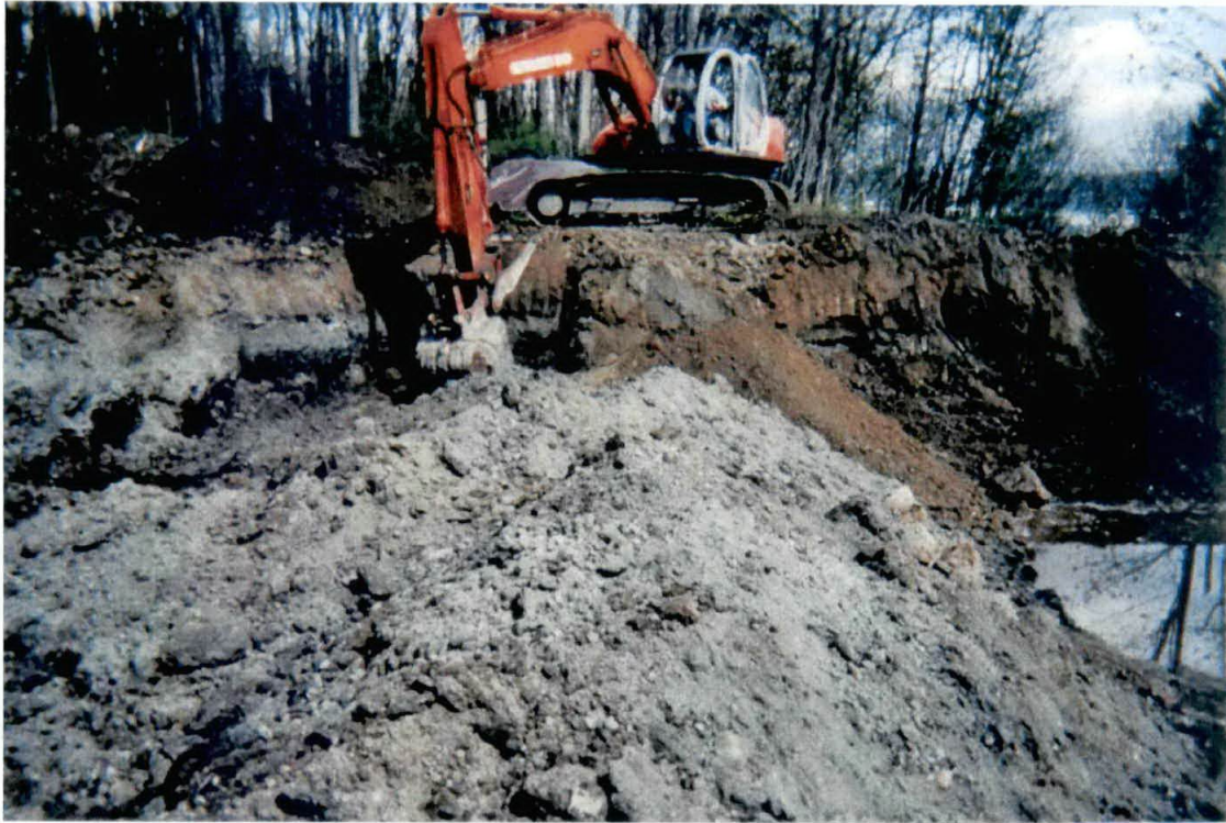
Photograph #11 – Further removal.
