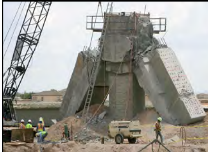
Demolition of Highway Bridge
