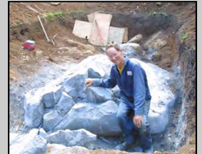
Swimming Pool Excavating
