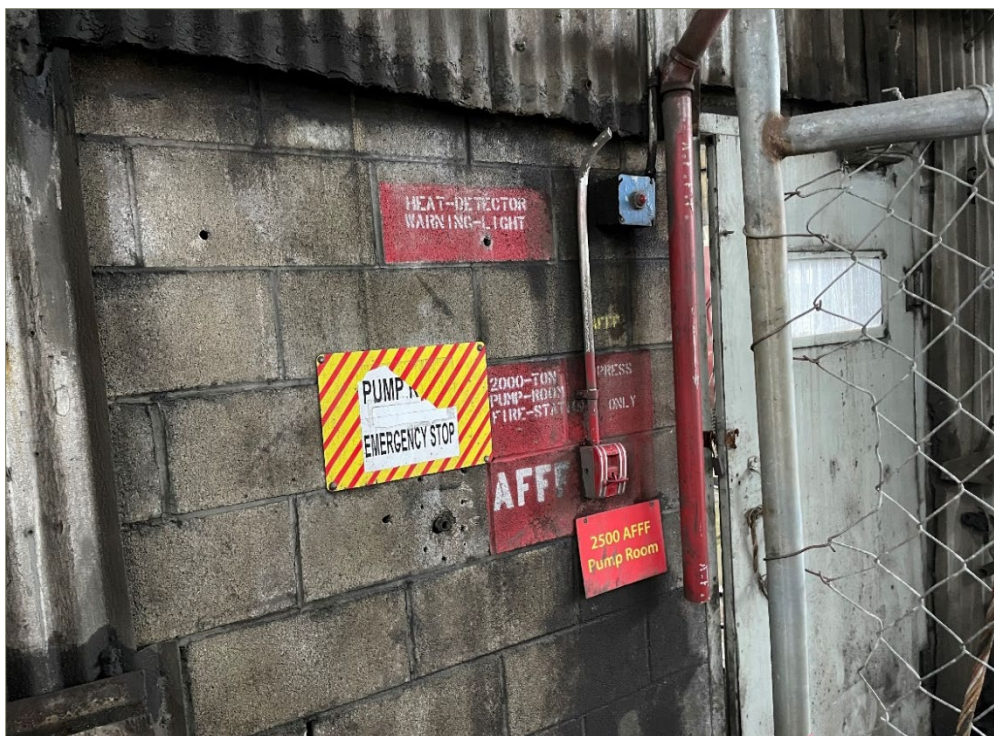
Exhibit 2-3: AFFF Wall Decals on the Exterior of the 2,500-Ton Press Pump Room (January 2022)
