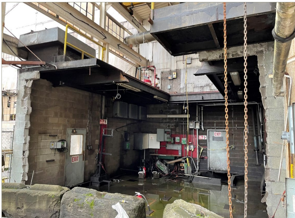
Exhibit 2-4: Interior of the 2,500-Ton Press Pump Room with AFFF Tank Visible on Roof (January 2022)
