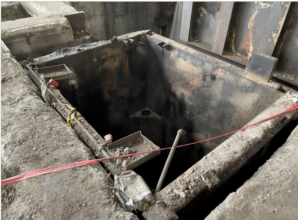
Exhibit 2-7: Sprinklers on Westernmost Quench Tank (January 2022)
