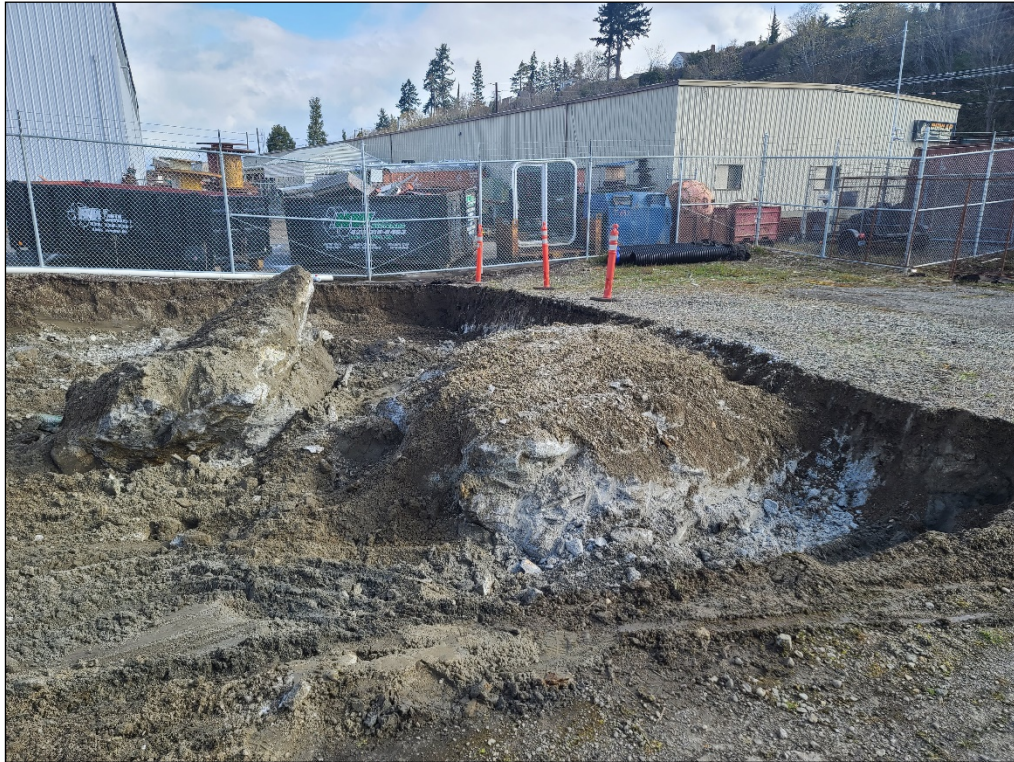
1. Looking northeast at area H with concrete material uncovered during excavation.
