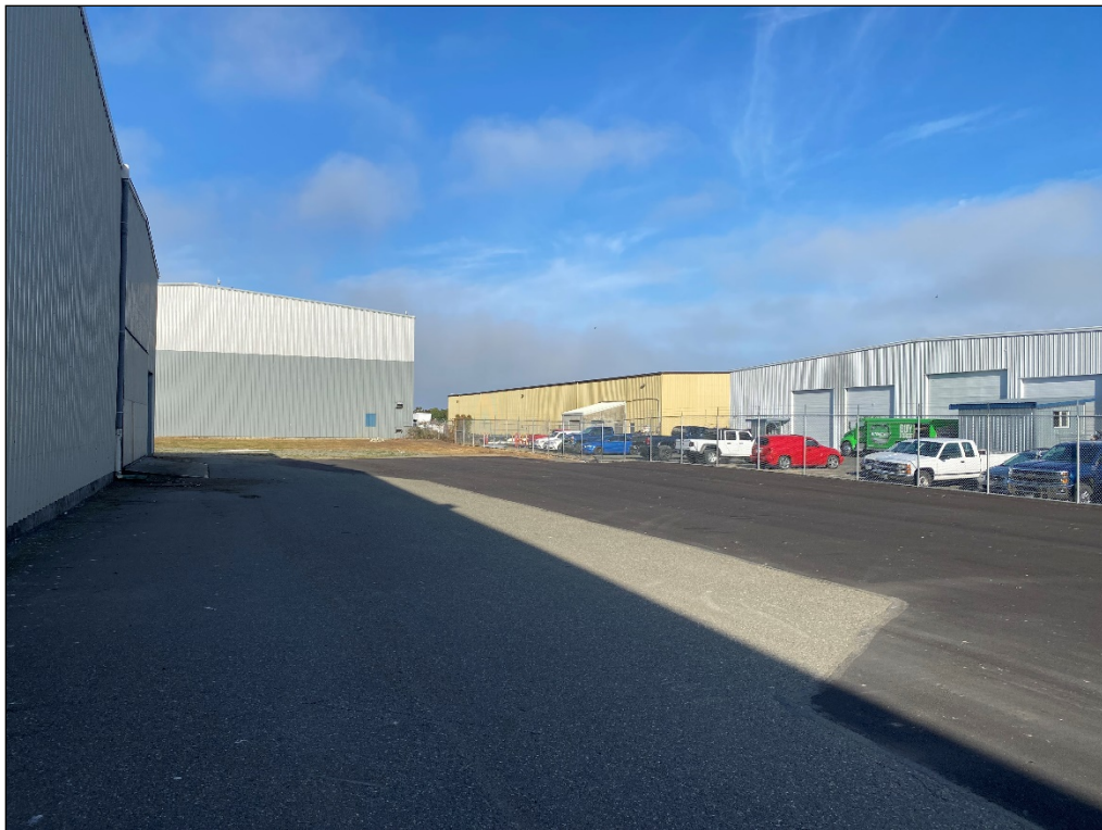
4. Looking west at paved and filled G-2 area.
