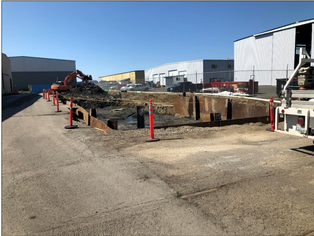
3. Looking west from area H with shoring installed during excavation.
