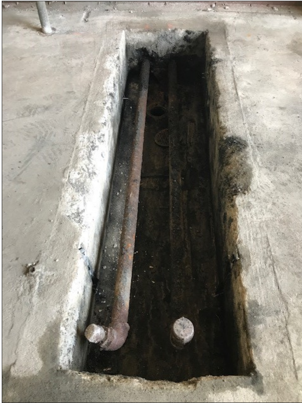
5. Cleanup Area G-4 vault after removal of sandblast grit.
