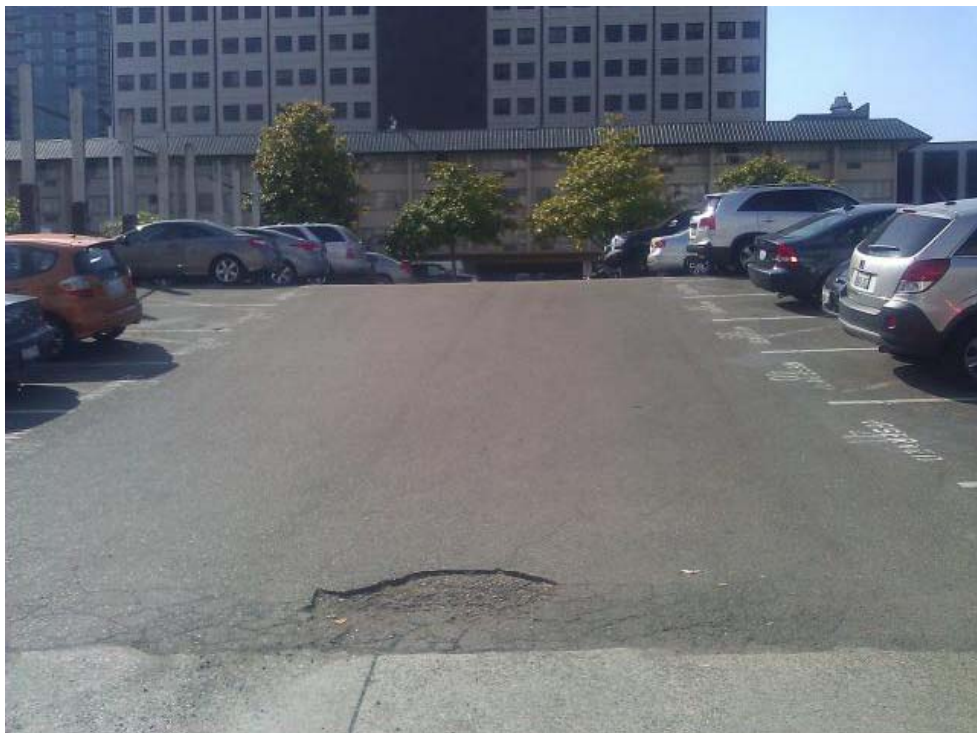
LOOKING WEST ACROSS SUBJECT PROPERTY FROM ALLEY
